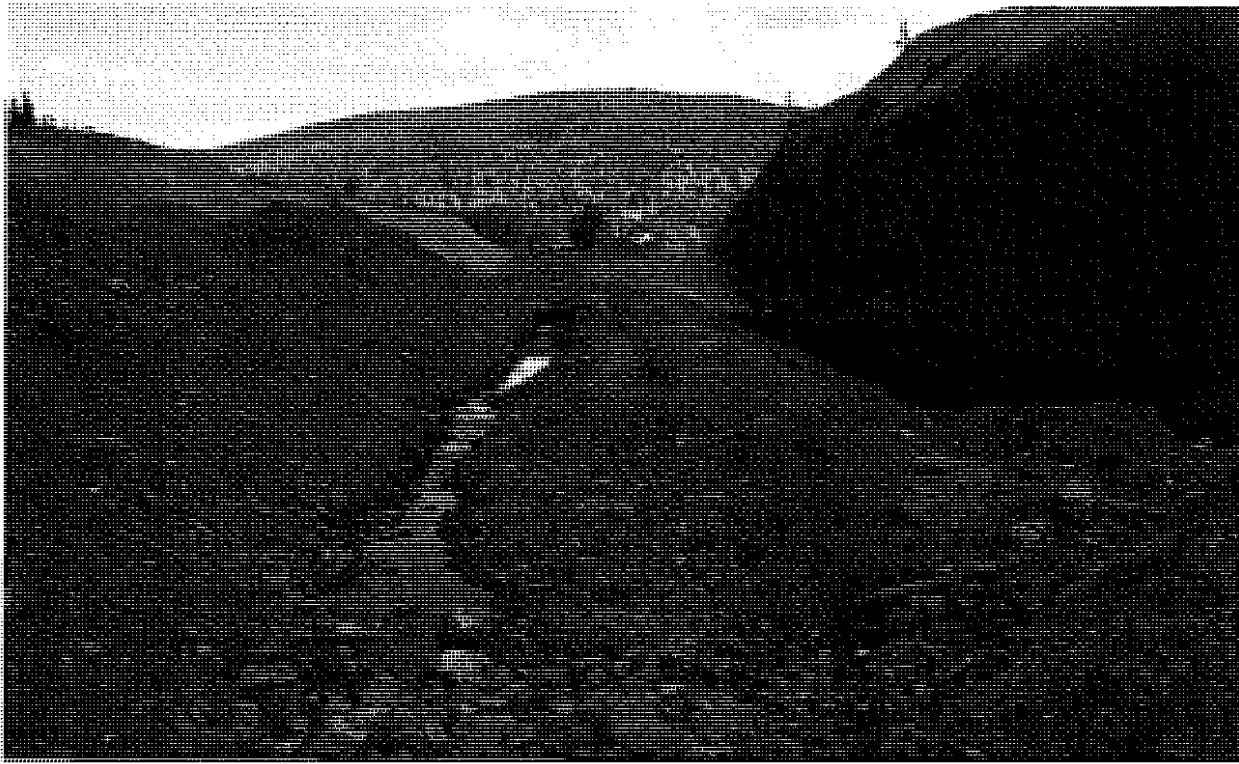
Figure 2. Excavated and diverted stream channel through placer mine site
