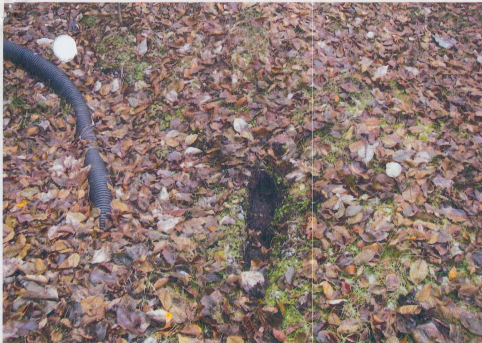
Small outflow below collection box
