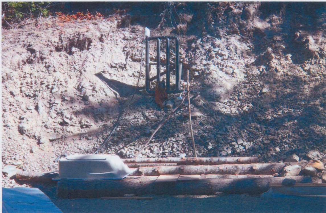
construction site/pipes - Jini + Noda's
