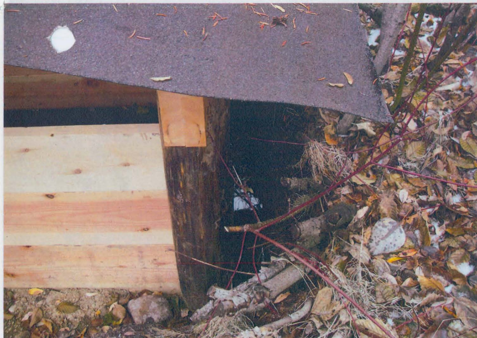
Inlet end of collection box dug into gully.
