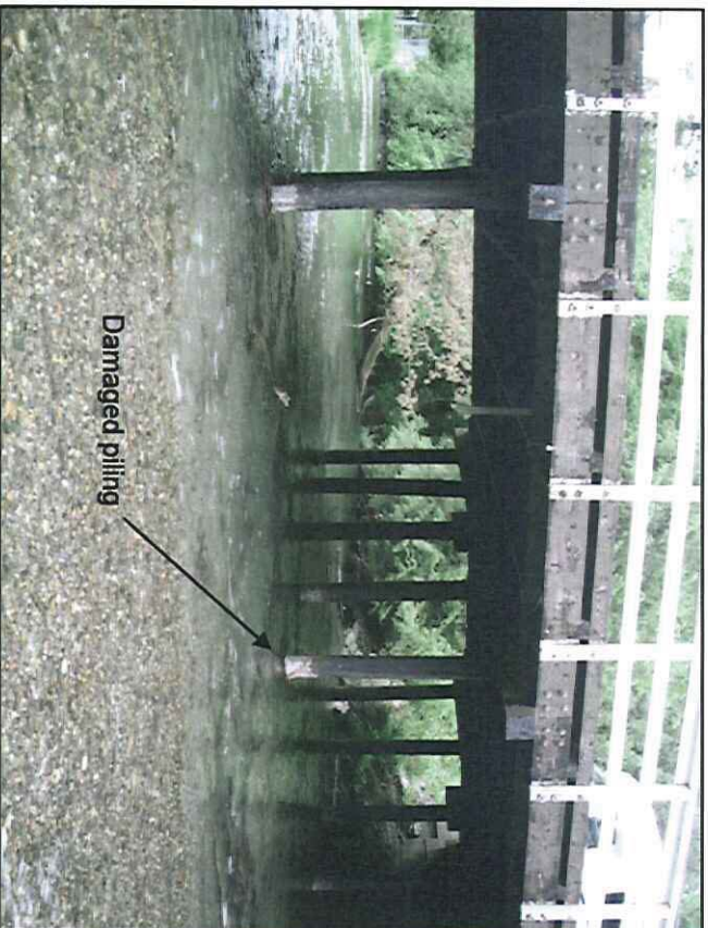
Photograph 3: View of piling repair location looking downstream. Recommended instream access would be from the right hand (southern) side of the photograph.
