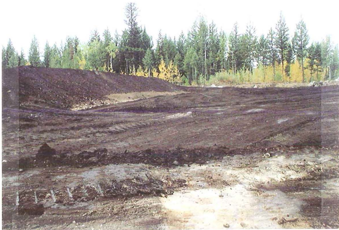
LEONARDITE STOCKPILE BEING USED FOR RECLAMATION AS TOP SOIL DRESSING - RED LAKE PIT.
