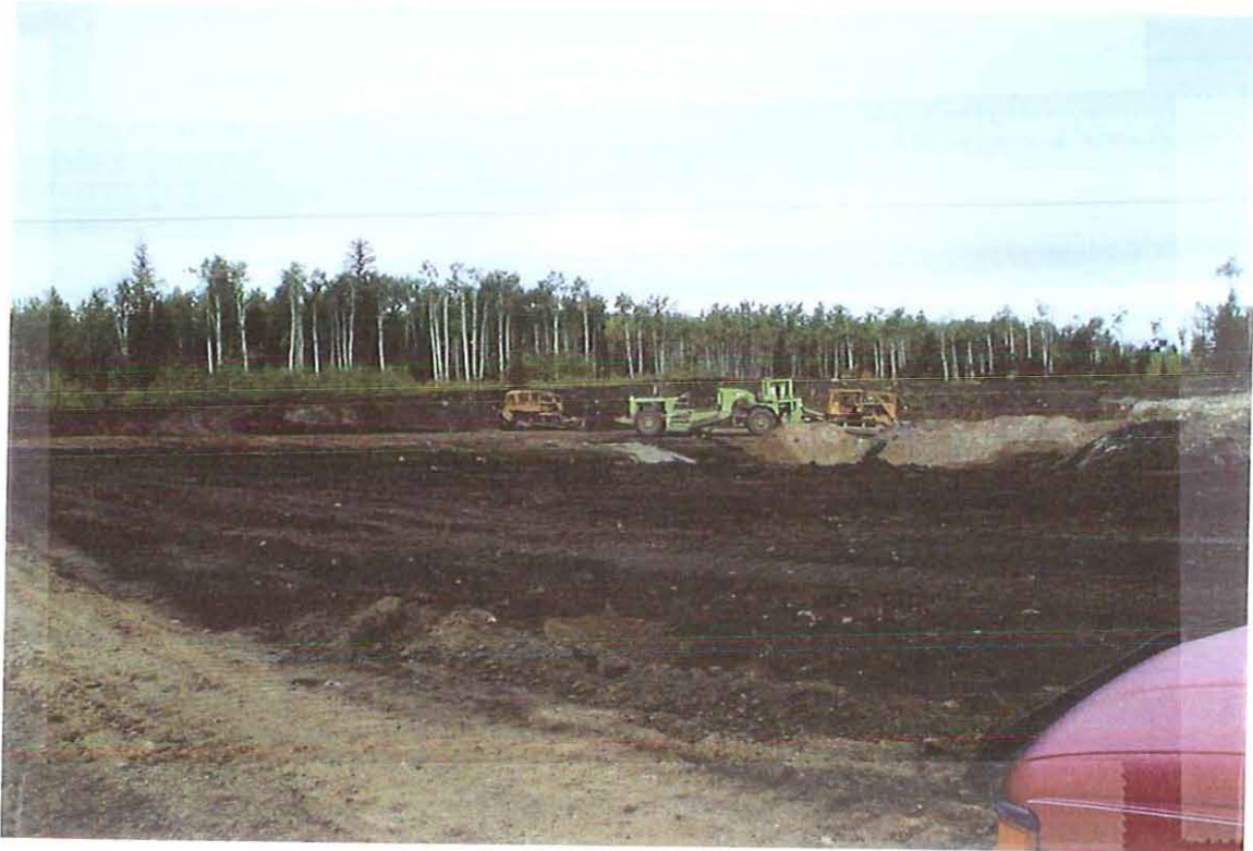
WEST PIT - BACKFILLING - PLACEMENT OF SOIL & LEONARDITE COVERING.
