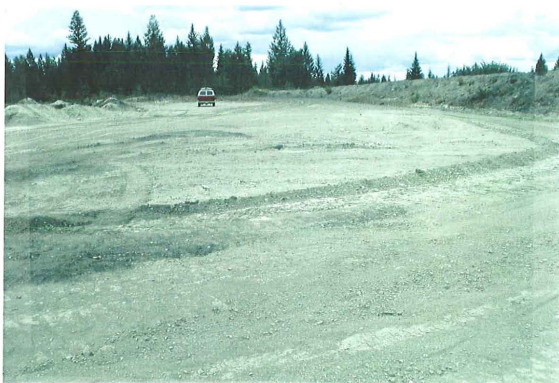
Red Lake Pit - backfilled and graded area ready for topsoil and seed
