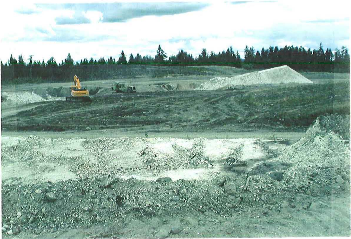
West Pit - levelling, topsoil placement from stockpile.
