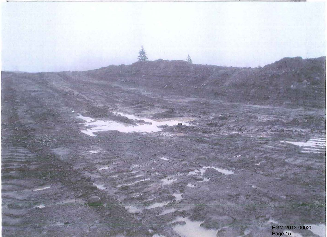
BACKFILL OF OVERBURDEN WASTE WITH SOIL COVERING - RED LAKE PIT
