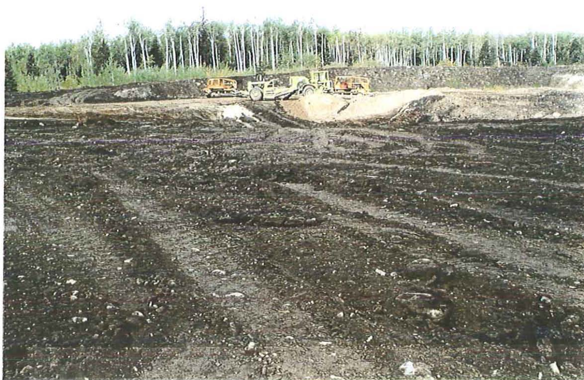
BACKFILLING OVERBURDEN | SOIL COVER - WEST PIT
