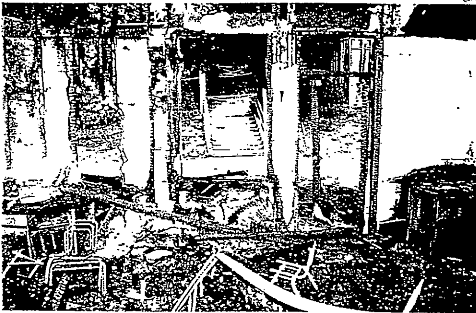
Figure 37 - Area of Origin - Multi-Purpose Room 2010 - Exterior door/window - fire and heat pattern indicators **
