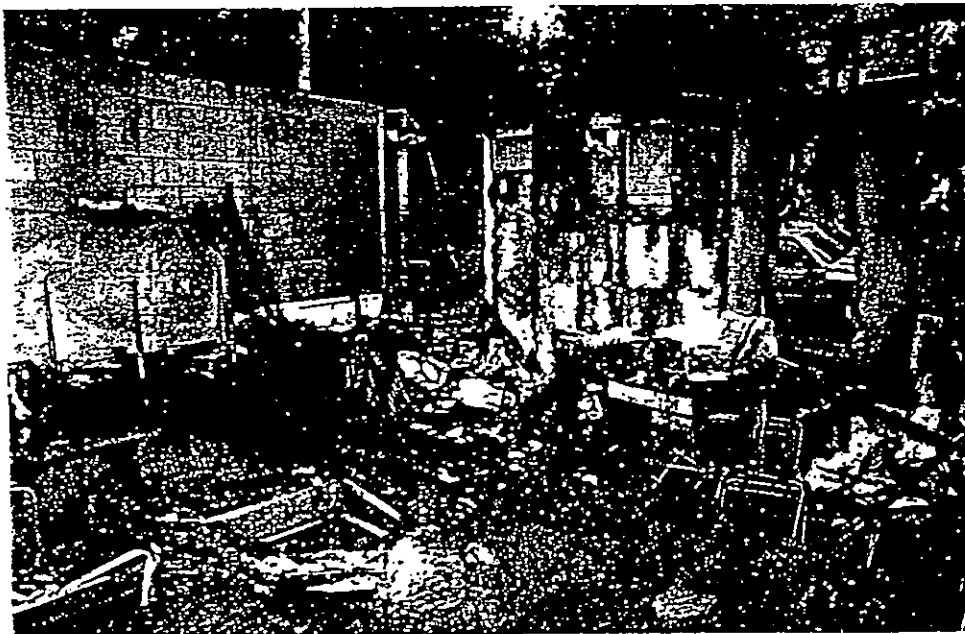
Figure 40 - Area of Origin - Multi-Purpose Room 2010 along exterior wall showing fire and heat pattern indicators **
