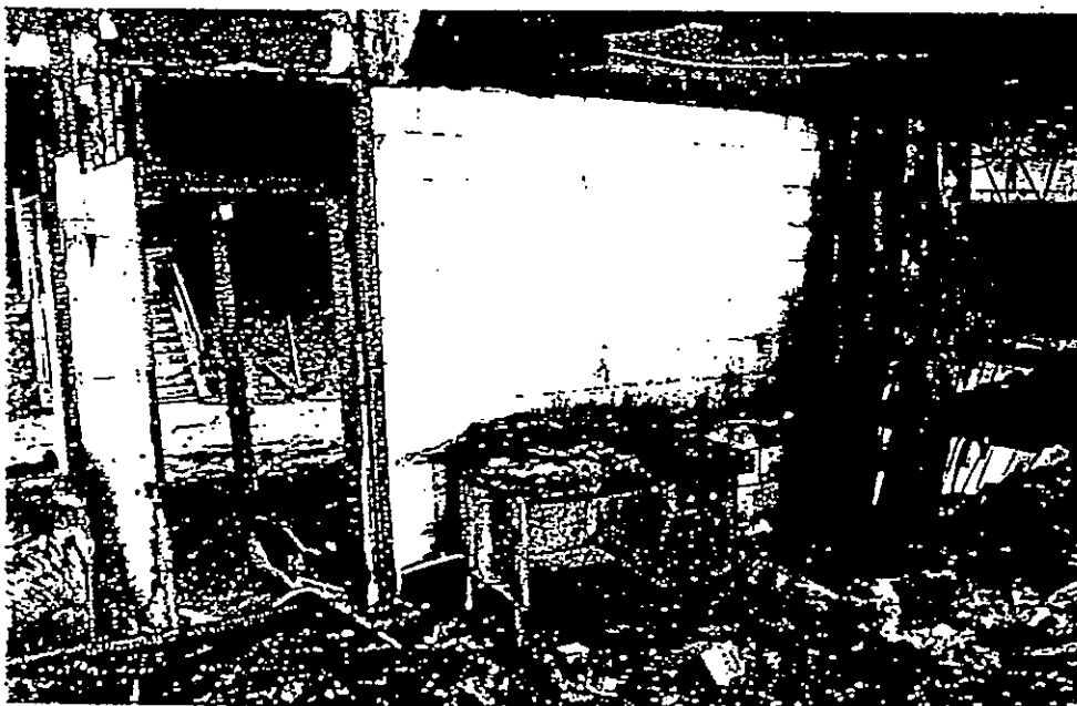
Figure 38 - Area of Origin - Multi-Purpose Room 2010 - exterior door/teachers desk - fire and heat pattern indicators **
