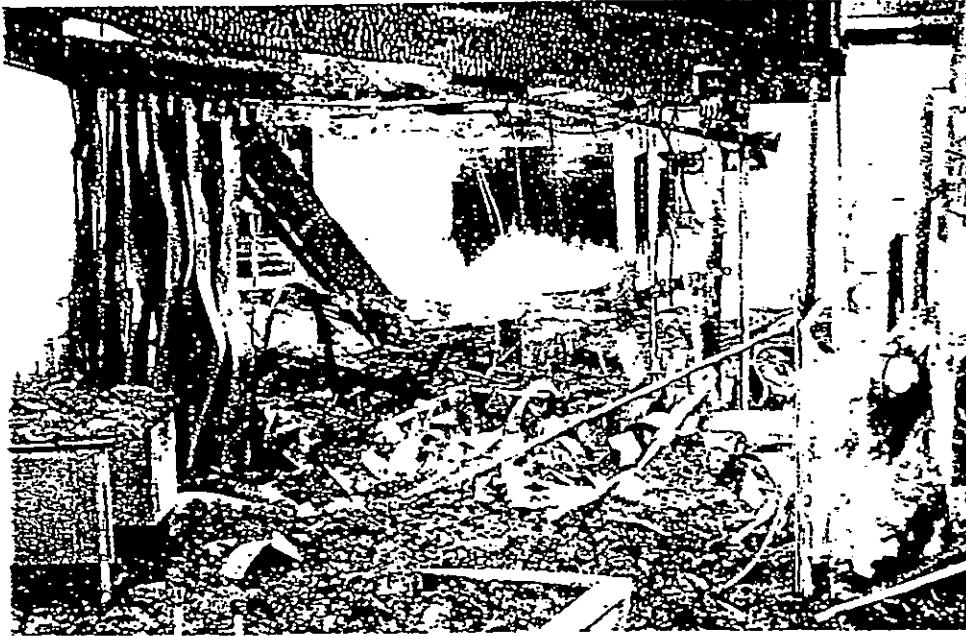
Figure 39 - Area of Origin - Multi-Purpose Room 2010 - Accordion partition wall showing fire and heat pattern indicators **
