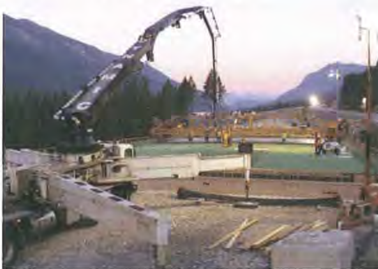
Placing deck concrete for the new four-lane Mount Hunter Creek Bridge on Phase 3 of the Kicking Horse Canyon Project, 20 km east of Golden.
