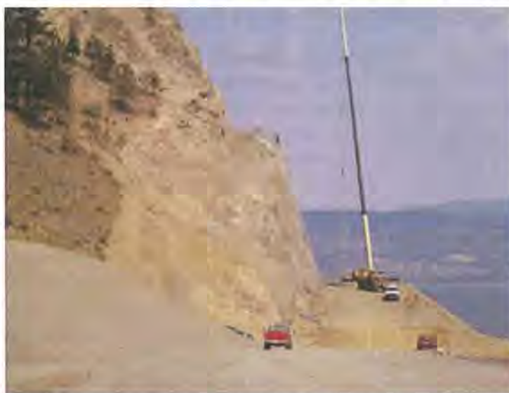
Workers install mesh to keep rock off the travelled roadway as part of the Highway 97, Bentley Road to Okanagan Lake Park Project.
