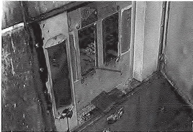
Photograph 3: Example of wood dust accumulation in MCC #9
