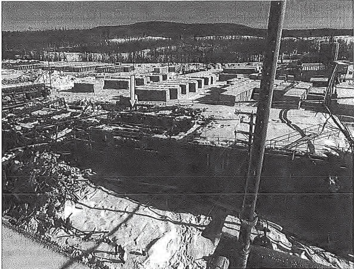
Figure 16: View of the sorter wing of the sawmill, looking east. The yellow arrow indicates approximately where the natural gas line broke. The fire damage near this location is evident.
