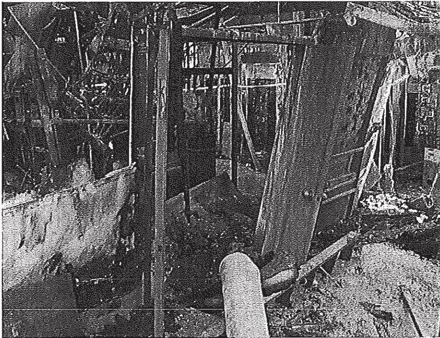
Figure 39: The line 3 hydraulic room looking south, the double doors pushed open westward. Some of the PDC electrical components are on the wall in the background.
