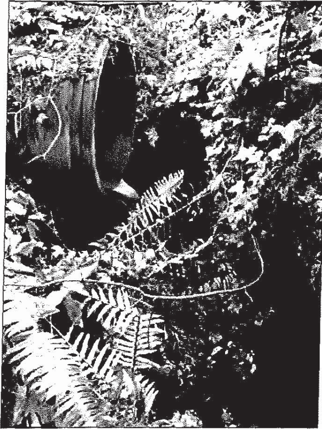
Figure 10. This culvert coming from Cedar Hill Road discharges water into a large, energy dissipating pool. This pool acts as an energy absorbing structure thereby reducing the erosional effect downstream of the water being ejected out of the mouth of the culvert. This point of discharge receives high volume, flashy, stormwater runoff from the headwater residential development in Oak Bay.
