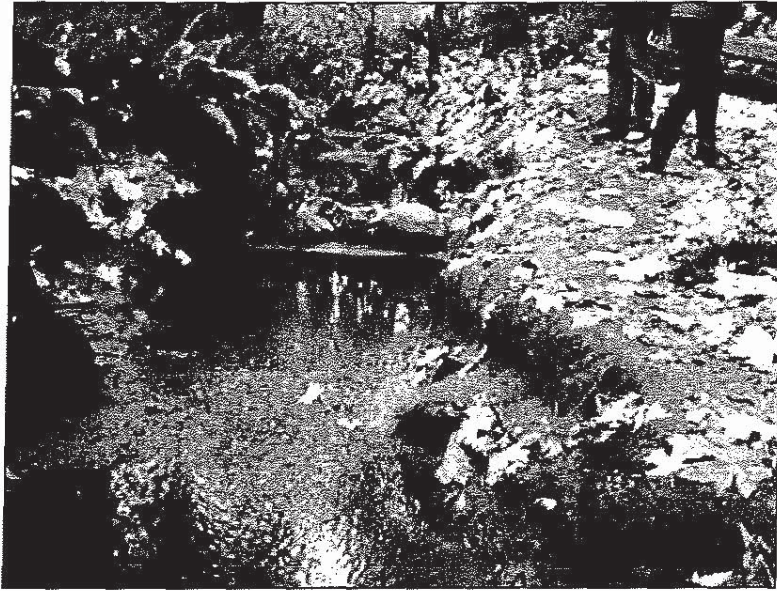
Figure 7. An example of a weir structure previously installed to minimize downstream sediment loading and to increase channel complexity. A review of existing structures for function, efficacy, and stability will enable the team to determine what needs to be replaced. Note the bare bank on the right of the photo caused by excessive trampling.
