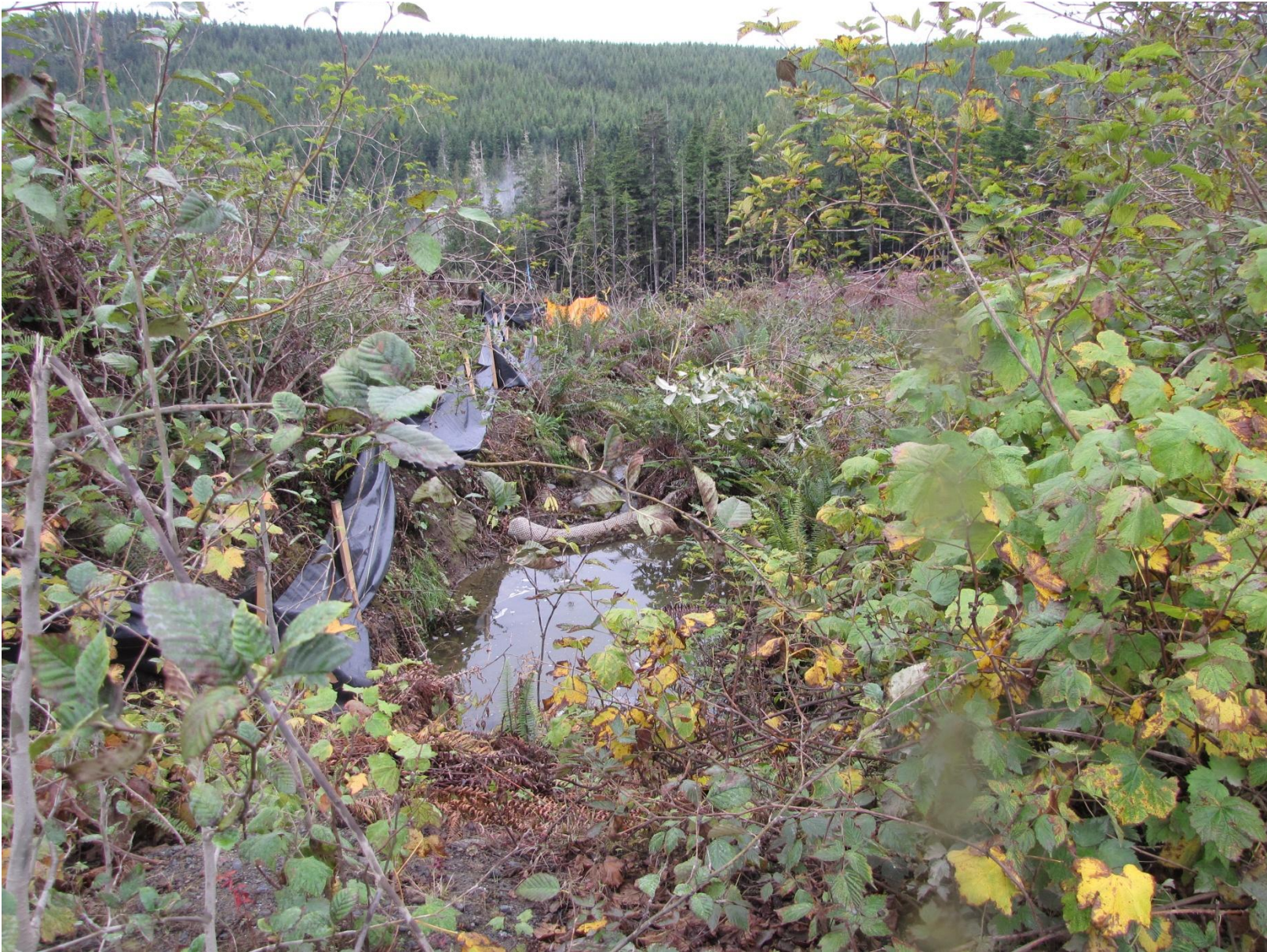
Photo 10 - French drain outflow
