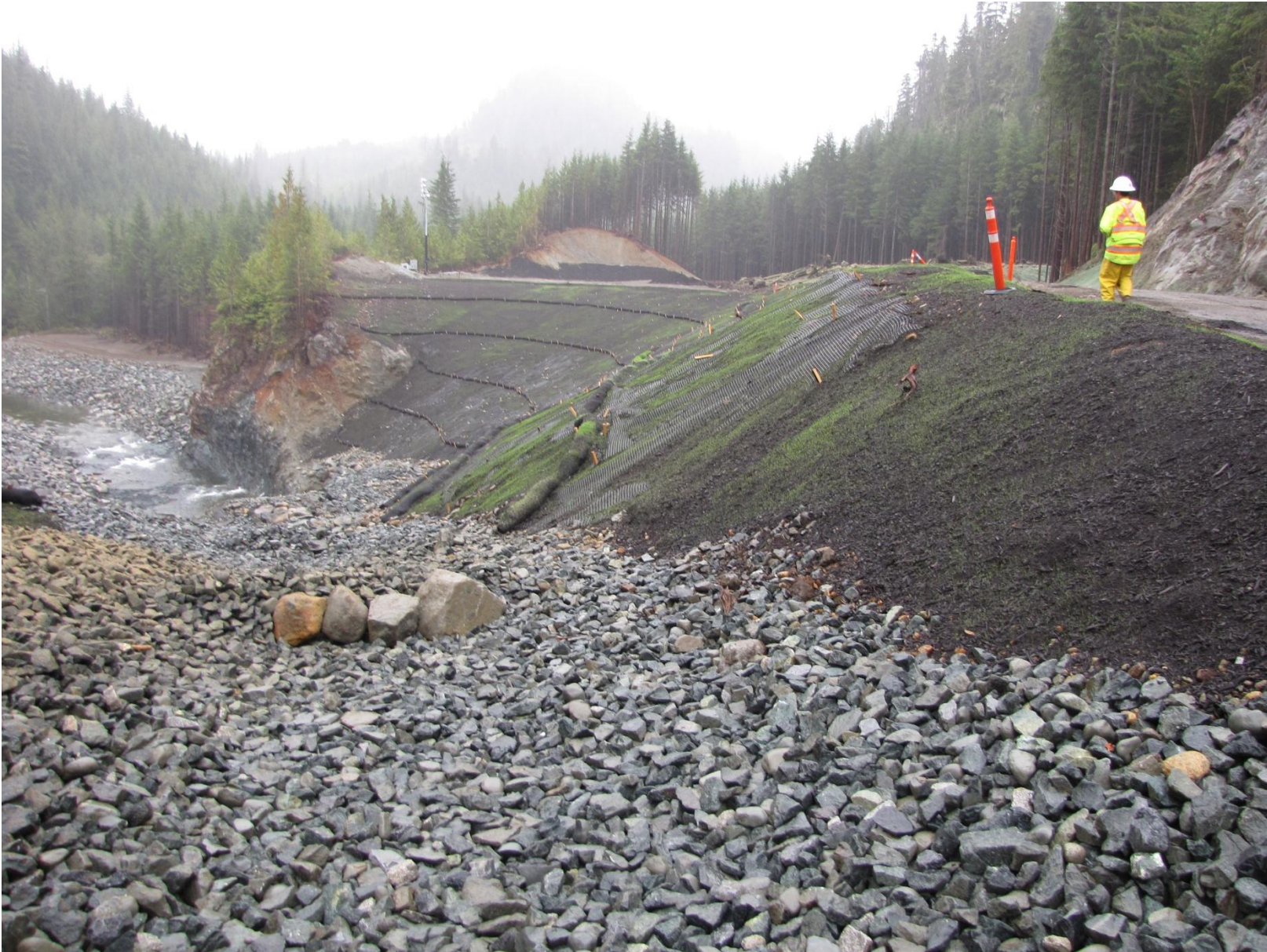
Photo 5 - slope above temporary diversion channel September 28. Hydroseeding germination
