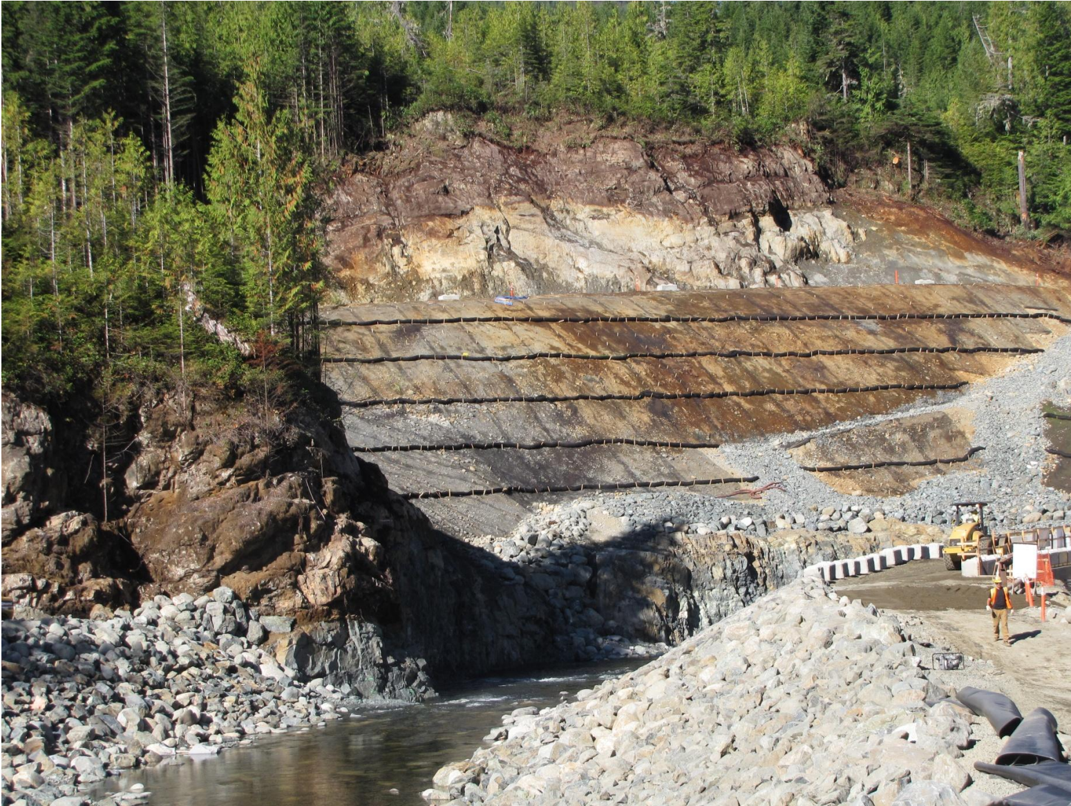
Photo 1 - Exposed soil above temporary diversion channel
