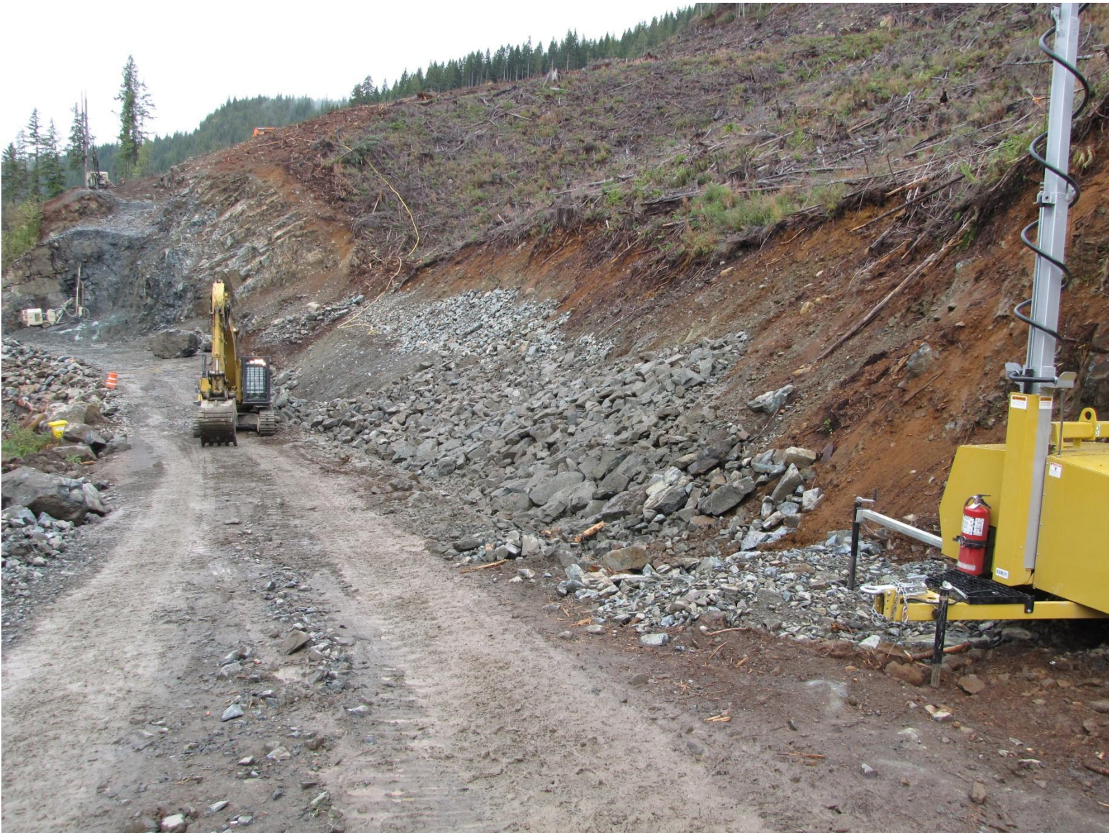
Photo 7 - Rock armouring of ditchline to minimize sedimentation
