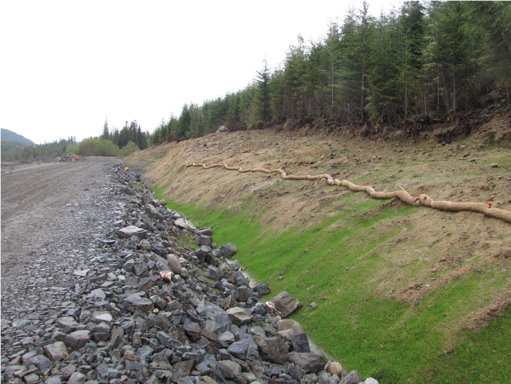
Photo 9 - hydroseeding of exposed slope and rock armouring of ditchline
