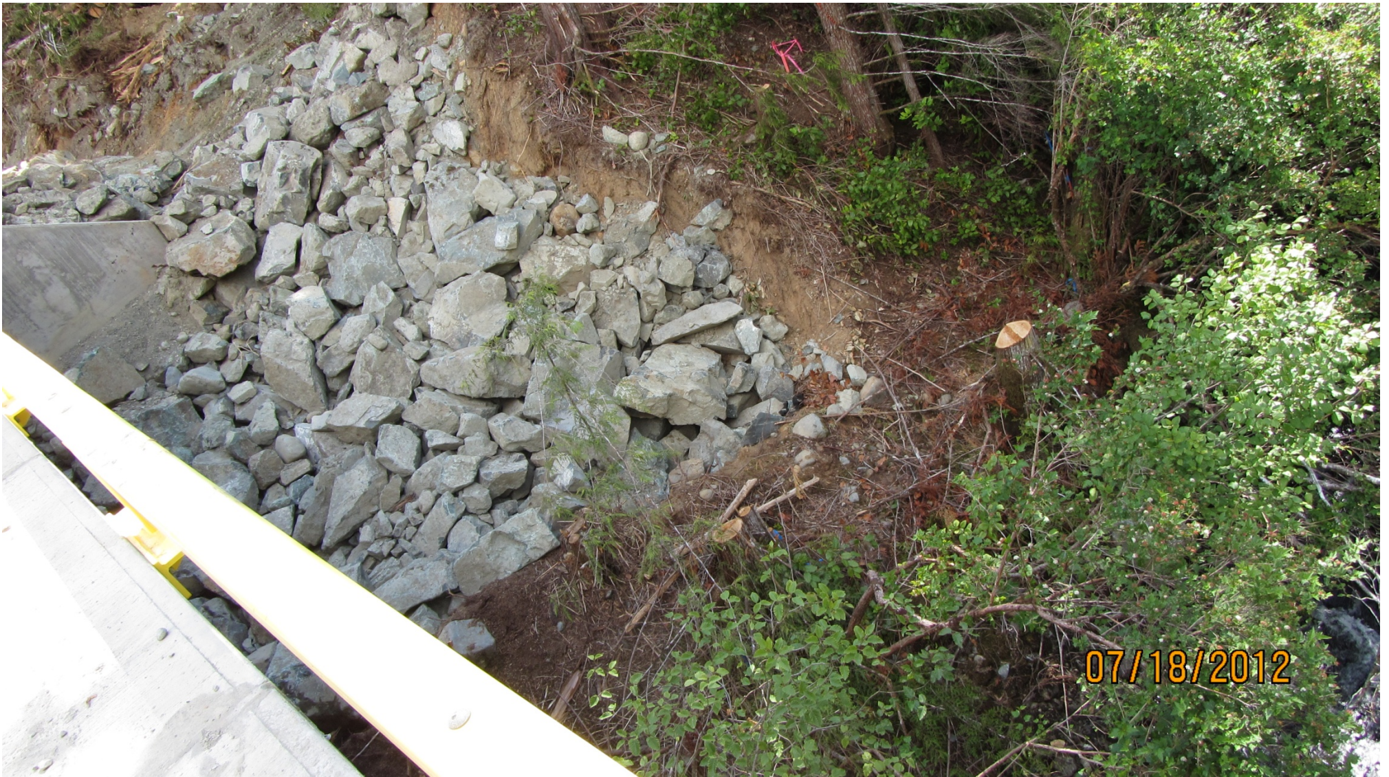
Attachment 2 - Erosion and Sediment control on Clear Span Bridge
