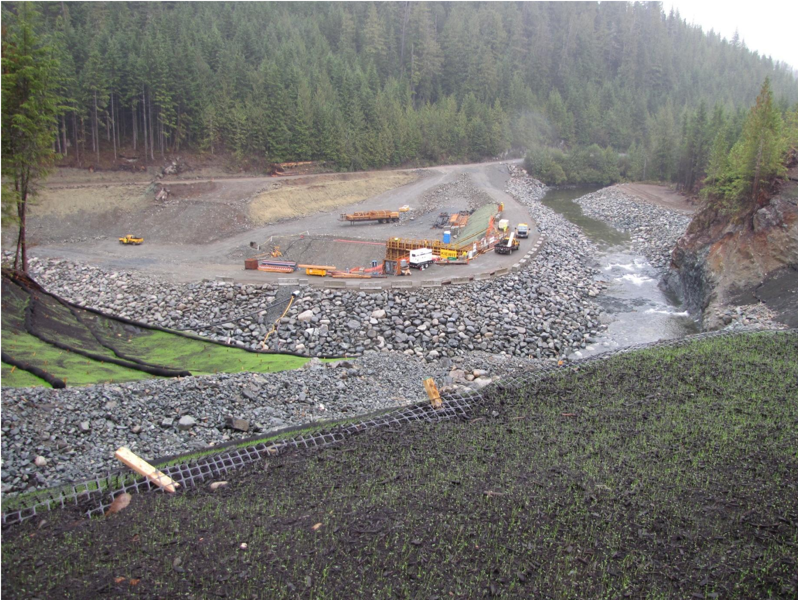
Photo 12 - Temporary diversion channel
