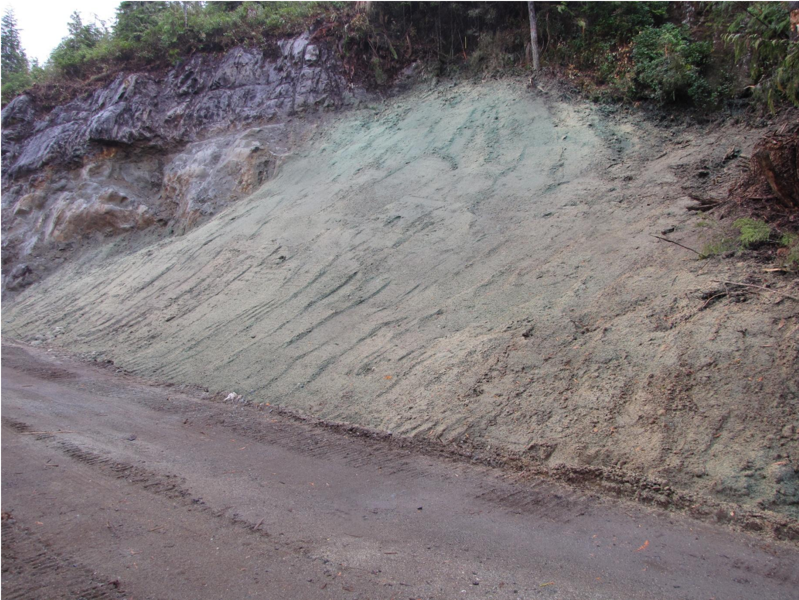
Photo 6 - Hydroseeding along Kokish Main road
