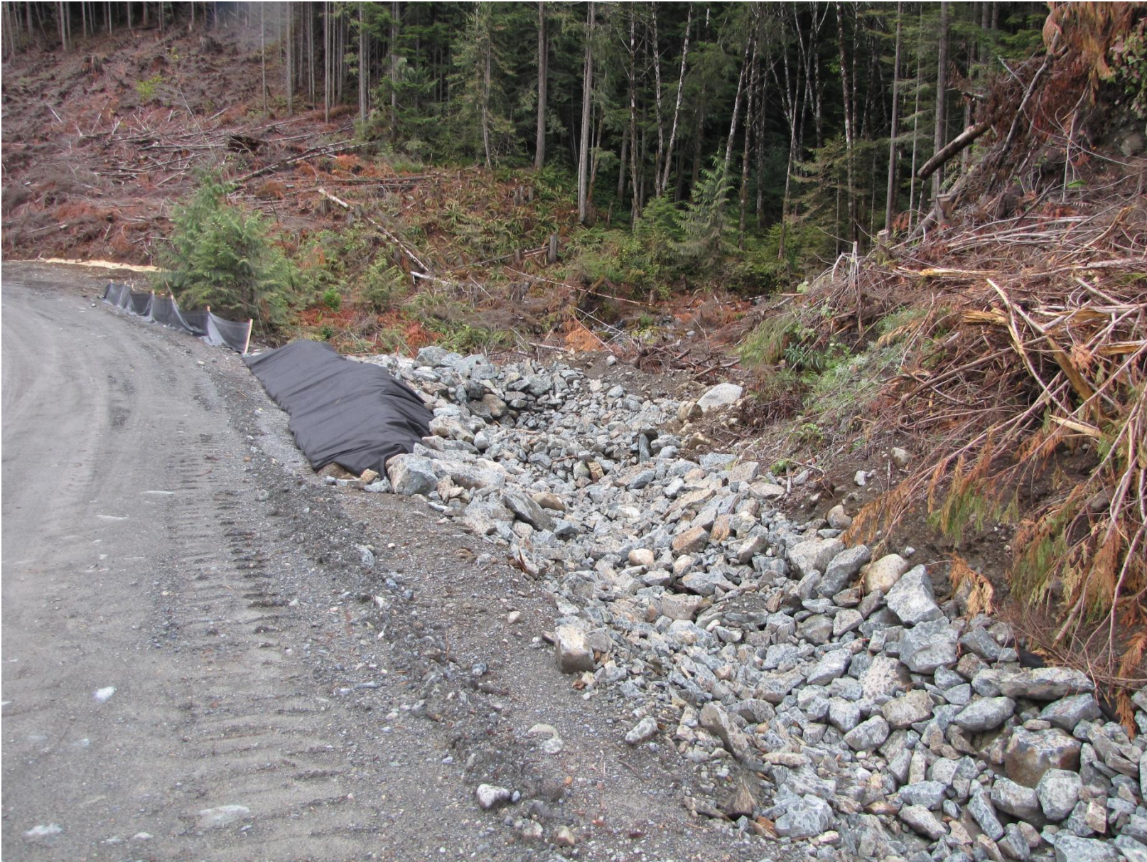
Photo 8 - October 17, ditchline armouring and sump for sediment settling prior to crossing road and flowing into Kokish River.
