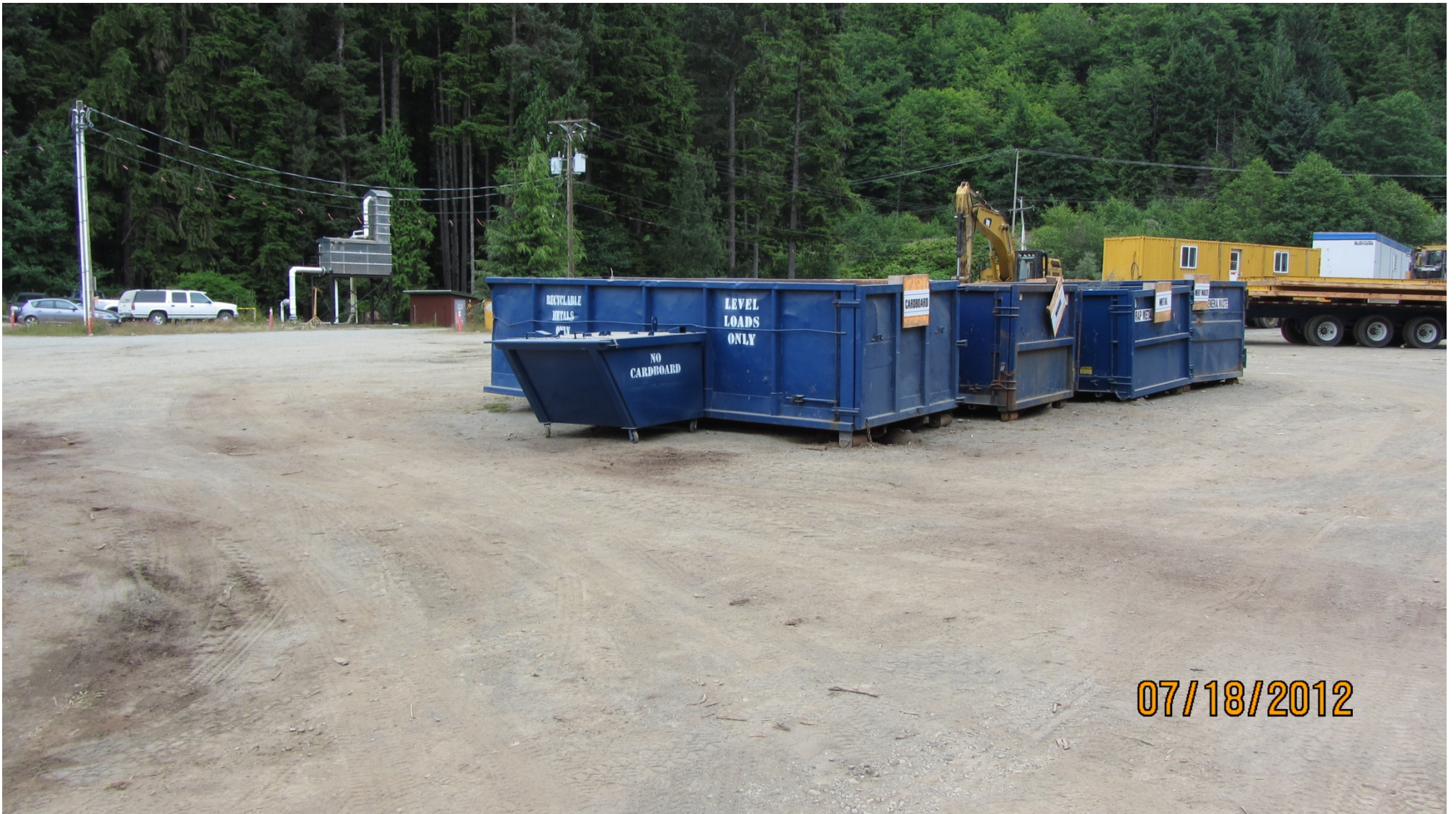
Attachment 5 - Waste Disposal
