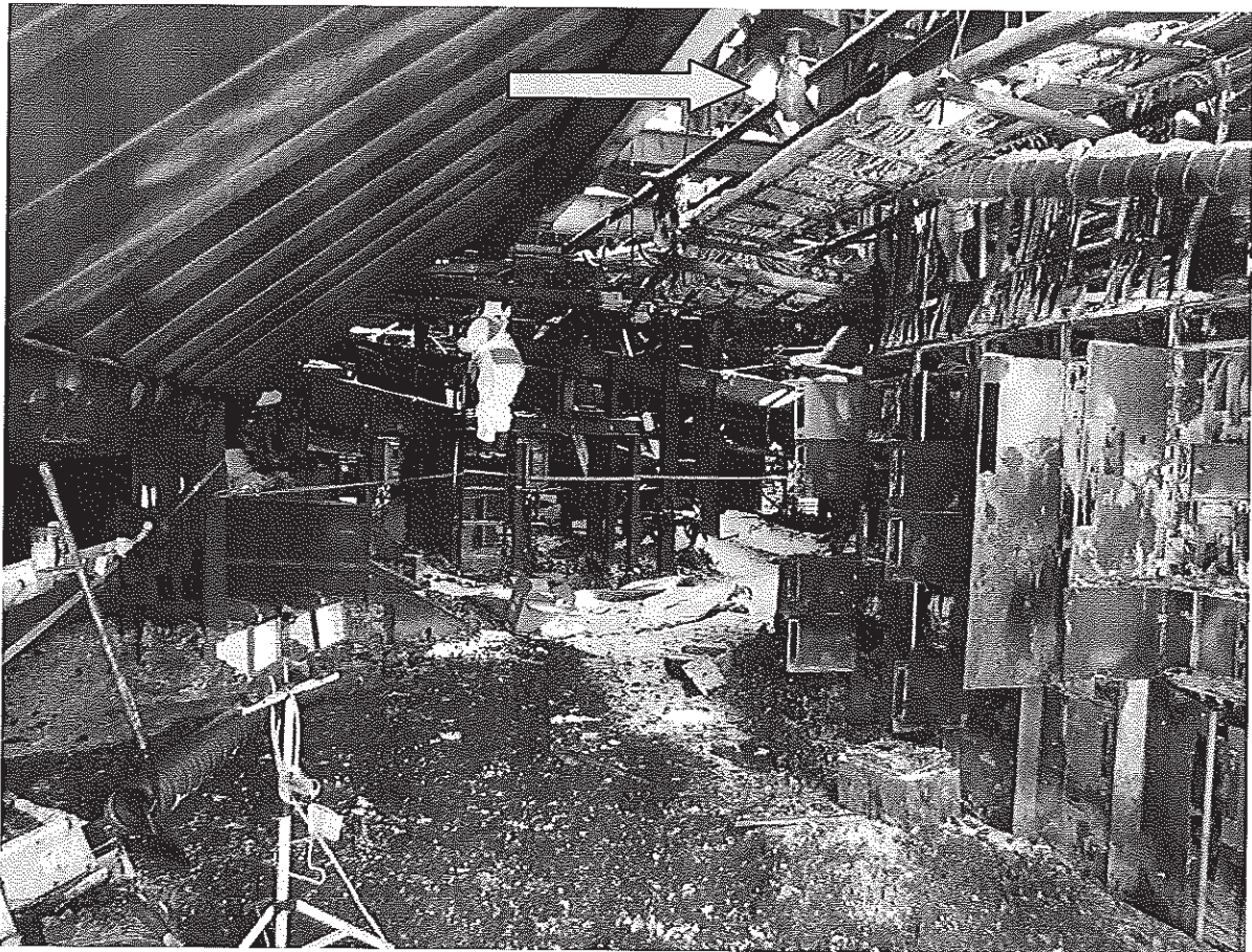
Figure 7: This view looking east from in front of the boiler room (G-15, Appendix 4) shows the MCC-10 electrical cabinet on the right and conveyor 9-92 on the left. The metal halide bulb (yellow arrow) is intact.
