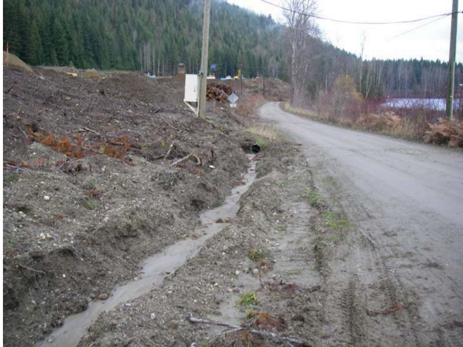
Photograph 2 A view of the silt being transported from the Sugar Lake Road culvert to Sugar Lake.
