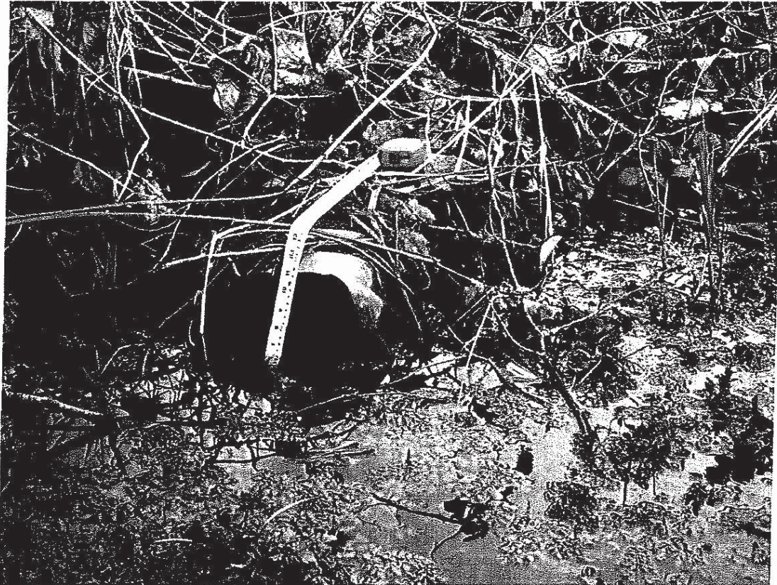
12" culvert south side of Park Drive showing standing water.
