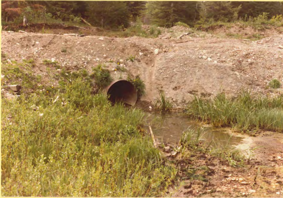
Standing seepage lying below the low level outlet exit.
