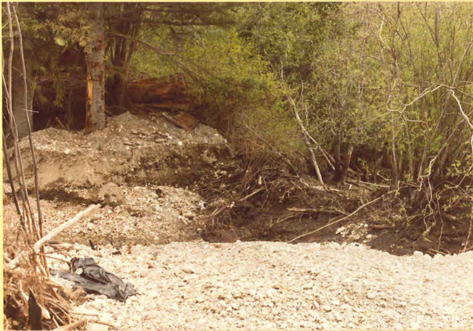
Dam crest showing failure from left.
