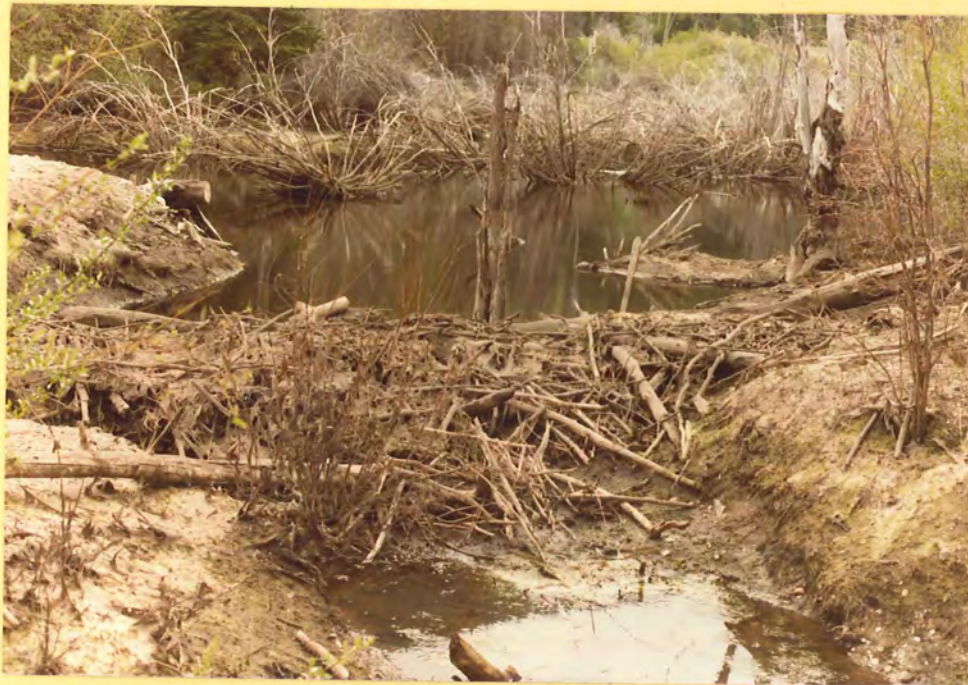
Remains of beaver dam blocking channel to gate works of low level outlet.
