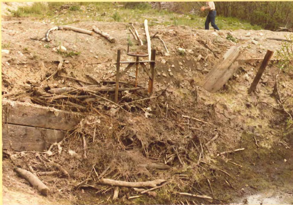
Debris blocking upstream entrance of low level outlet - the valve is still functioning.
