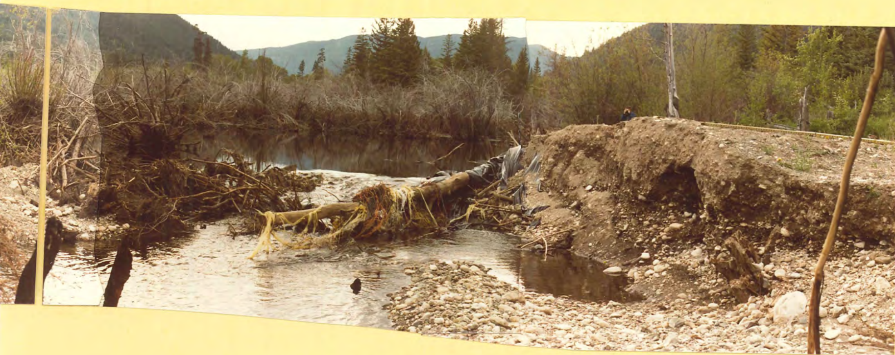
View of dam failure from downstream showing exposed netting and plastic.
