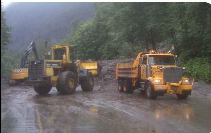
Heavy equipment moves in to remove the fallen debris caused by a mudslide on Highway 1 near Chilliwack. Crews are working to clear the road for traffic.
