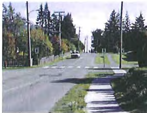
Looking Church Road South at South End of Frontage
