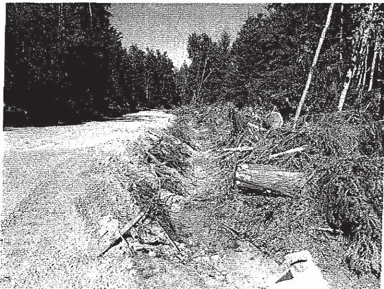
Photo 11, Ditchline 1: This is a newly excavated ditch adjacent to the northeast side of the recently built road that bisects the property. It was dry at the time of the assessment, but would normally flow to the southeast.
