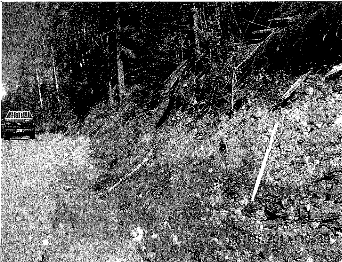
Photo #6 View of failing cutslope and lack of functional ditchline.
