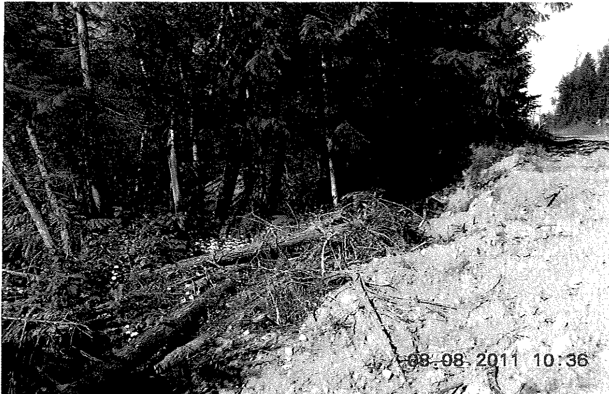
Photo #3 View cutslope slope failure debris pushed over fill slope
