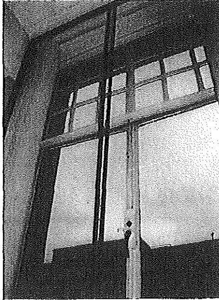
17 Secondary glazing within tea point misaligned.
