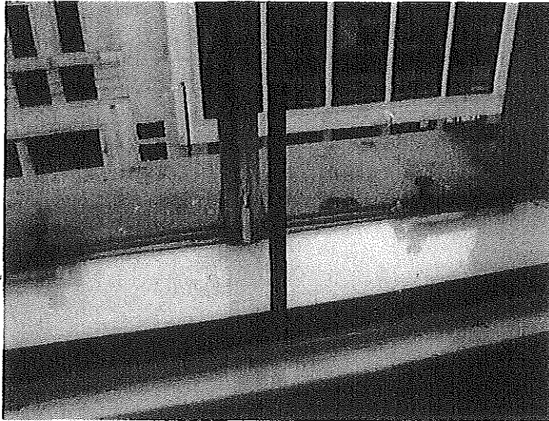
41 Paintwork to window unit within office 5 generally in poor order
