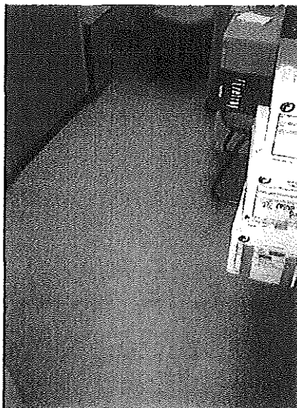
35. Carpet finish within office 4 generally in satisfactory condition although pile slightly worn and discoloured.
