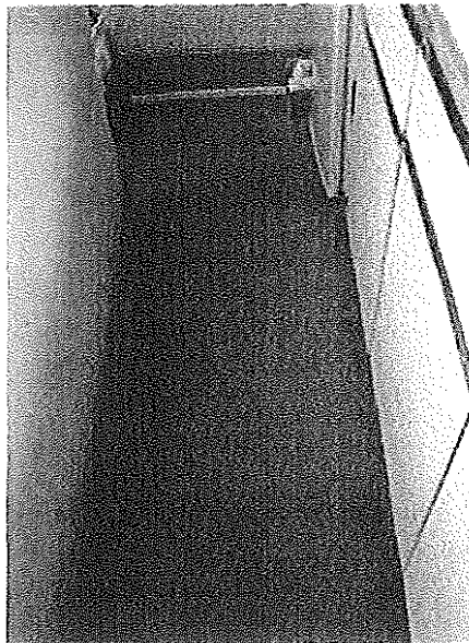
18. Carpet within tea point generally in a soiled condition, especially adjacent fridge and below cupboards. Scuff marks and surface soiling evident at low level on partition.
