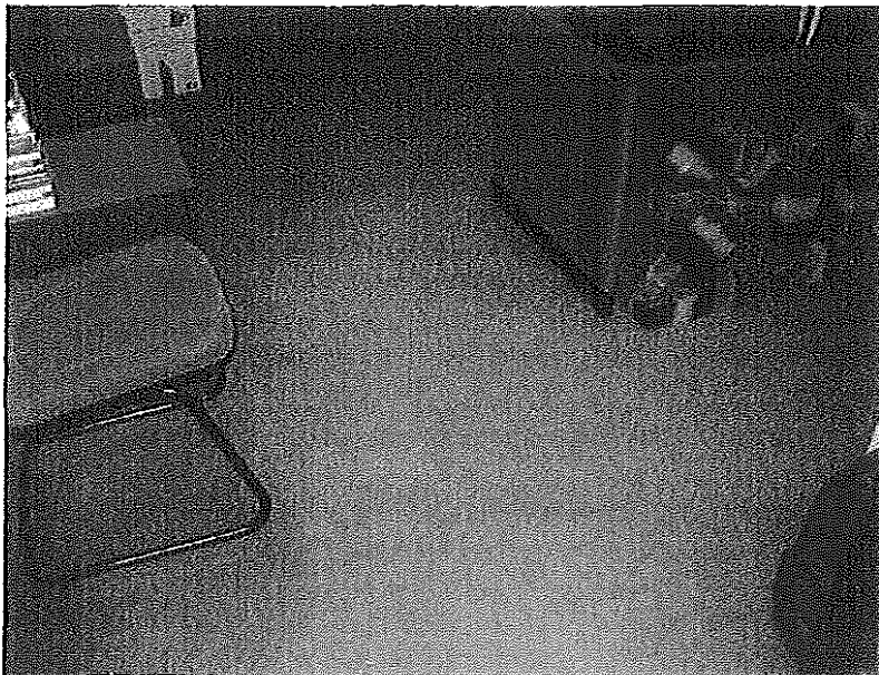
28. Carpet finish within office 3 generally in satisfactory condition although pile is worn and discoloured.
