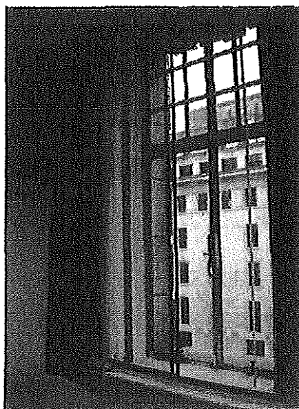
22 Secondary glazing within office 2 misaligned and paintwork to window in poor decorative order
