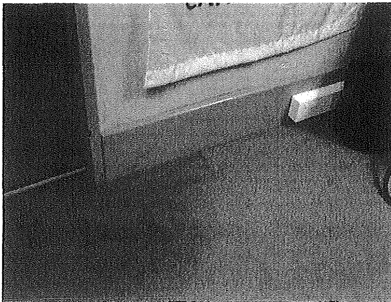
10. Low level paintwork on door frames and skirting's generally scuffed, chips also evident in isolated locations. Generally wallpaper is lightly soiled and marked at low level.
