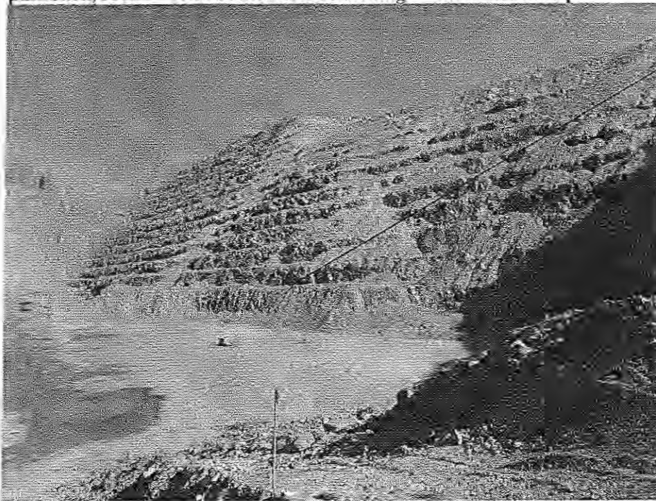
Photo 4 Northwest corner of Springer Pit. Triple bench
