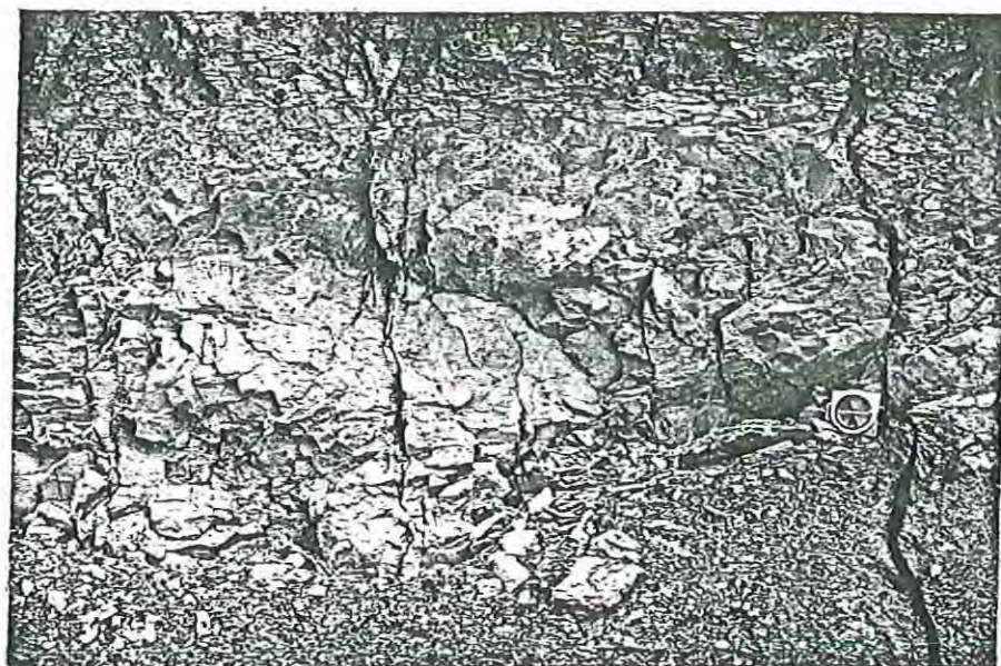
Plate B14 - Heavily-preconsolidated banded silts on Red Bluff.
