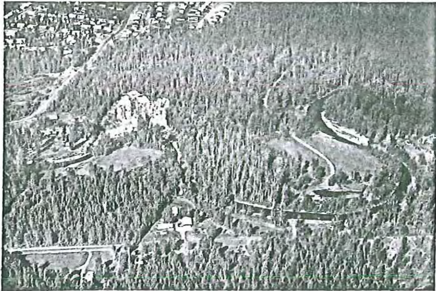
PLATE F25 Baker Creek. One of the Baker Creek Slides in a meander bend.
