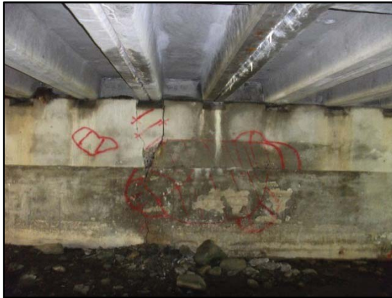
Red marking indicates areas of structural instability at Upper Cambie.
