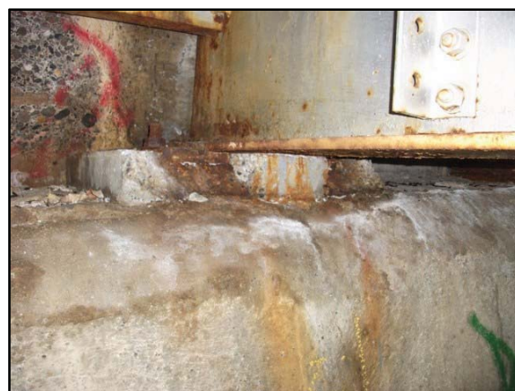
Evidence of rust and damage to the concrete abutment at Lower Cambie.
