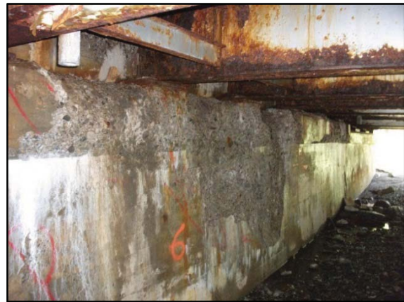
Evidence of rust and damage to the concrete abutment at Upper Cambie.
