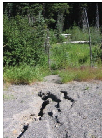
Bank erosion along the northwest fill slope.
