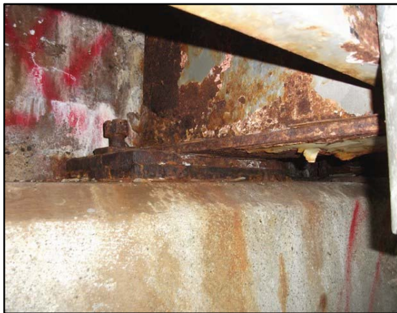
Evidence of rust and damage to the concrete abutment at Middle Cambie.
