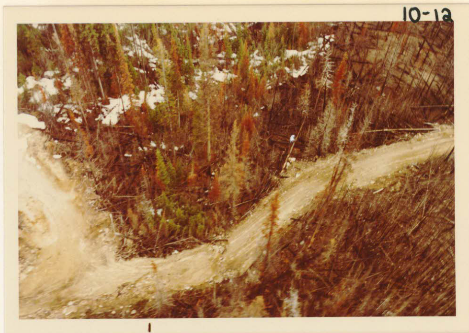
10-12 Washed out creek crossing on fire road on south east side of Pentticton Creek catchment.
