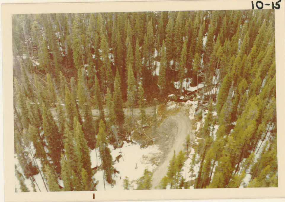
10-15 Wash across fire road on north west side of Penticton creek. No drainage diversion apparent.
