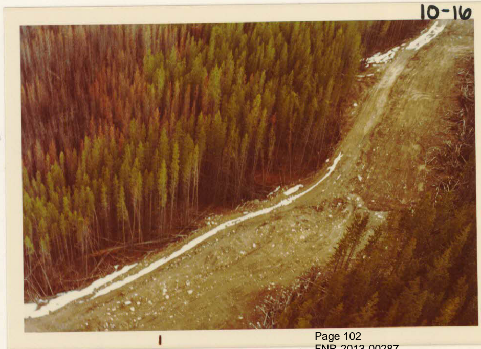
10-16 Erosion on fire guard on north west side of Penticton Creek. Drainage diversion possible.
