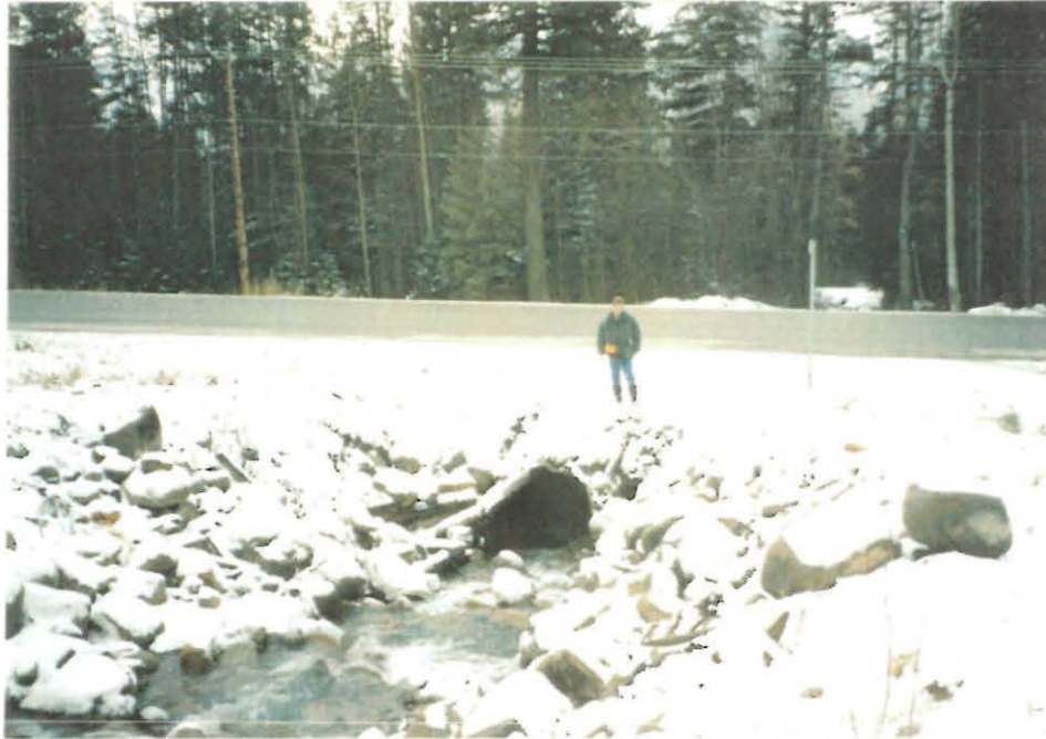
PHOTOGRAPH 1: (Spittal Creek, Nov. 17, 1998): Metal Culvert (1500 mm diam.) at Highway 16.
