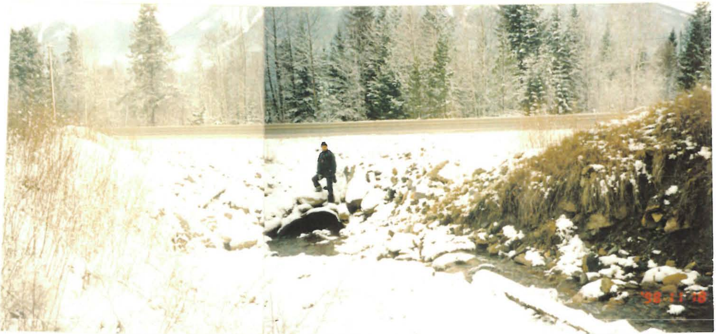
PHOTOGRAPH 7: (Leona Creek, Nov. 18, 1998): Deformed metal culvert (1500mm diameter) at Highway 16.
