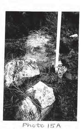
a closer view of the seepage in 19A. The spring accuss right at the tog mear the pregometer stand-pipe,
