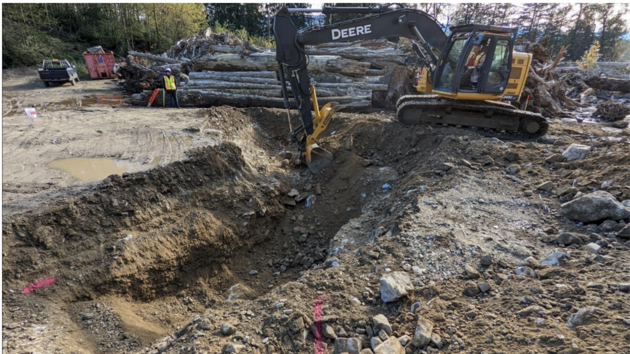
Figure 3 Excavating the test pit
