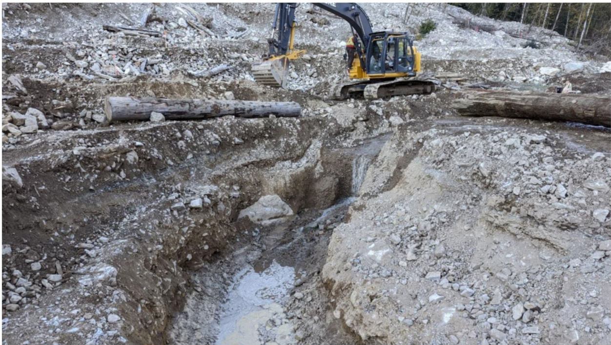
Figure 5 Water flowing into the soakaway (note small water fall in right centre)
