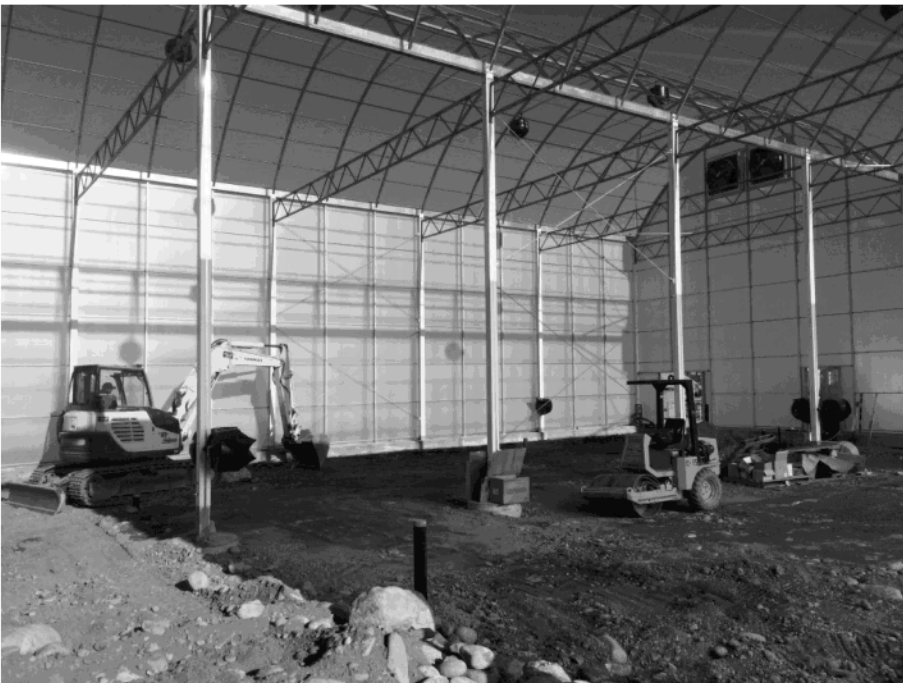
Below: Vertical polycarbonate panels installed and rough grading underway in greenhouse
