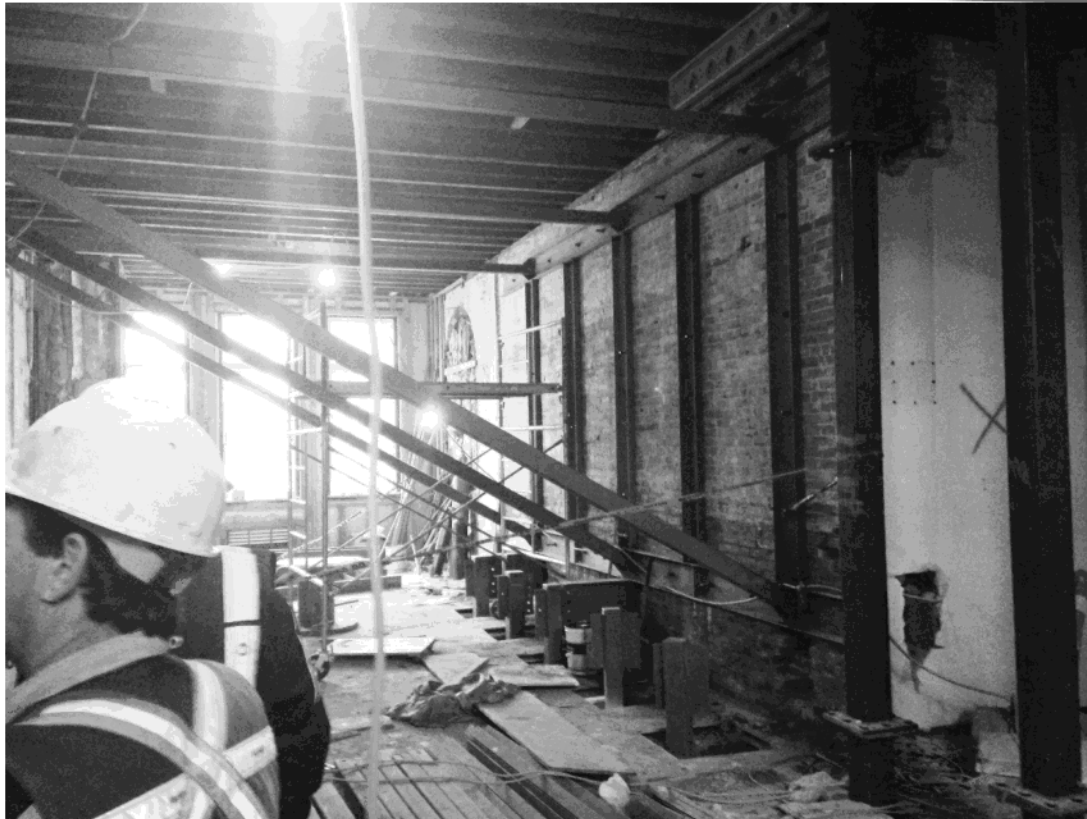
Structural shoring of interior brick walls to be retained above isolation plane
