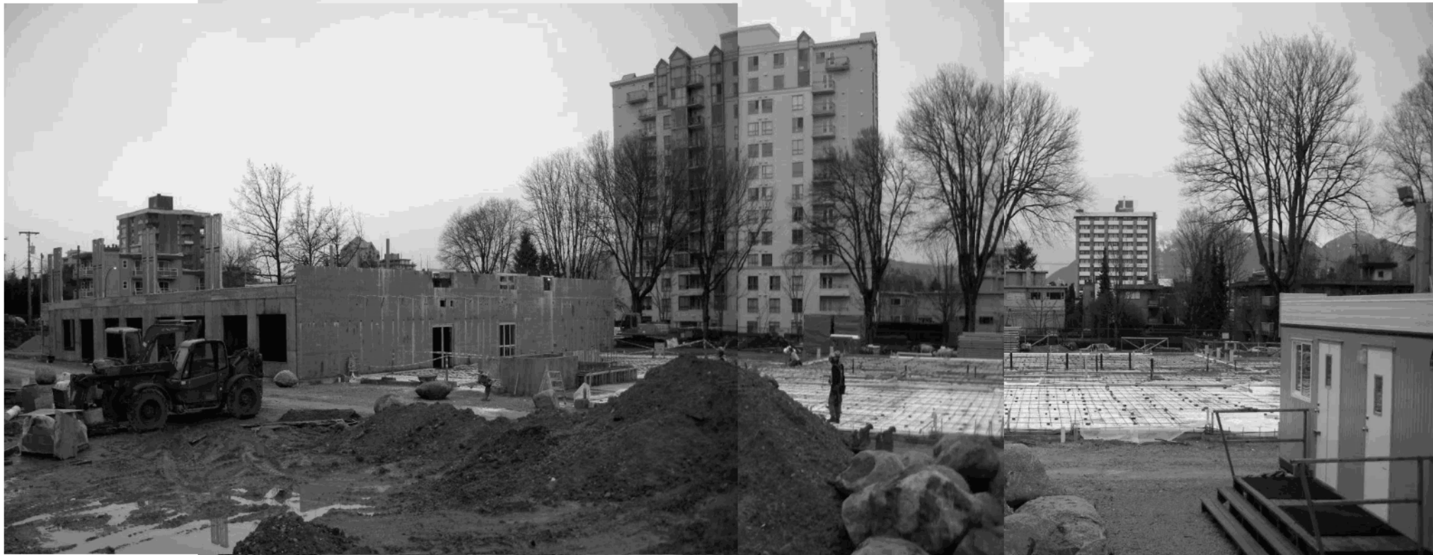
Feb 10: View from Southeast – First floor framing complete. Second floor framing underway.
