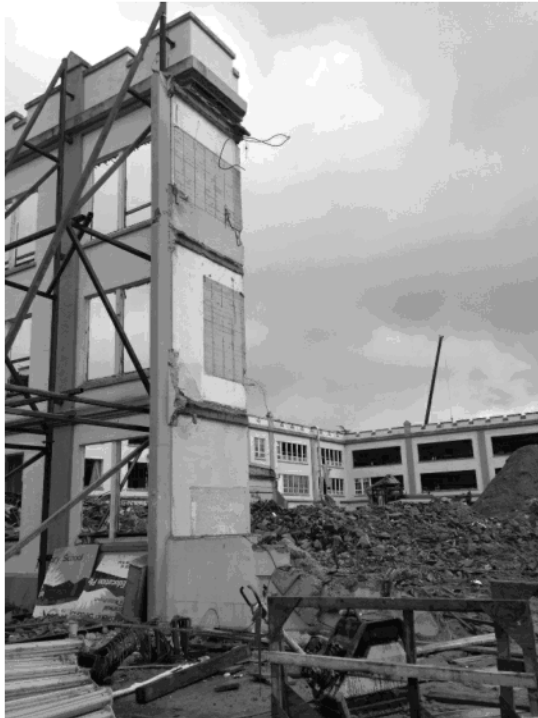
Full demolition while retaining the heritage façade (SW corner)
