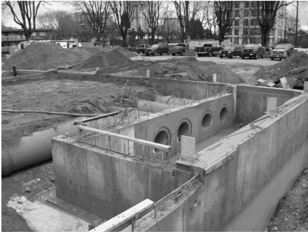
View of earth tubes under MP slab – simplified for cost savings
