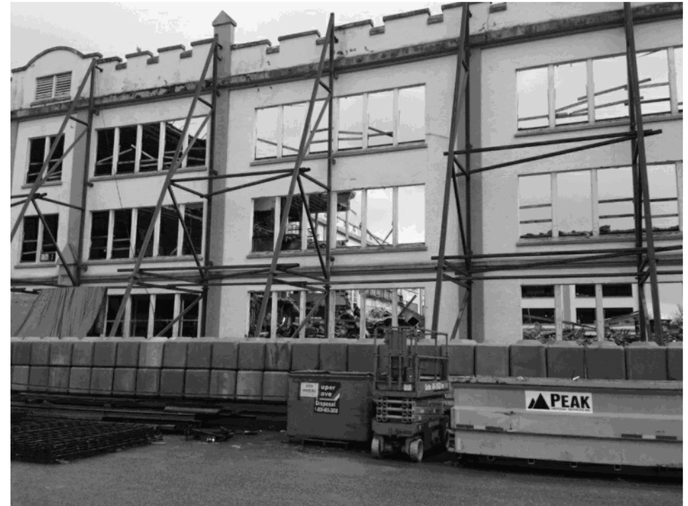
Heritage facade retention with steel bracing and concrete lock blocks (west façade)
