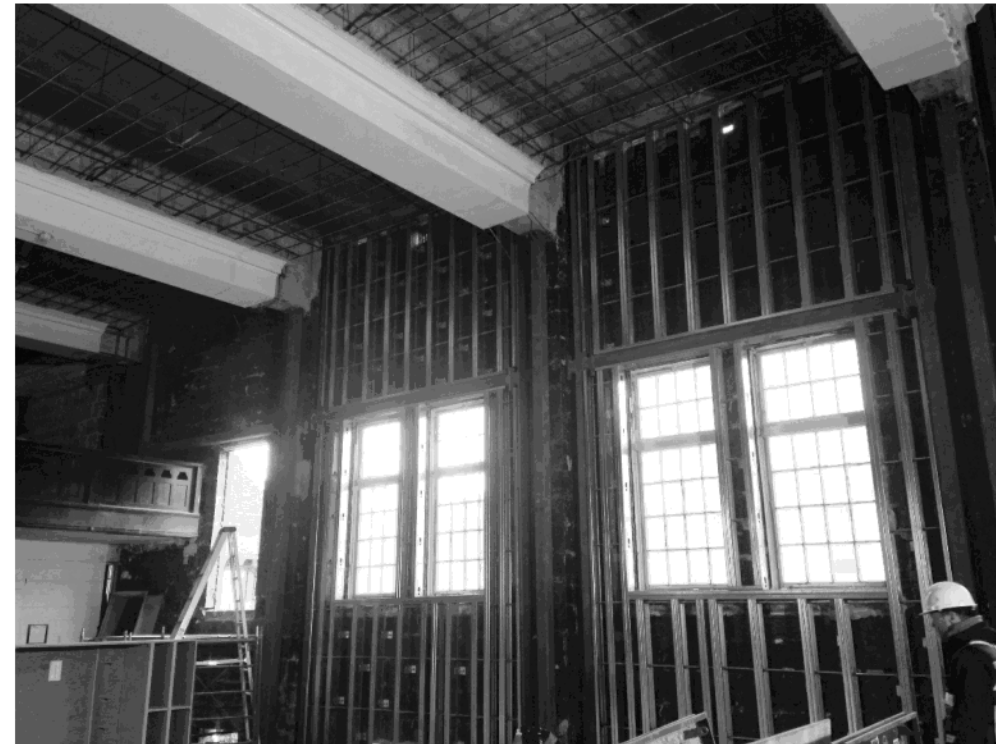
Interior struc. steel and steel studs (auditorium level)
