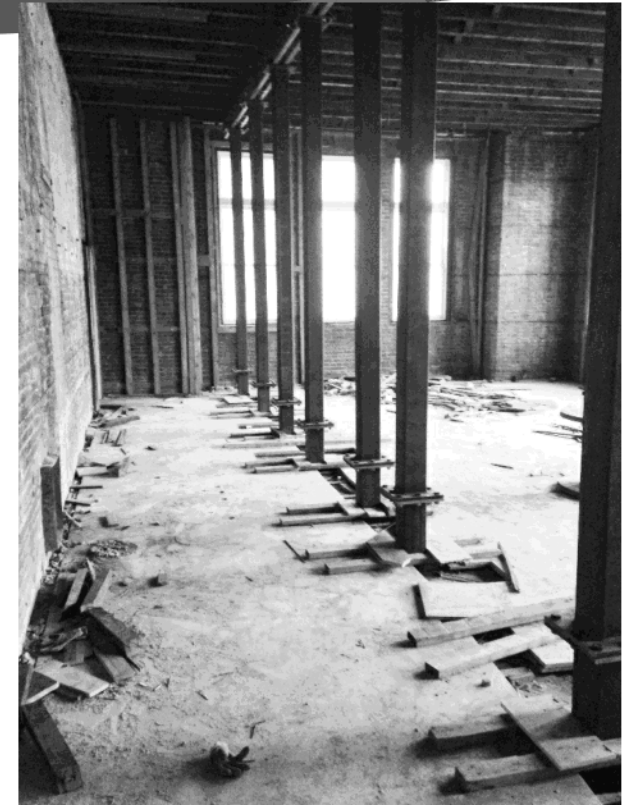
Structural Shoring of Building C complete
