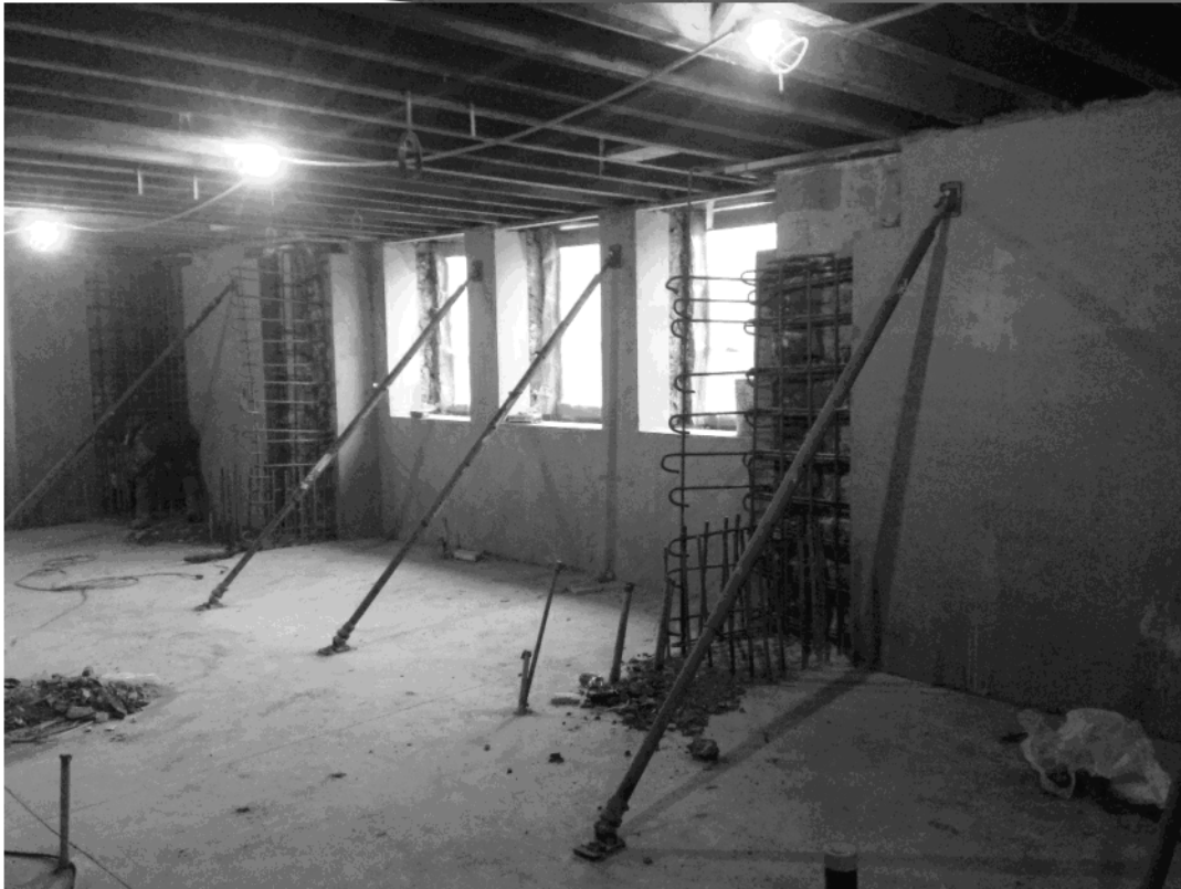
Slab on grade and shotcrete exterior walls complete in basement. Reinforcing steel in place for concrete columns that support Isolators
