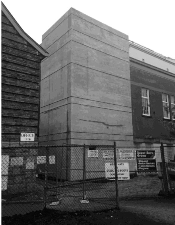
Exterior concrete shearwalls (photo taken from Pender St)
