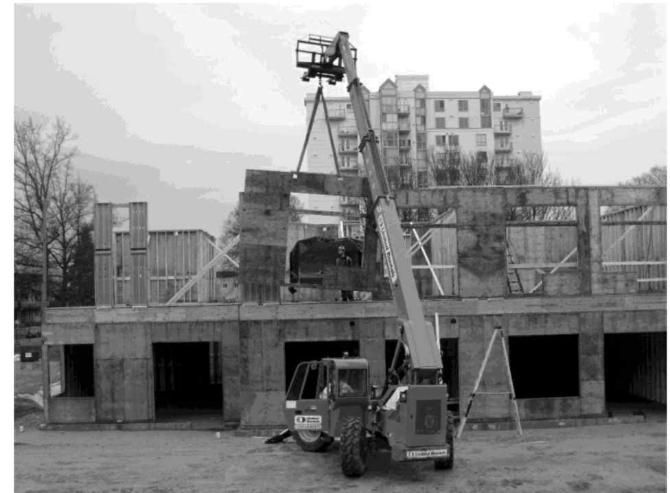
Feb 12: Installation of prefabricated walls underway
