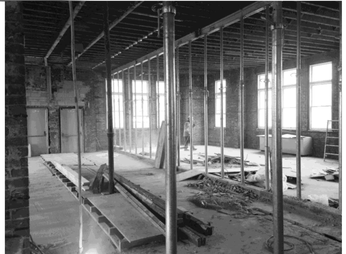
Structural demolition of interior brick walls on Upper Level complete
