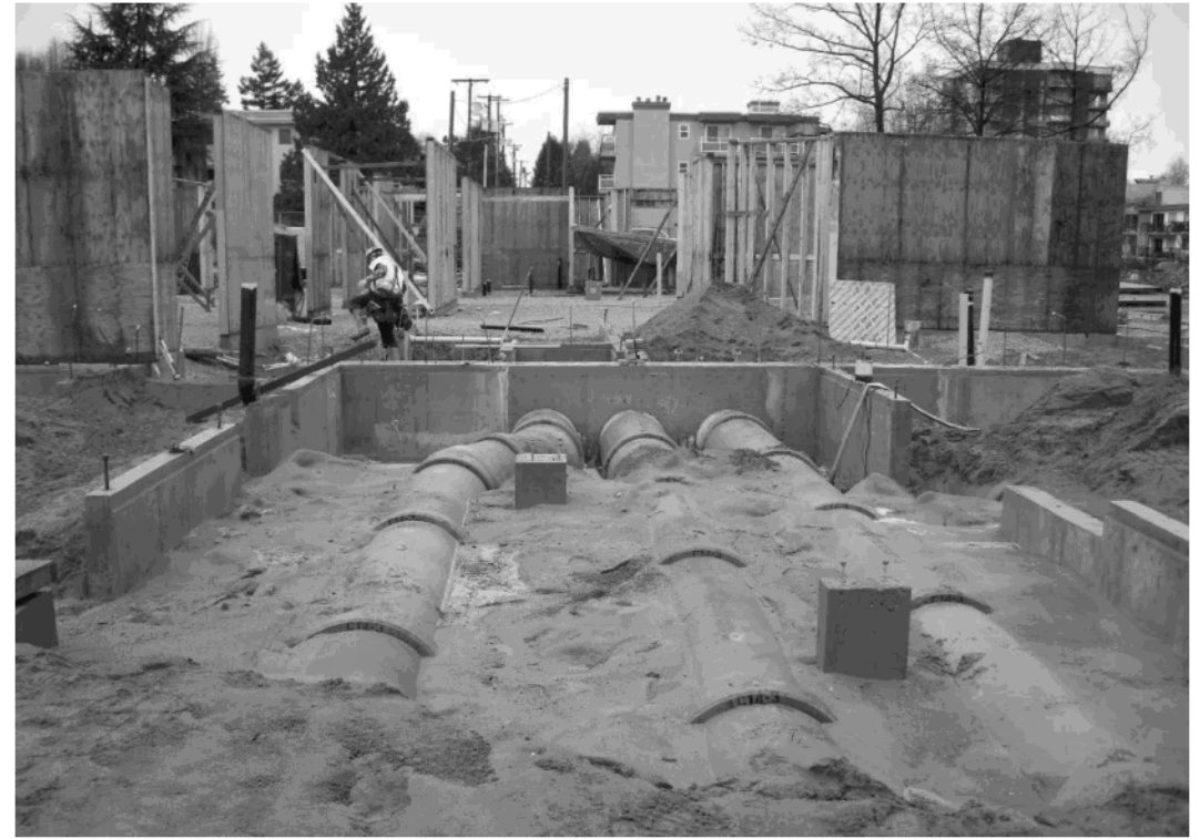
View of earth tubes under gym slab – simplified for cost savings
