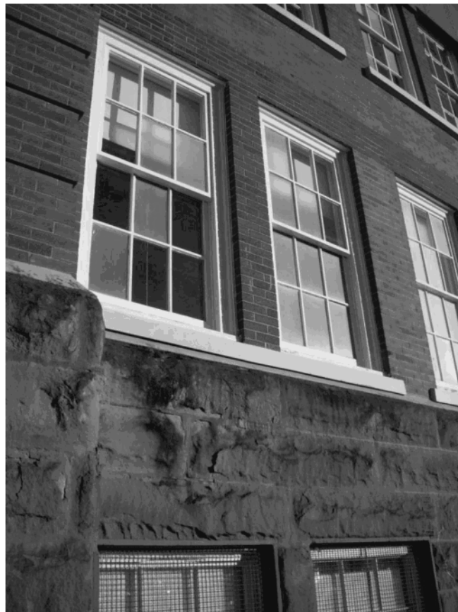
Figure 14: Close-up of Brick and Sandstone Façade
