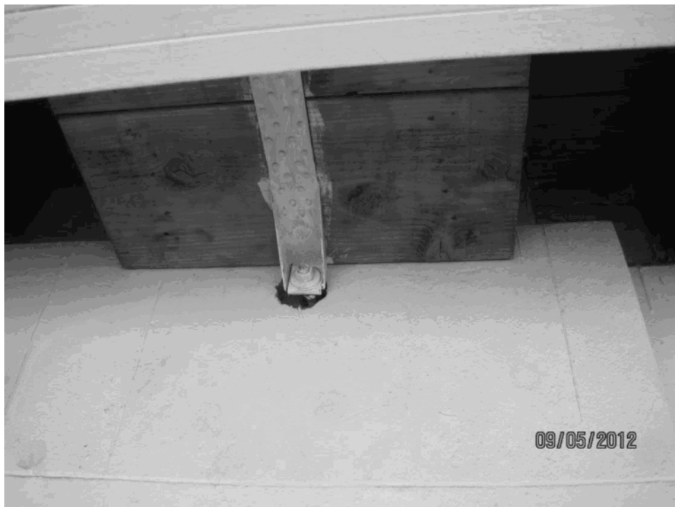
Figure 8: Play Area Cover Attachment to Classroom Wall
