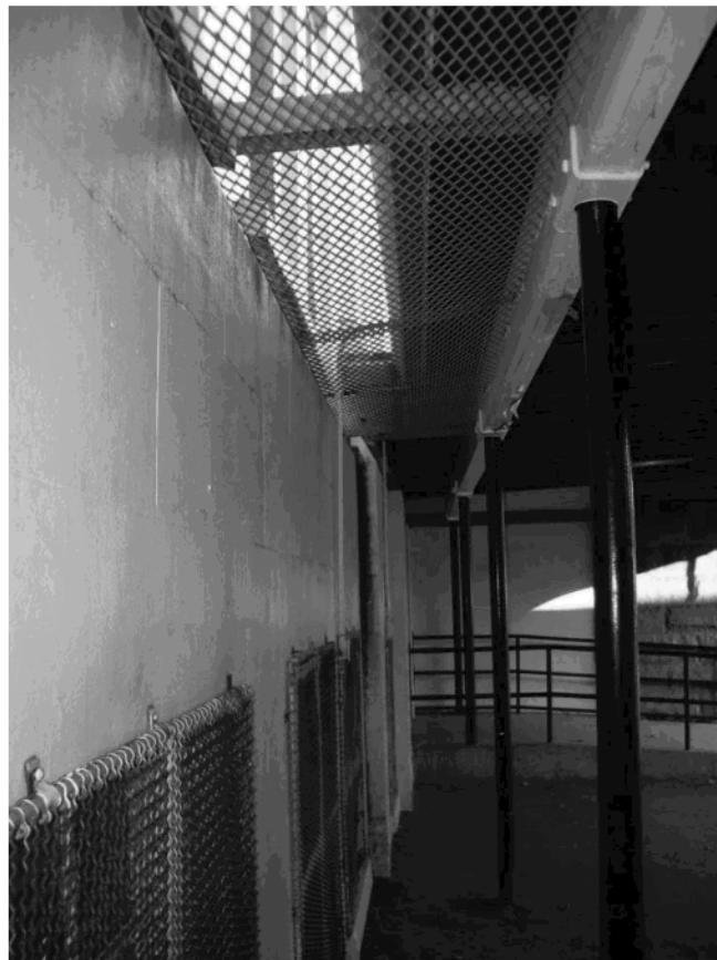
Figure 10: Gap Between Cover and South Wall of Classroom Block
