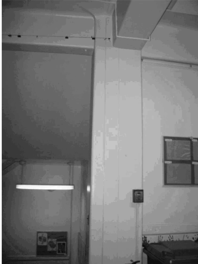
Figure 21: Joint between Phases of Classroom Block Construction
