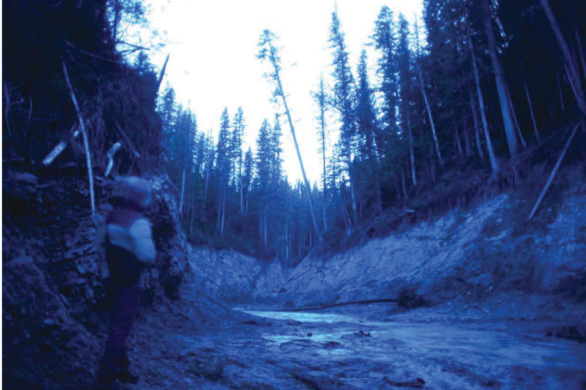
Figure 5: Soil instability caused by scouring of cliffs during tailings flow slide, April 5th 2015
