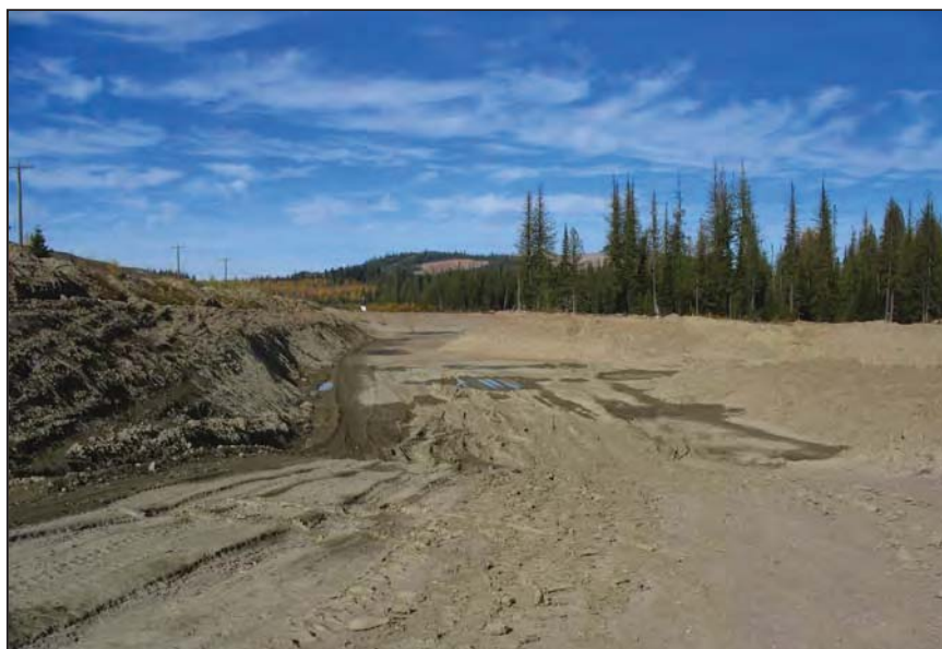
PHOTO 4 – Glacial Till borrow Downstream of Perimeter Embankment.
