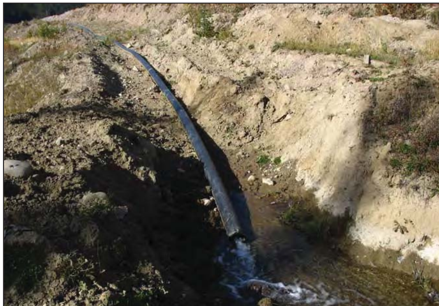
PHOTO 15 – South Embankment Upstream Toe Drain flow.
