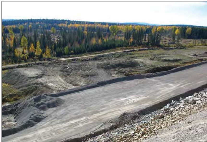
PHOTO 10 – Main Embankment Buttress.
