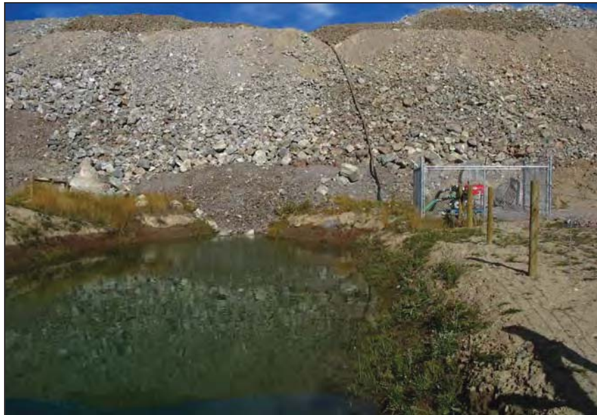
PHOTO 14 – South Embankment Seepage Collection and Recycle Pond.
