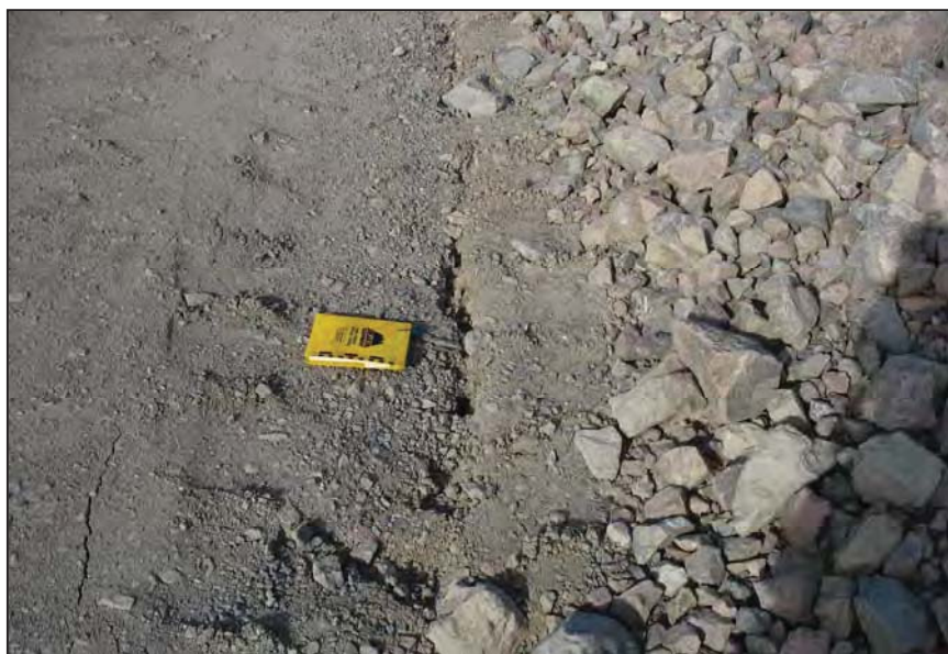
PHOTO 6 – Tension Crack at the Perimeter Embankment.
