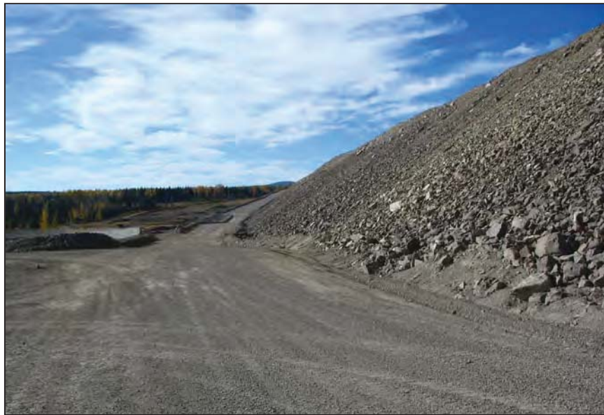
PHOTO 8 – Downstream Slope of Main Embankment.
