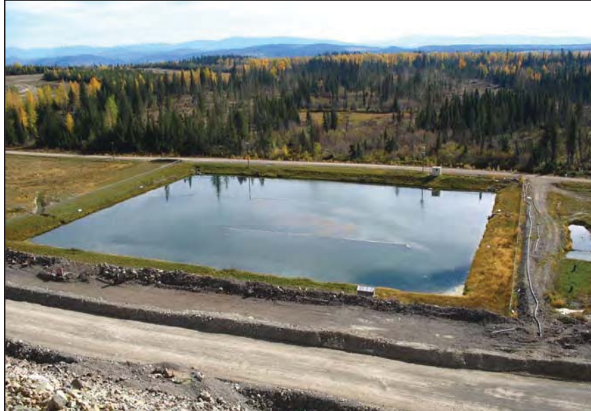
PHOTO 9 – Main Embankment Seepage Collection and Recycle Pond.
