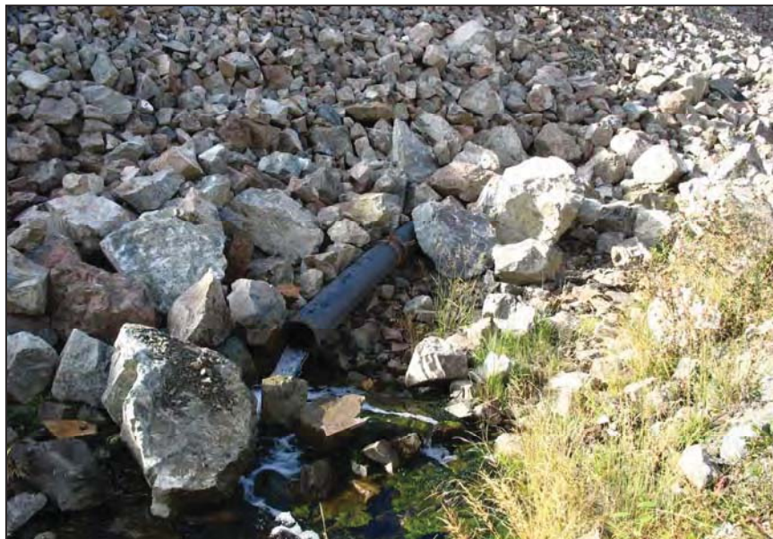
PHOTO 3 – Perimeter Embankment Toe Drain Flow.
