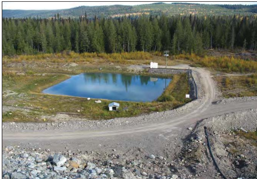
PHOTO 2 – Perimeter Embankment Seepage Collection and Recycle Pond.
