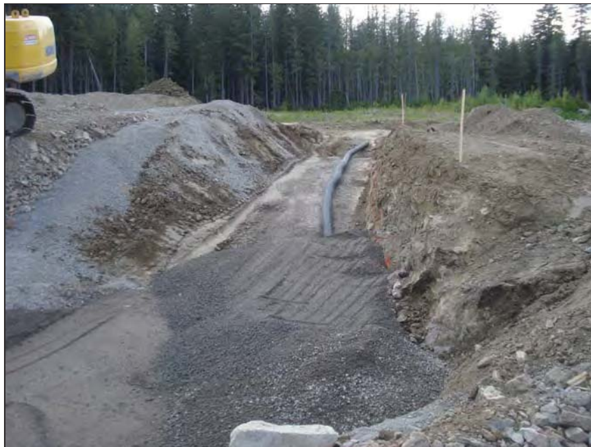
PHOTO 18 – Toe drain extension on the South Embankment abutment
