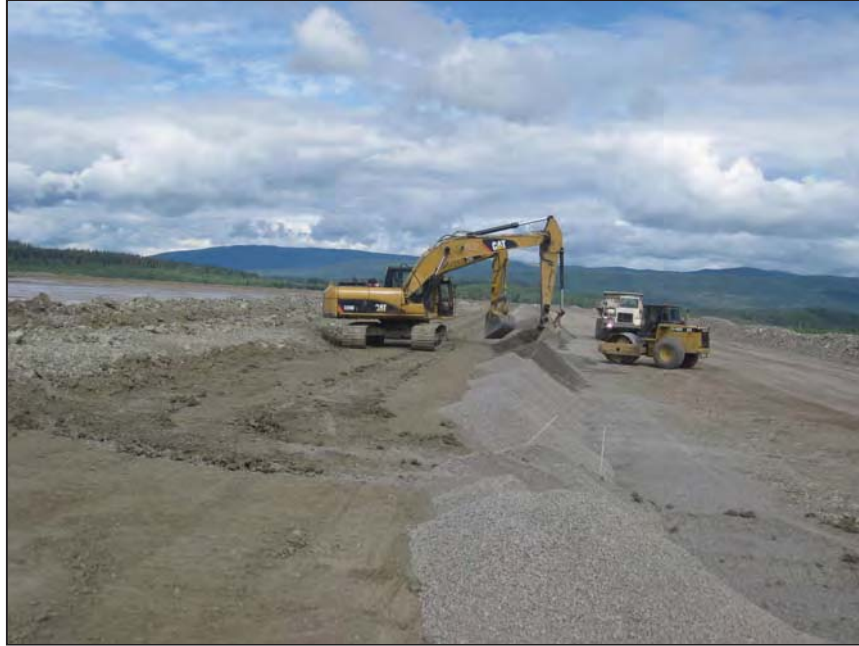
PHOTO 9 – Placement of Zone F filter material on the South Embankment
