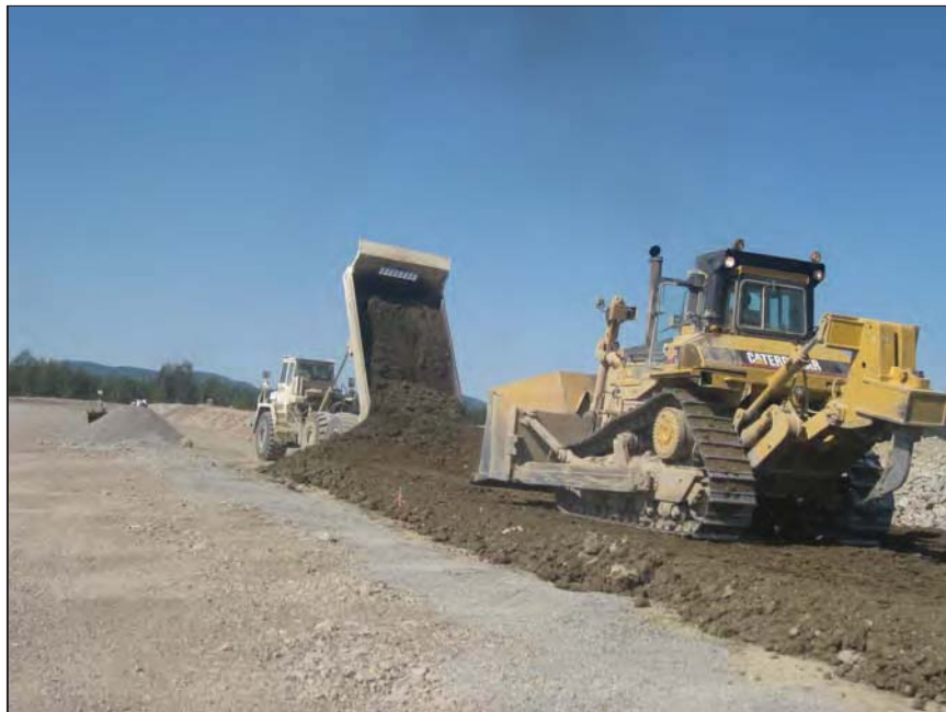
PHOTO 4 – Placement of till material on the Main Embankment
