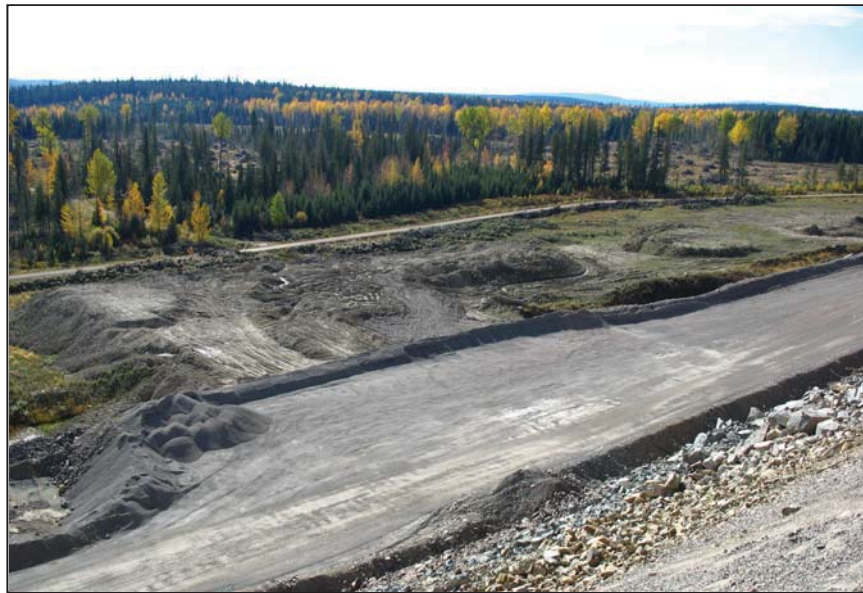
PHOTO 10 – Main Embankment Buttress.
