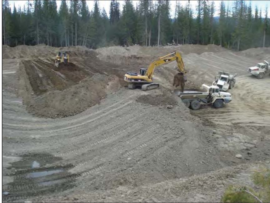
PHOTO 3 – Haulage of till material from the Perimeter Embankment borrow pit
