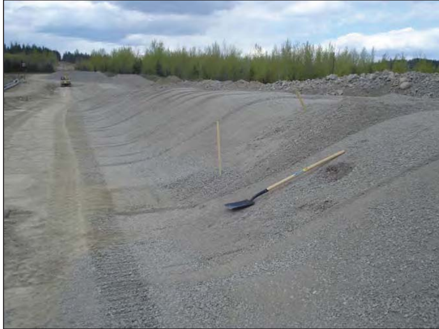
PHOTO 11 – Record sampling of the Zone F filter material on the Perimeter Embankment
