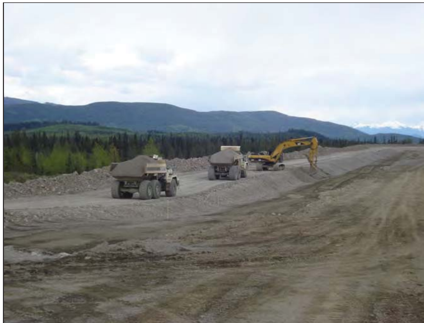
PHOTO 8 – Placement of Zone F filter material on the Perimeter Embankment
