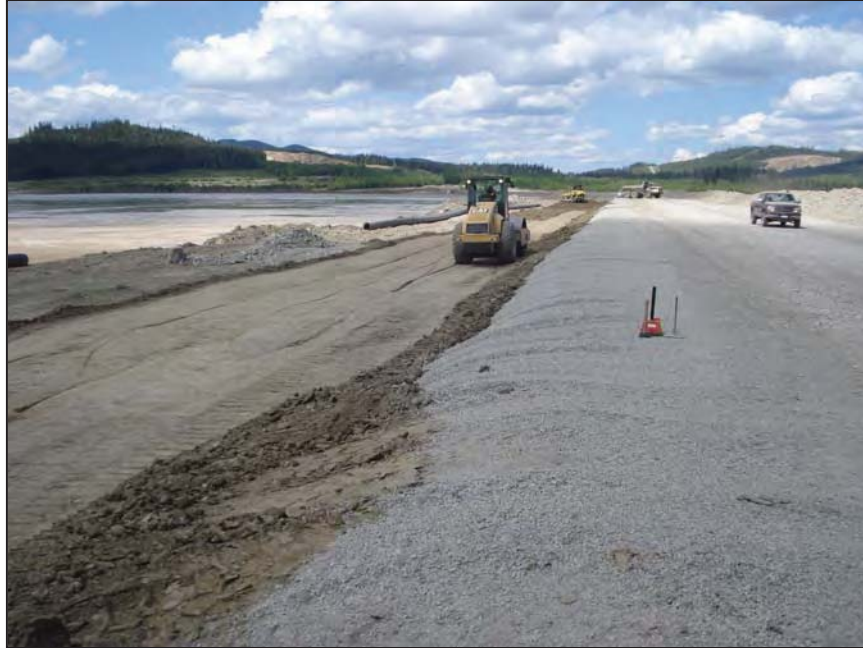
PHOTO 5 – Compaction of till material on the Perimeter Embankment
