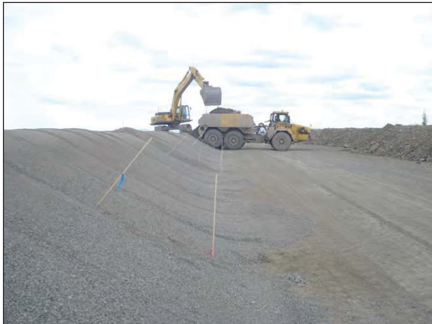
PHOTO 12 – Placement of Zone T transition material on the South Embankment
