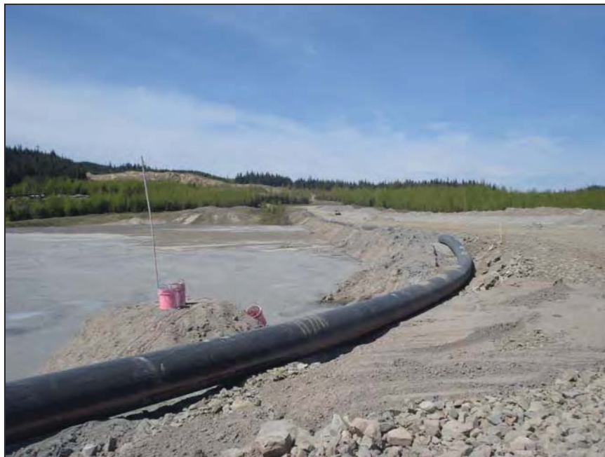
PHOTO 19 – Tailings beach piezometers on the Perimeter Embankment
