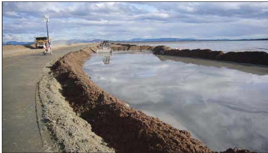
PHOTO 2 – Sand cell construction on the Perimeter Embankment
