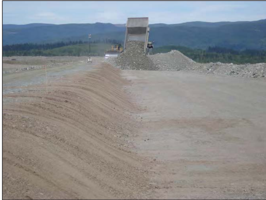
PHOTO 15 – Zone C NAG waste rock material placed in 2 m lifts
