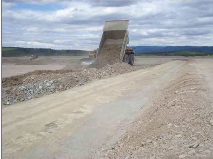
PHOTO 17 – Placement of Zone U material on the Main Embankment using the mine fleet
