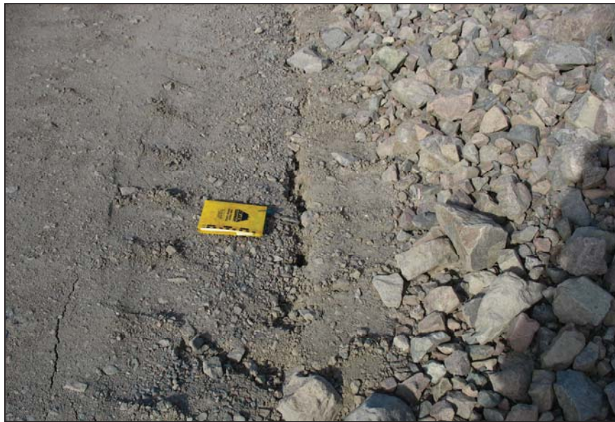
PHOTO 6 – Tension Crack at the Perimeter Embankment.
