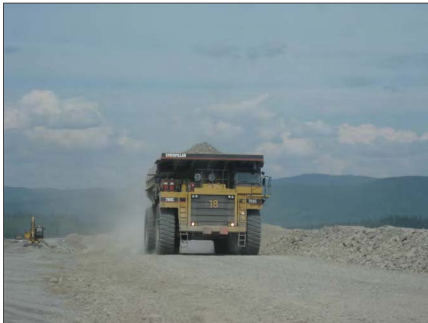
PHOTO 14 – Zone C NAG waste rock hauled to the Main Embankment using the mine fleet
