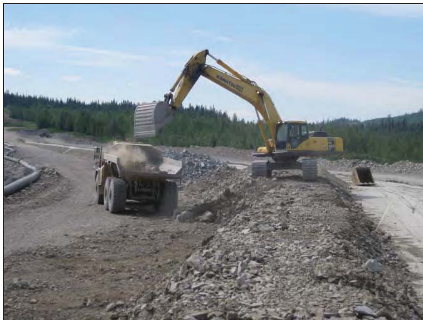
PHOTO 16 – Construction of Zone U waste rock berm for future sand cell construction on the Perimeter Embankment
