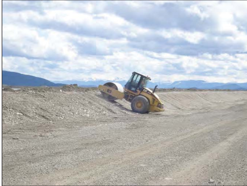
PHOTO 13 – Compaction of Zone T transition material on the South Embankment
