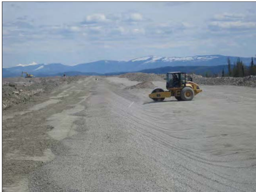
PHOTO 10 – Compaction of Zone F filter material on the South Embankment
