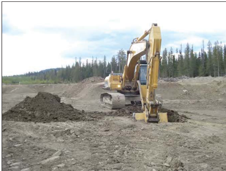
PHOTO 6 – Control sampling of the till material at the Perimeter Embankment borrow pit
