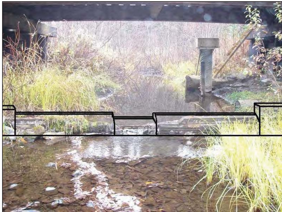
PHOTO 2 – Existing Weir and Approximate Profile of New Weir Structure.
