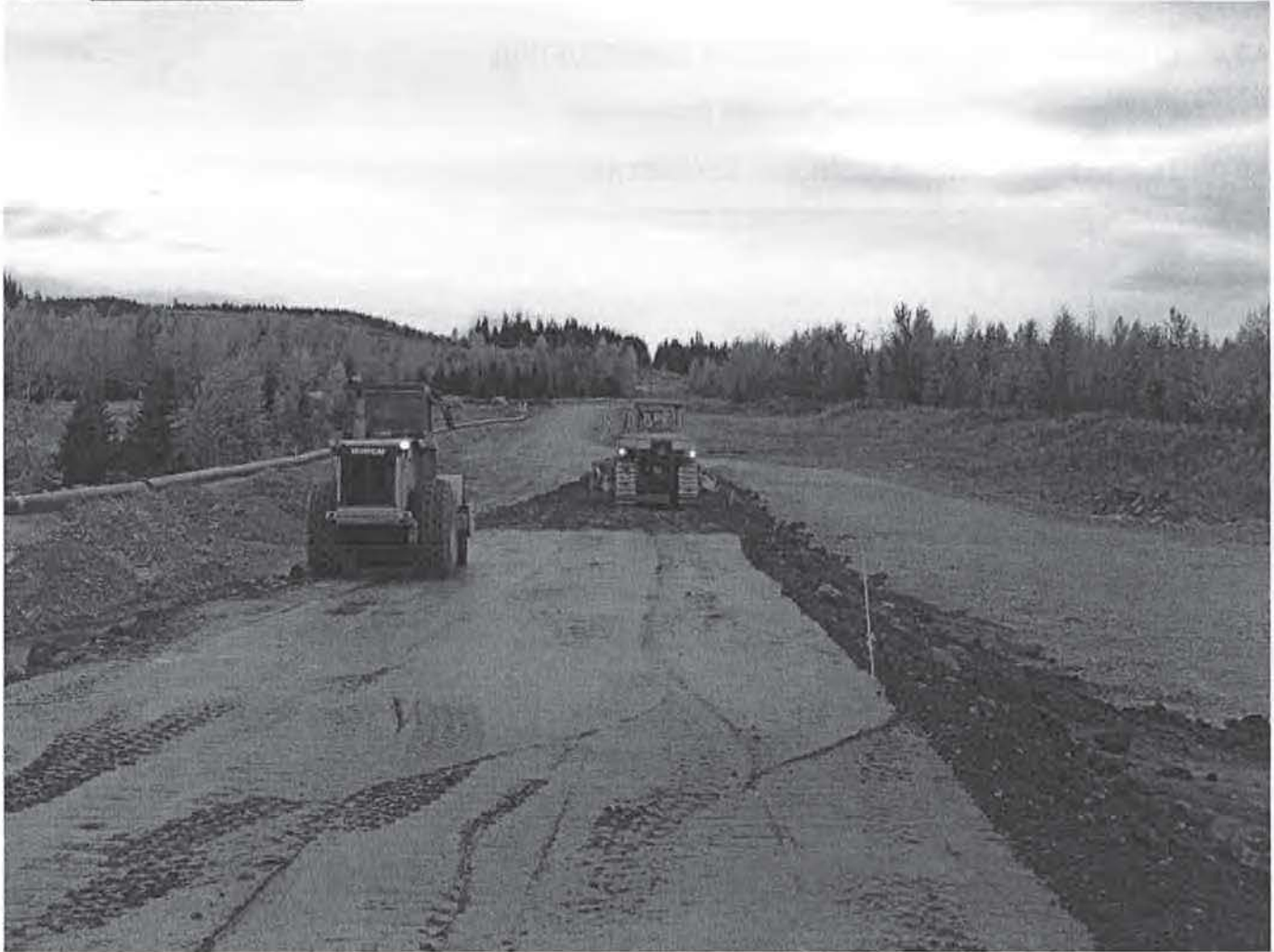
Photo 4: Till placement on the Perimeter Embankment at Ch. 46+00 m.
