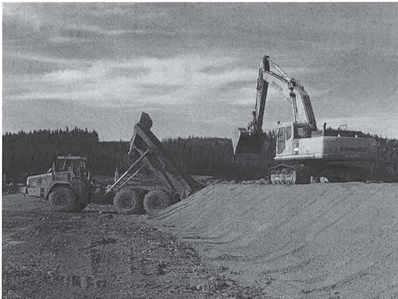
Photo 5: Zone F and T placement to elevation 954 on 2:1 slope.
