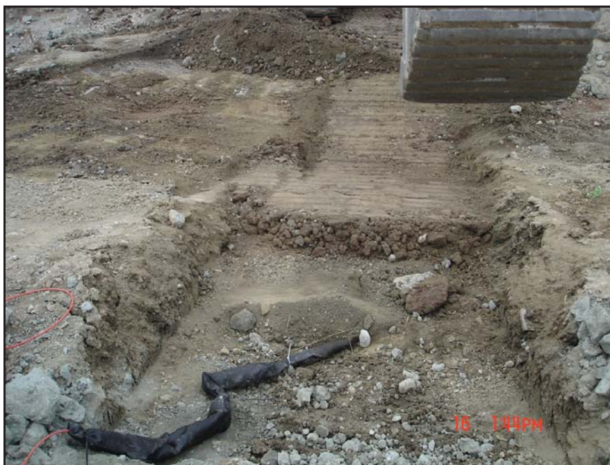
Photo 4: Cable placed approximately 0.5 m under surface of Zone S slope.
