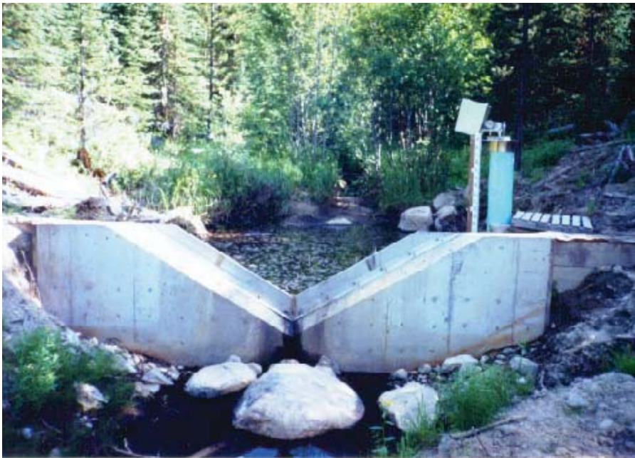
Figure G-6. 120° stainless steel weir plate set in re-enforced concrete. Whitehead Creek below Whitehead Lake (Summerland District water supply).
