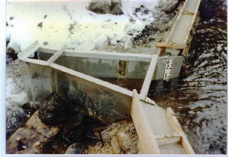
Figure C-33. Six-inch Montana flume set in permanent concrete sack structure.
