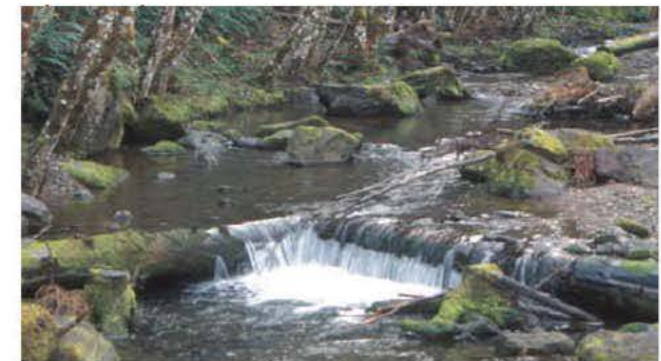
Typical Log Weir Construction
