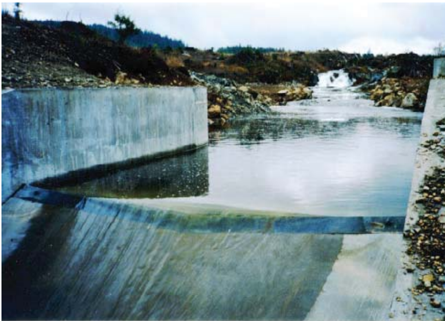
Figure B-2. Pool formed by a modified Crump Weir, where both a digital and an analogue recorder are installed. Judge Creek, Victoria Water Board. The crest has been formed with a shallow vee to increase low flow sensitivity.
