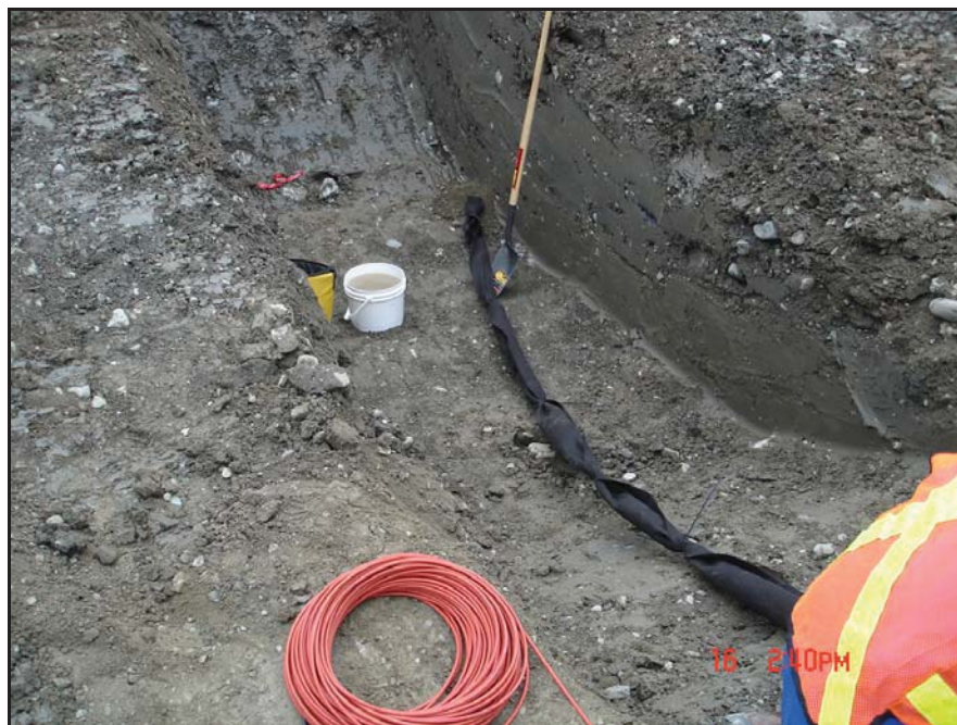
Photo 2: Cable wrapped in geotextile
