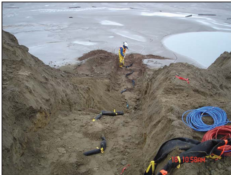
Photo 6: Installing piezometer in tailings sand on ME.
