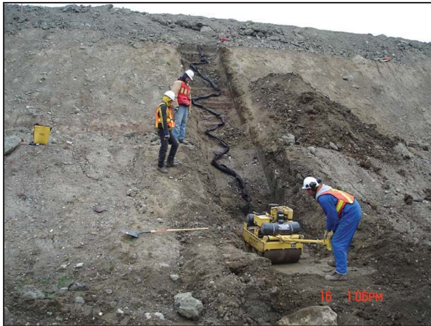
Photo 3: Material packed on top of cable with 2 tonne roller.
