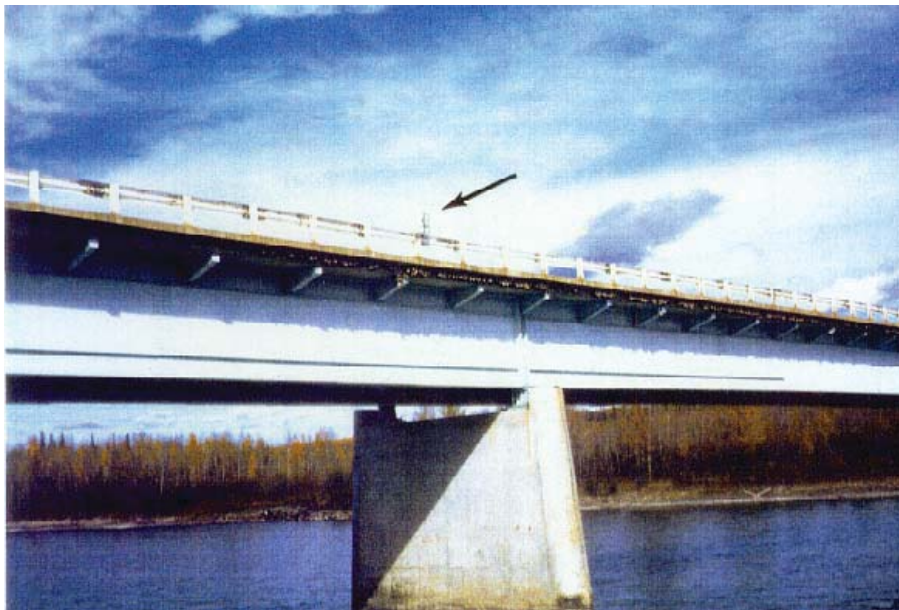
Figure B-15. Wire-weight gauge mounted to a bridge rail. Bear River, near Stewart.
