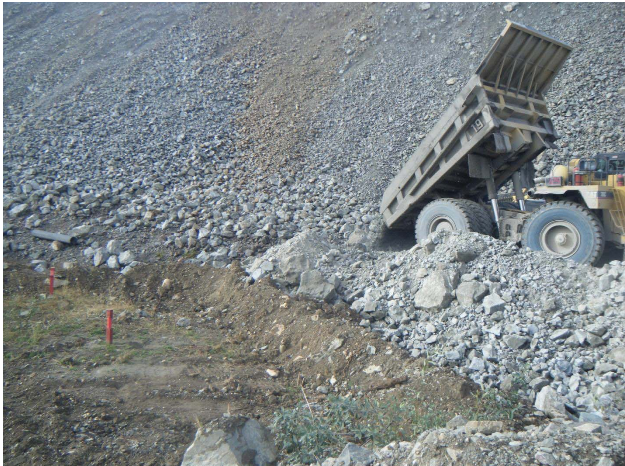
Spreading C Zone material to create buttress below PE.
