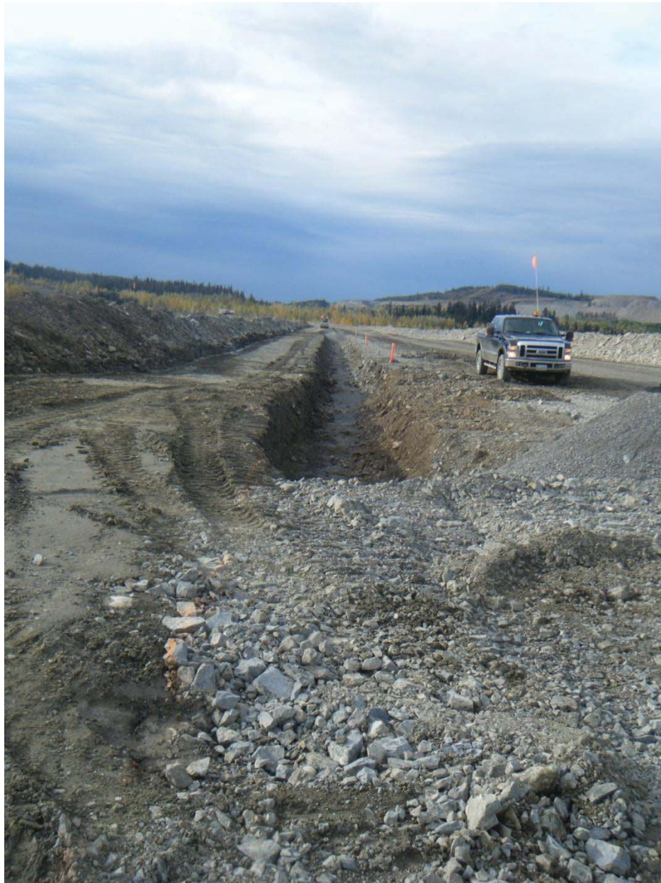
Filter trench being excavated along PE
