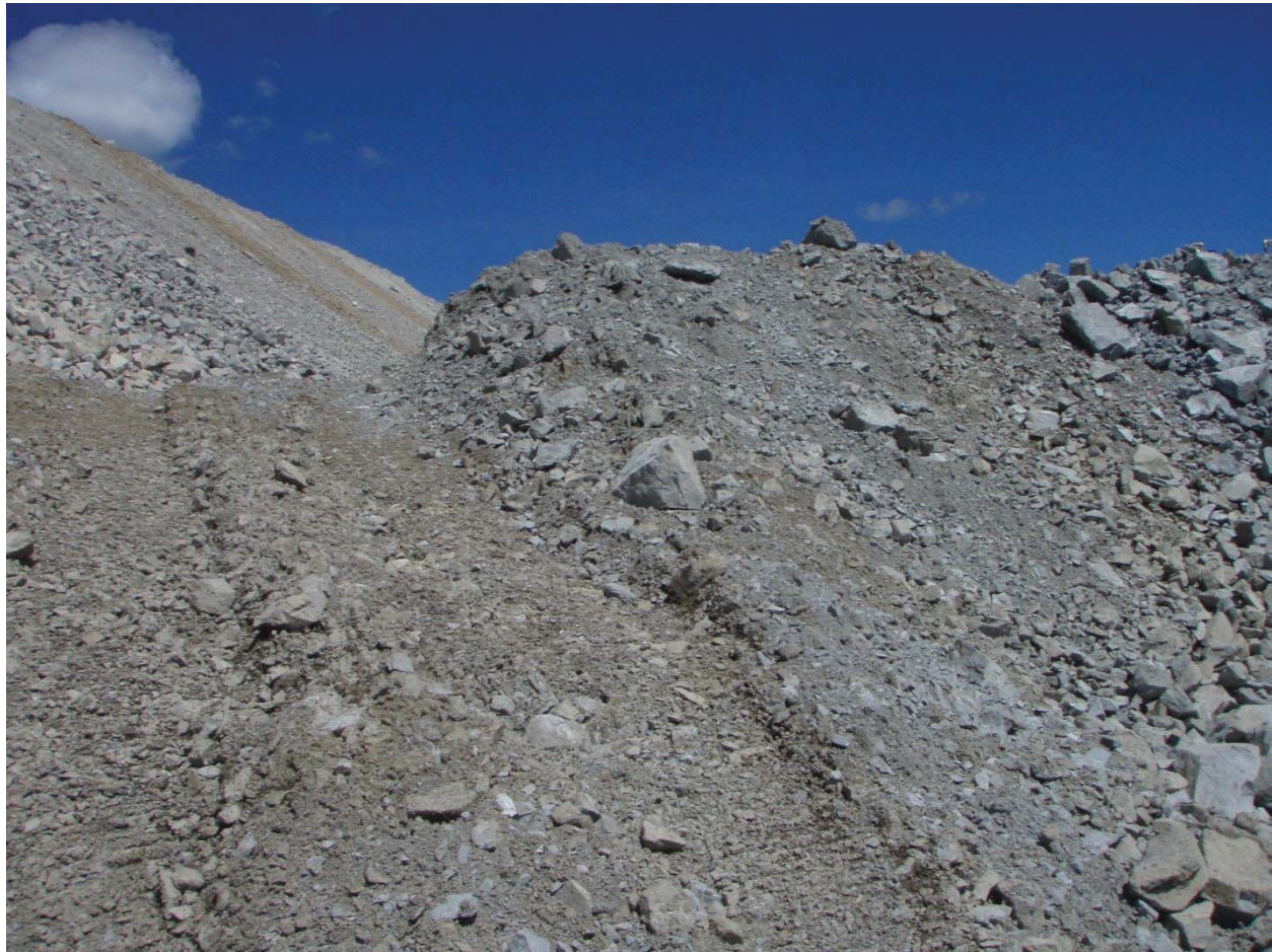
Buttress construction below ME
