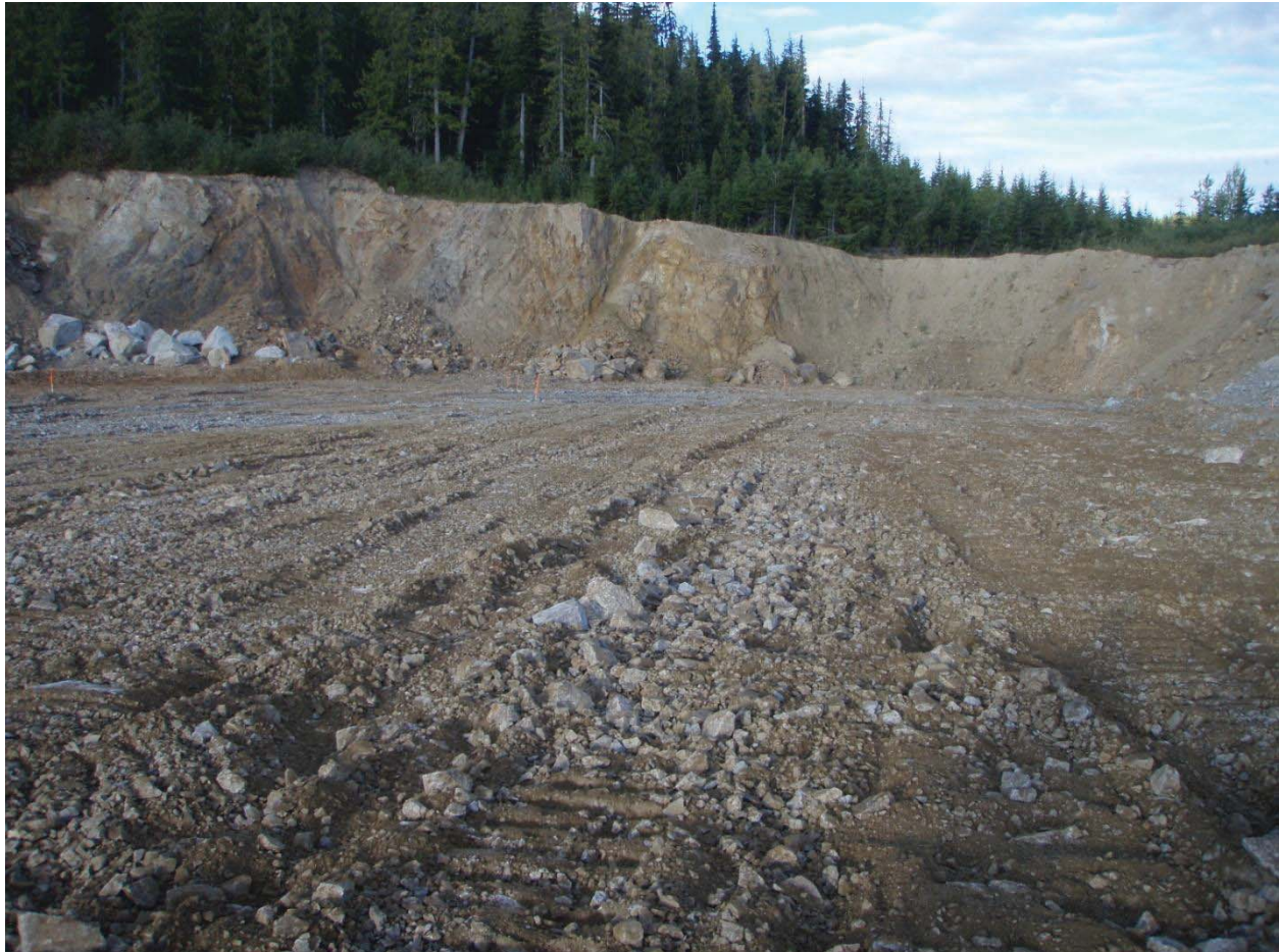
Spreading C Zone material in quarry to reach Elev 1030.1
