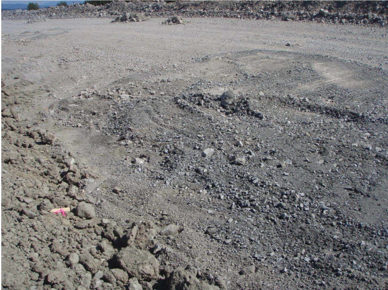
Trench after coarse material removed and Transition material filled
