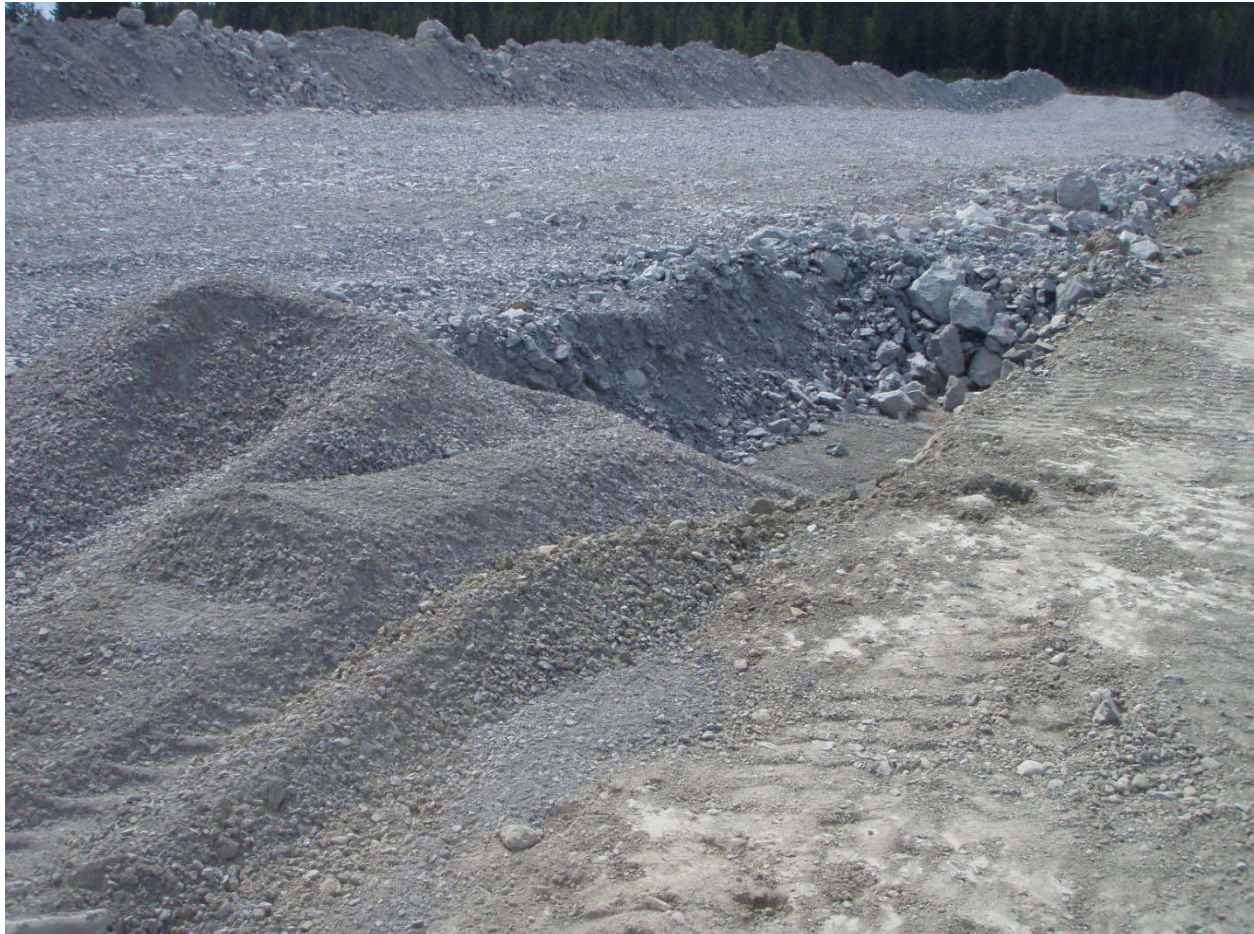
Trench filled with filter material to station 0+840
