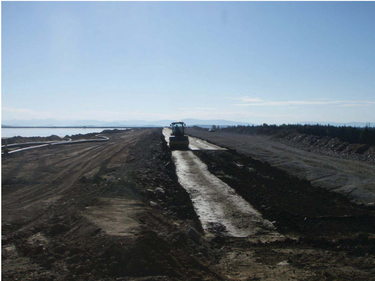
Vibrating roller compacting till on SE (lift #7)
