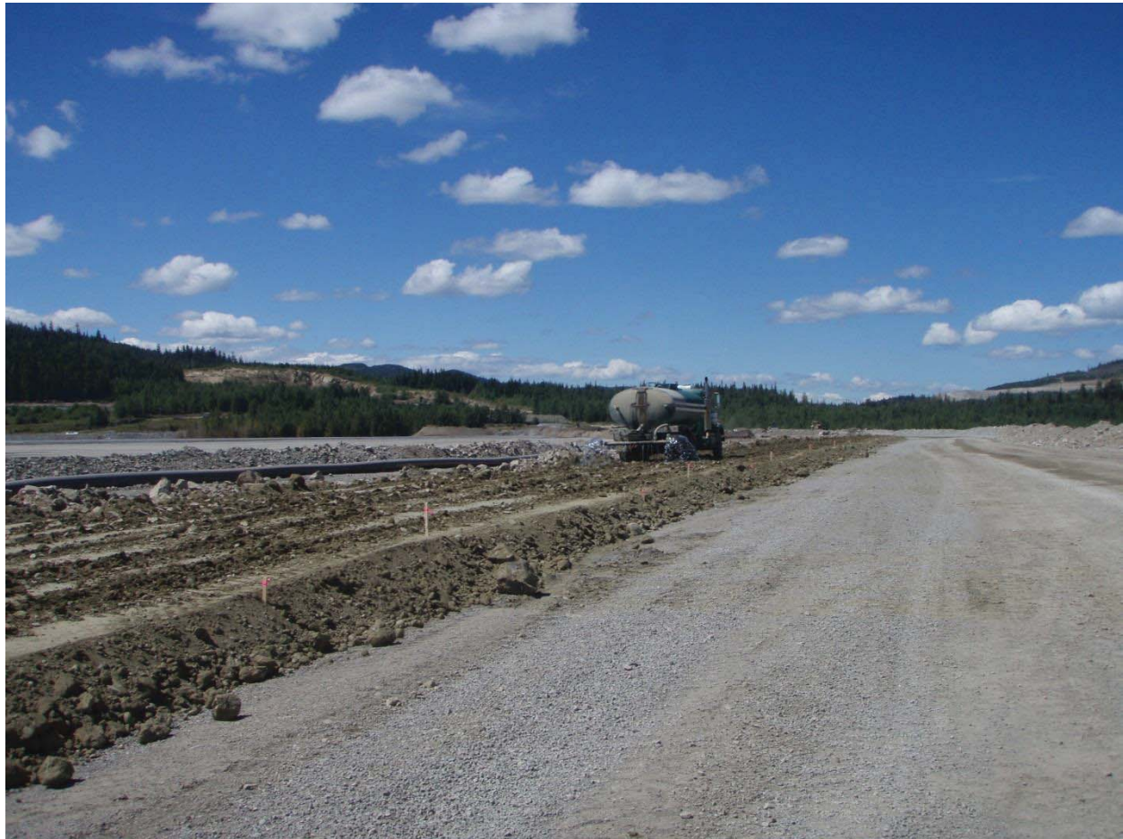
Water Truck soaking till
