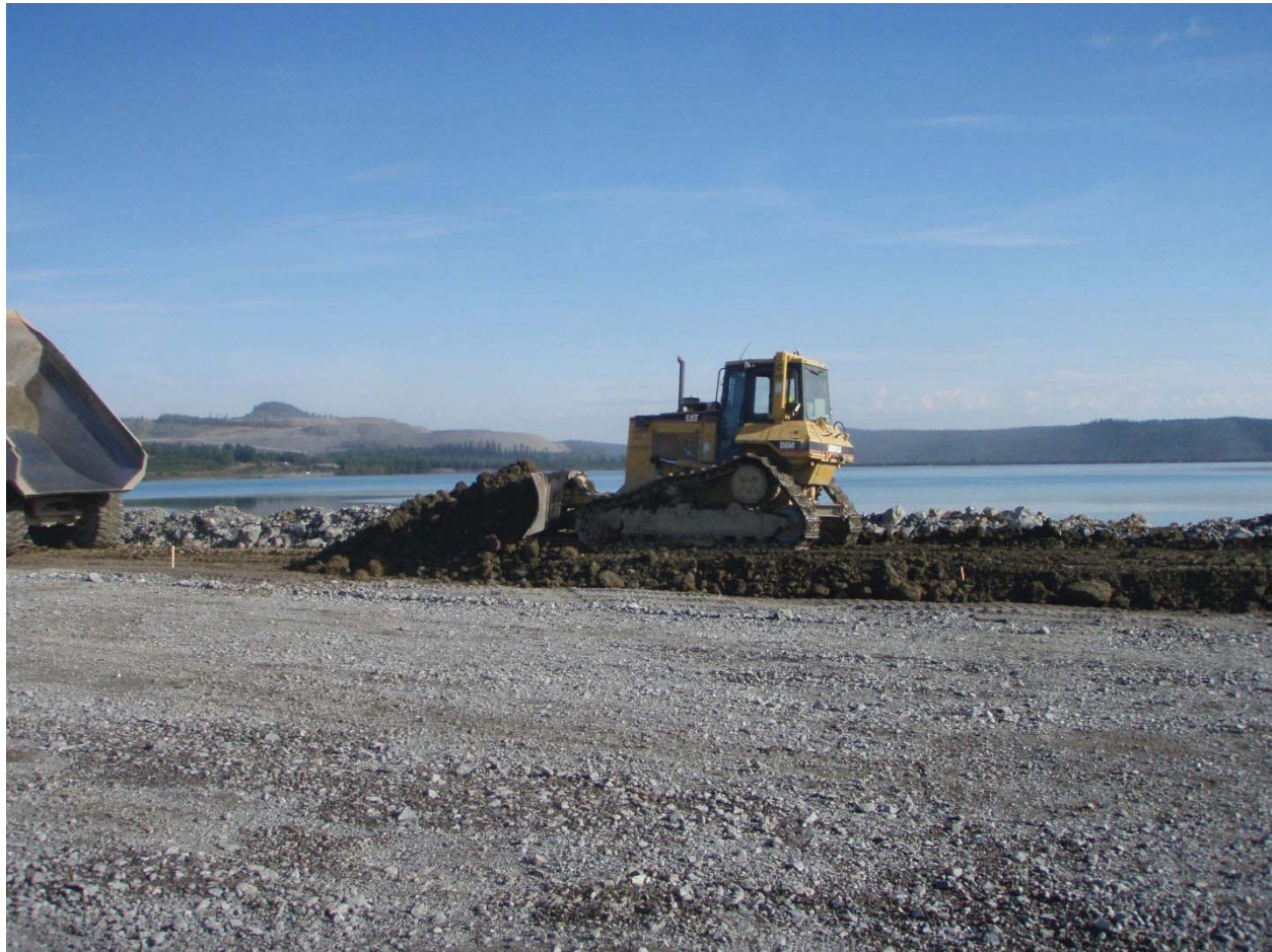
Dozer spreading till on SE (lift #7)
