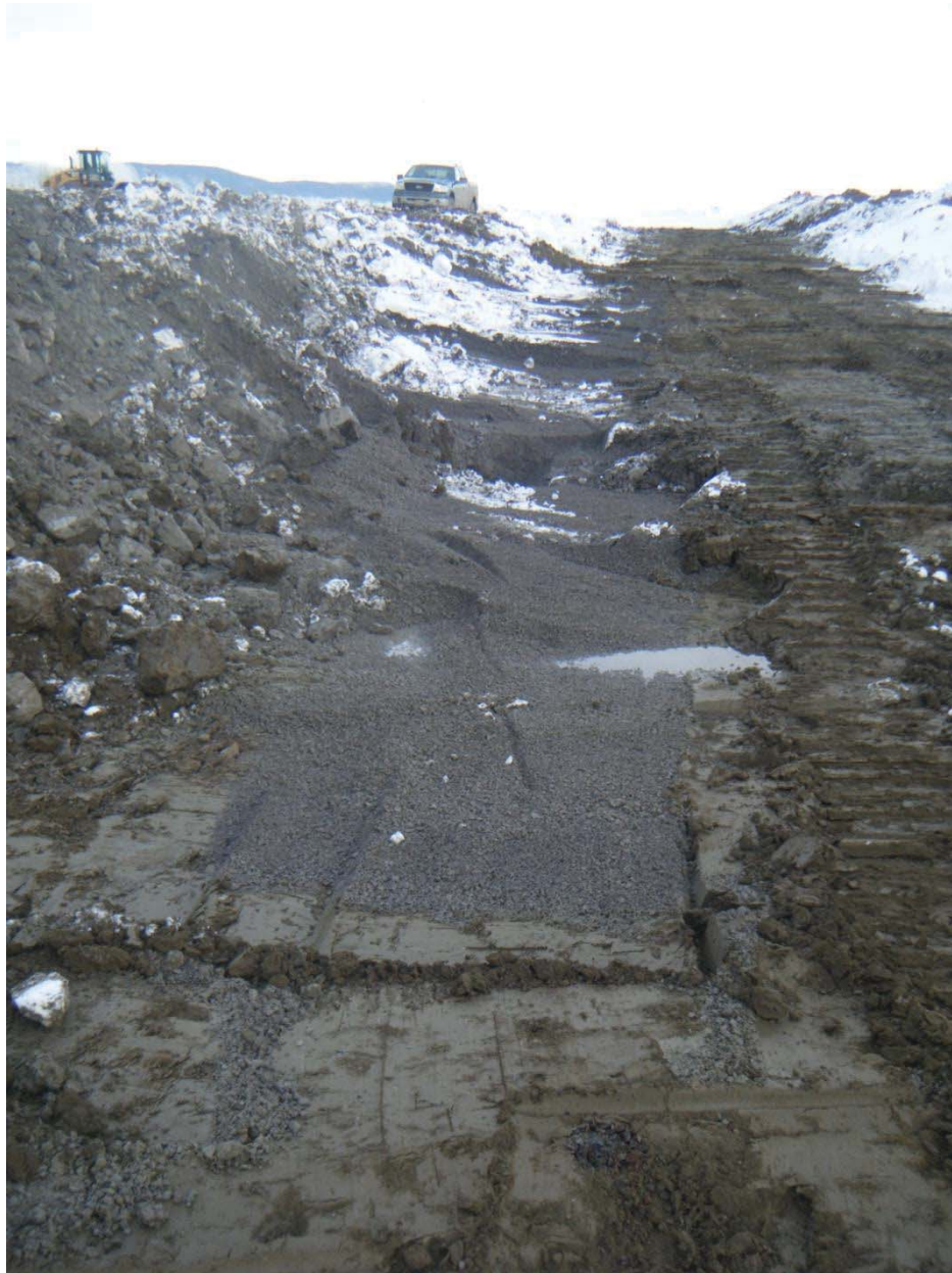
End of filter trench at corner 5 tie-in
