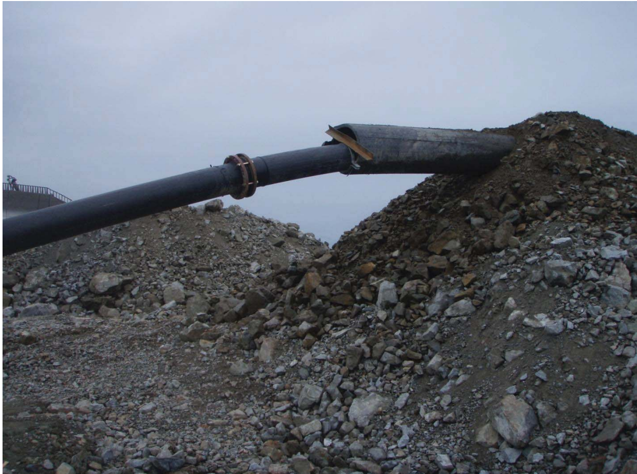
Ramp being built over ME tailings pipe using C zone material
