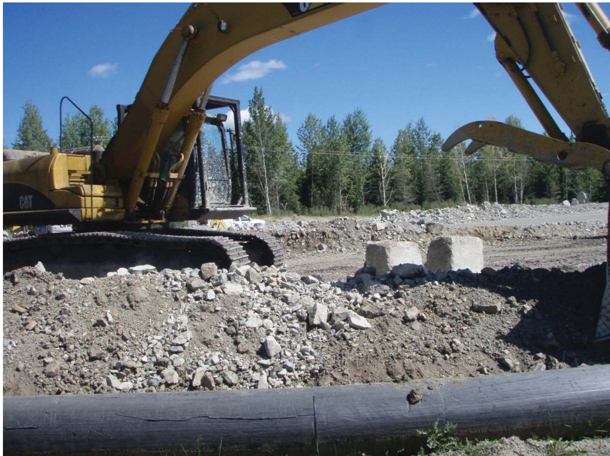
Tailings pipe at 5 corner raised to elevation 967.5
