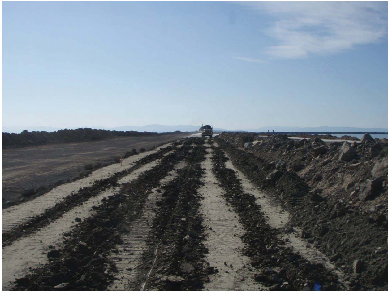
Water Trucking soaking ripped till
