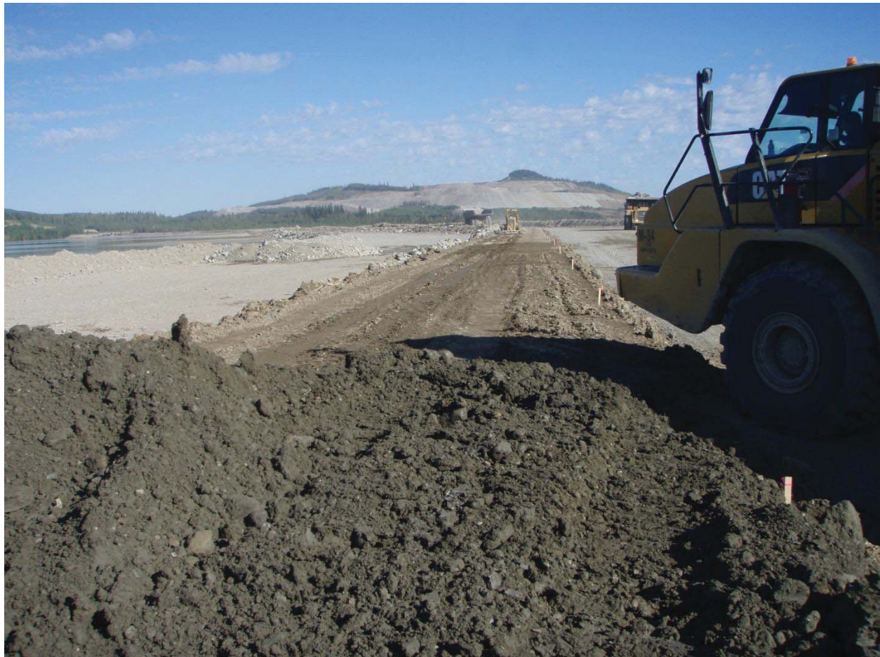
Ripped Till after water truck soaked with water
