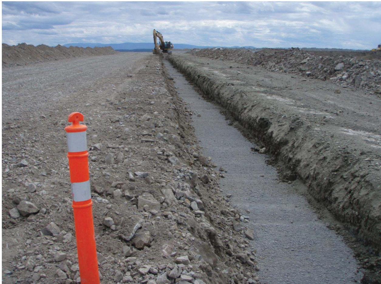
Filter trenching on PE from Station 3+500 to 2+850
