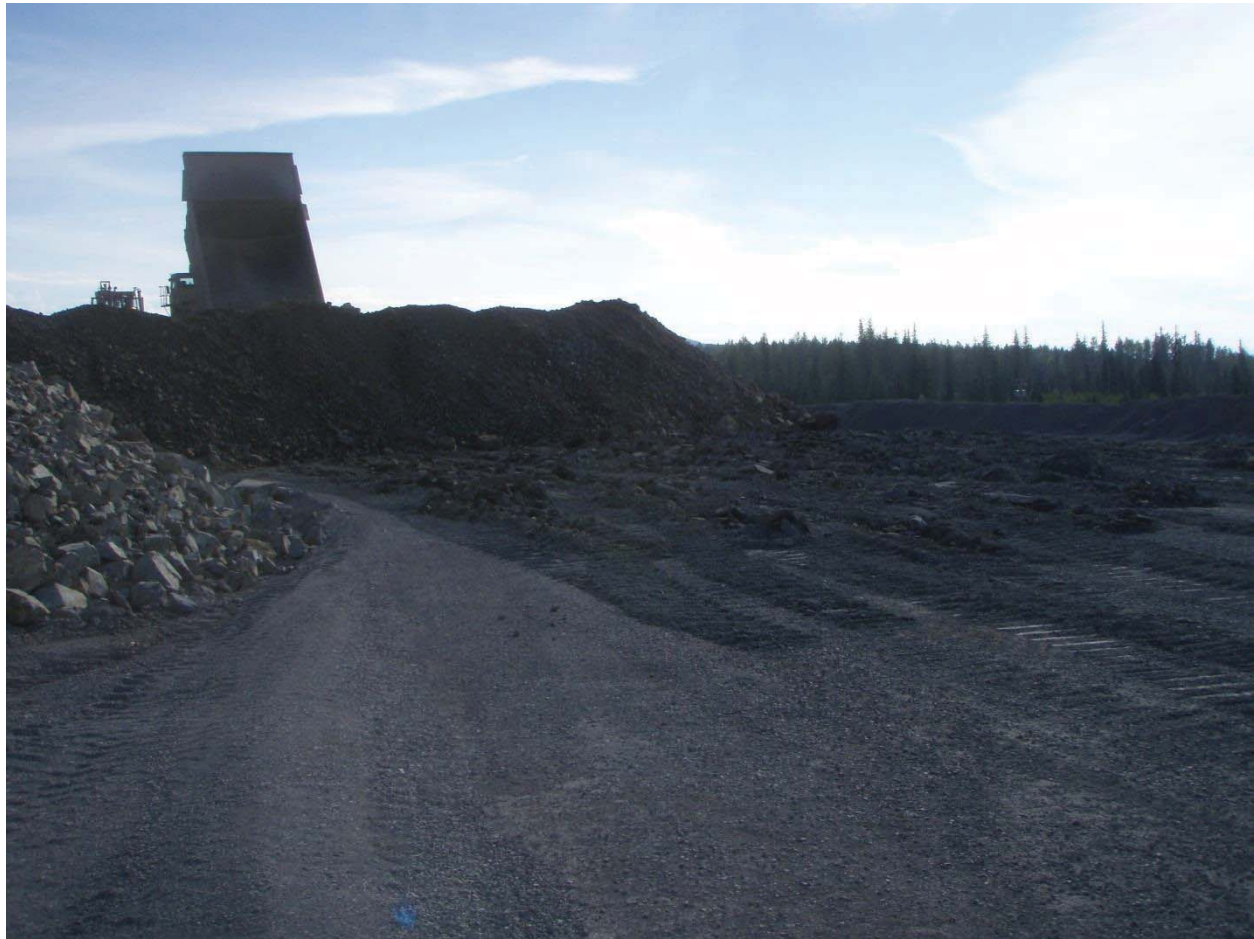
Haul Truck dumping rock for buttress below ME
