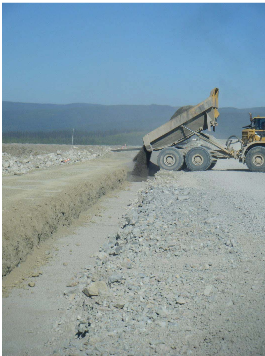
Filter material being placed on ME
