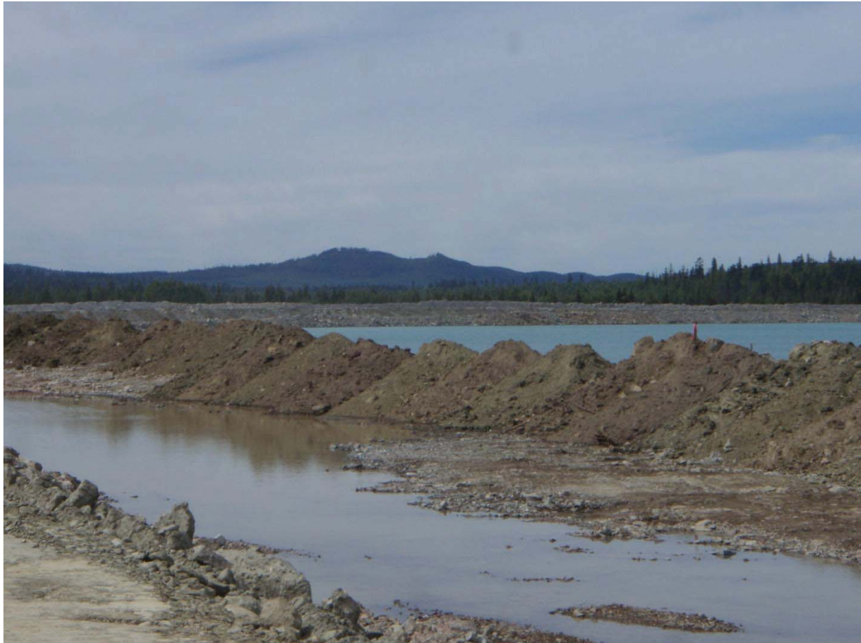
Waste material from the bottom of Corner 2 placed on top of ME US U Zone berm
