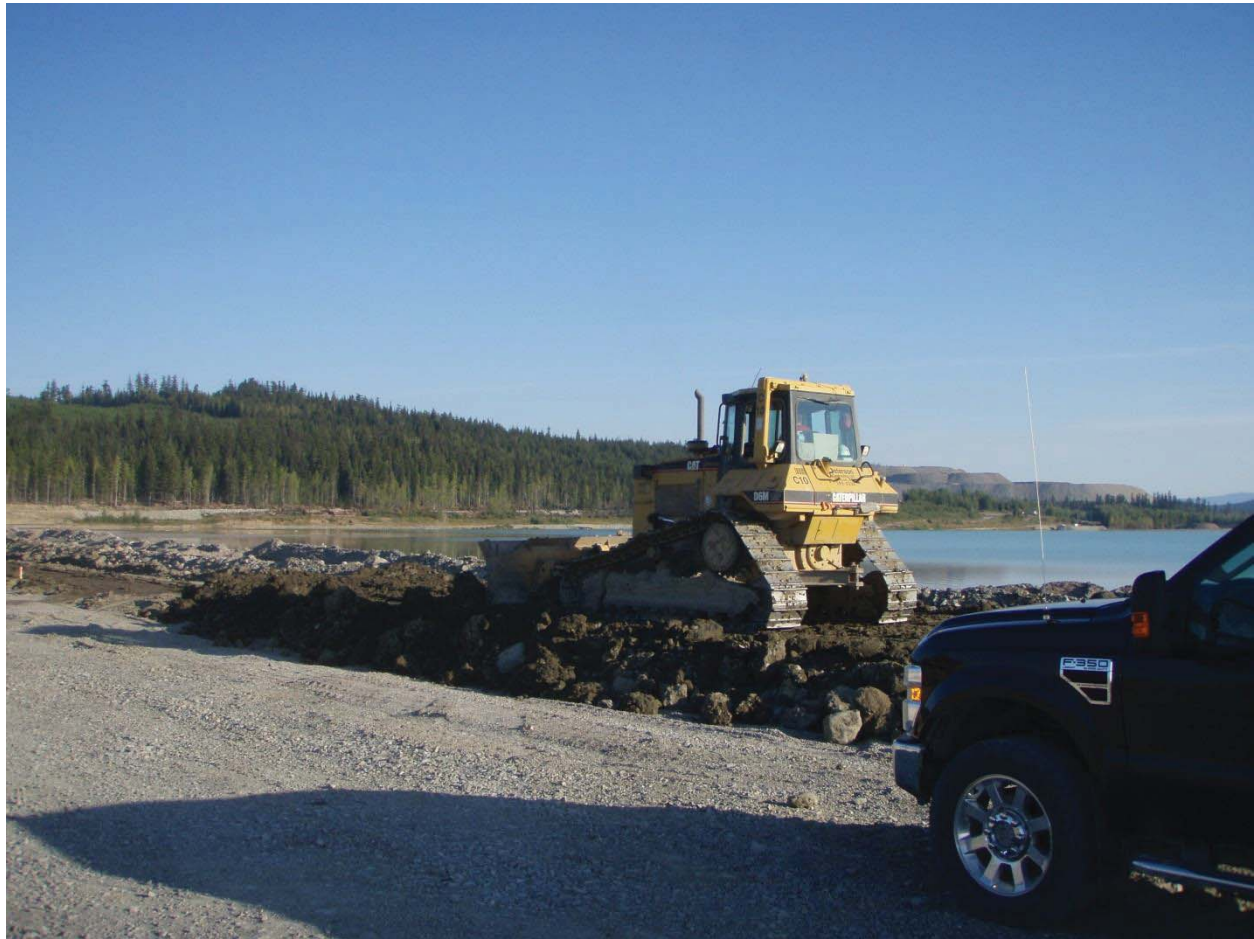
Dozer pushing till on SE (SE lift #8)
