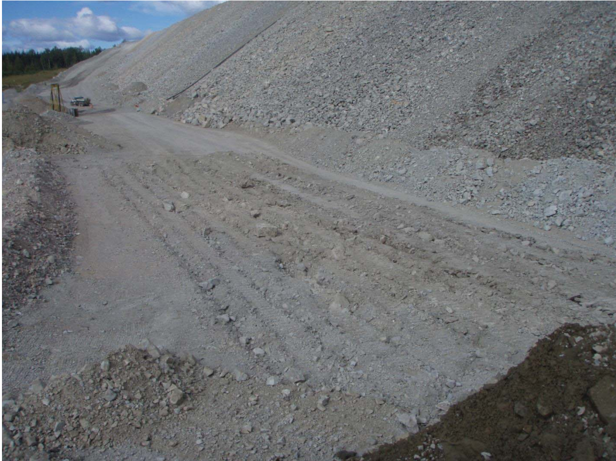
Scarification of C Zone in preparation for buttress lift
