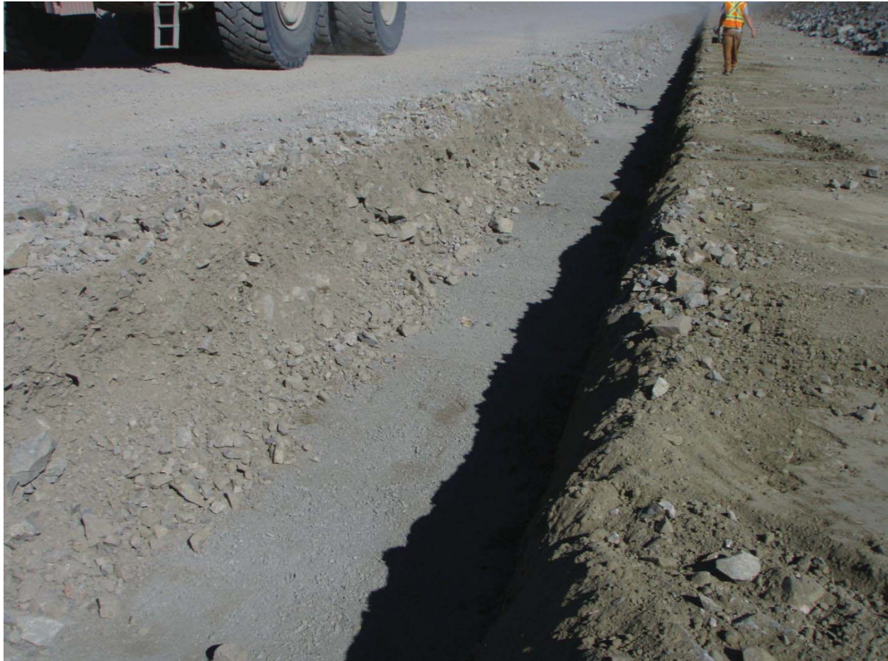
Filter trenching on PE from Corner 5 to Station 4+500
