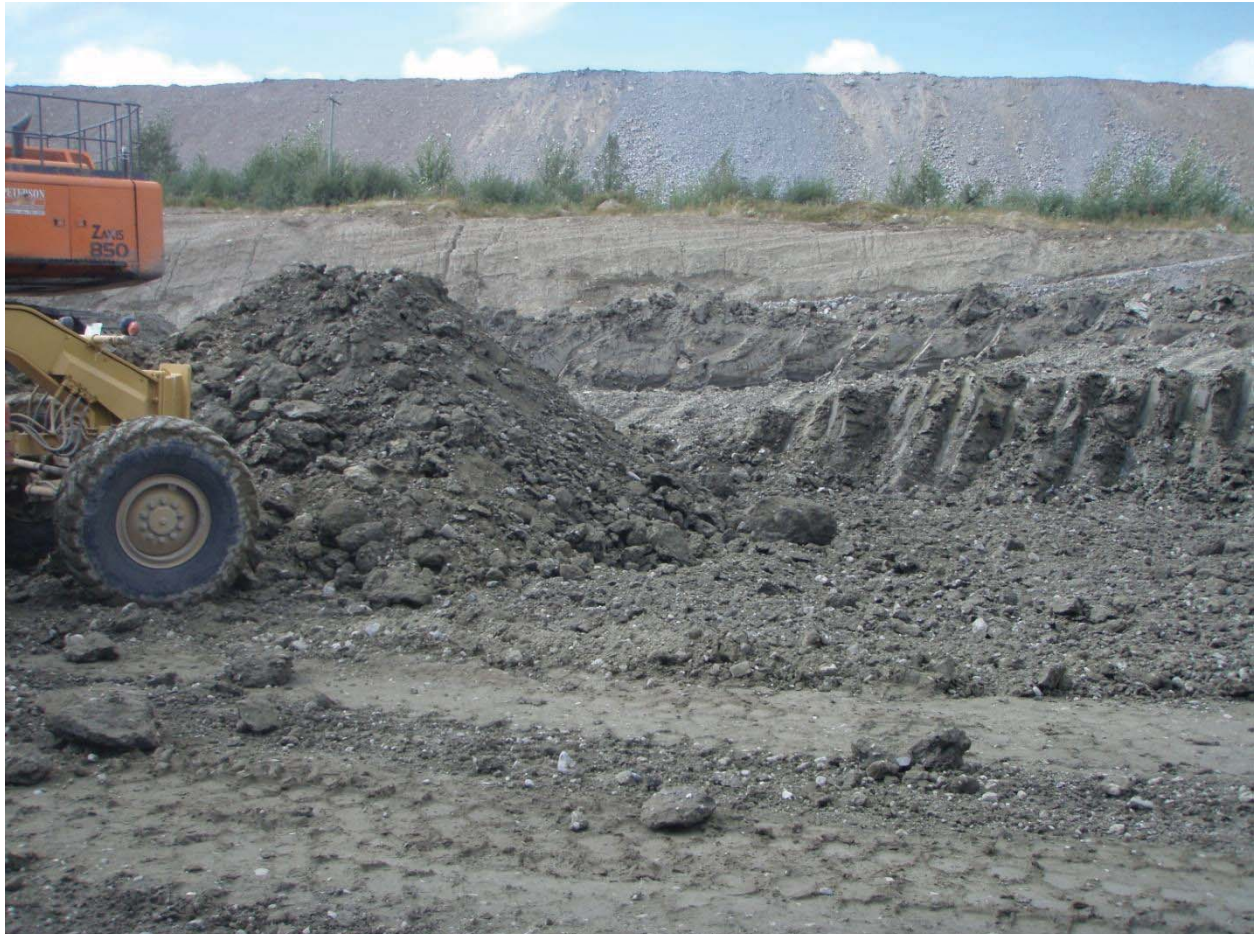
PE Borrow pit below corner 1 – Till being used for the lifts on ME
