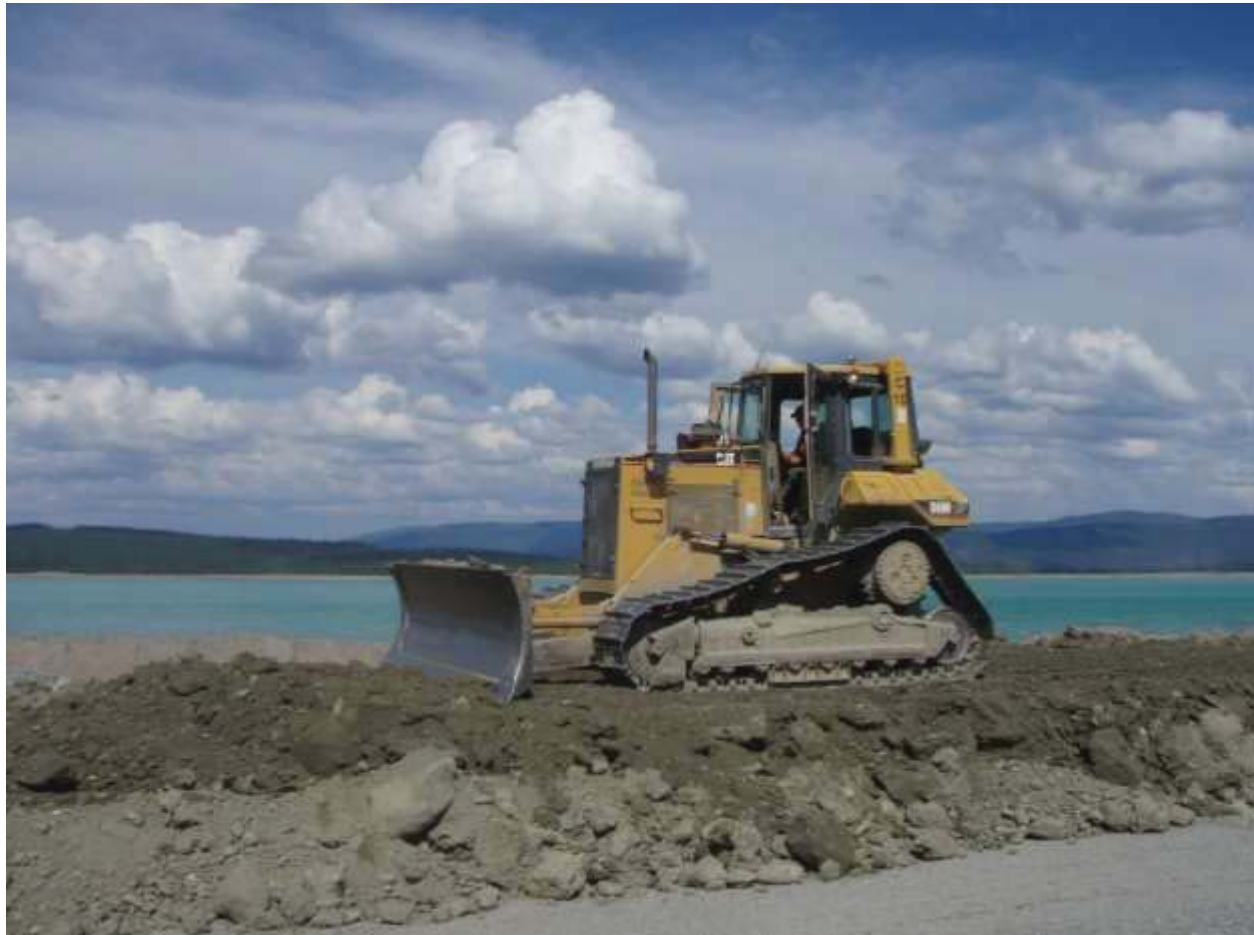
Dozer pushing Till on SE (SE lift #8)
