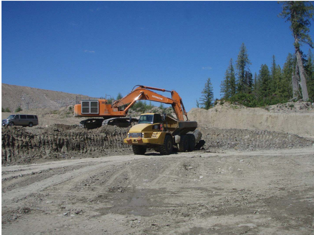
Wiggly being loaded with Till from Perimeter Borrow Pit
