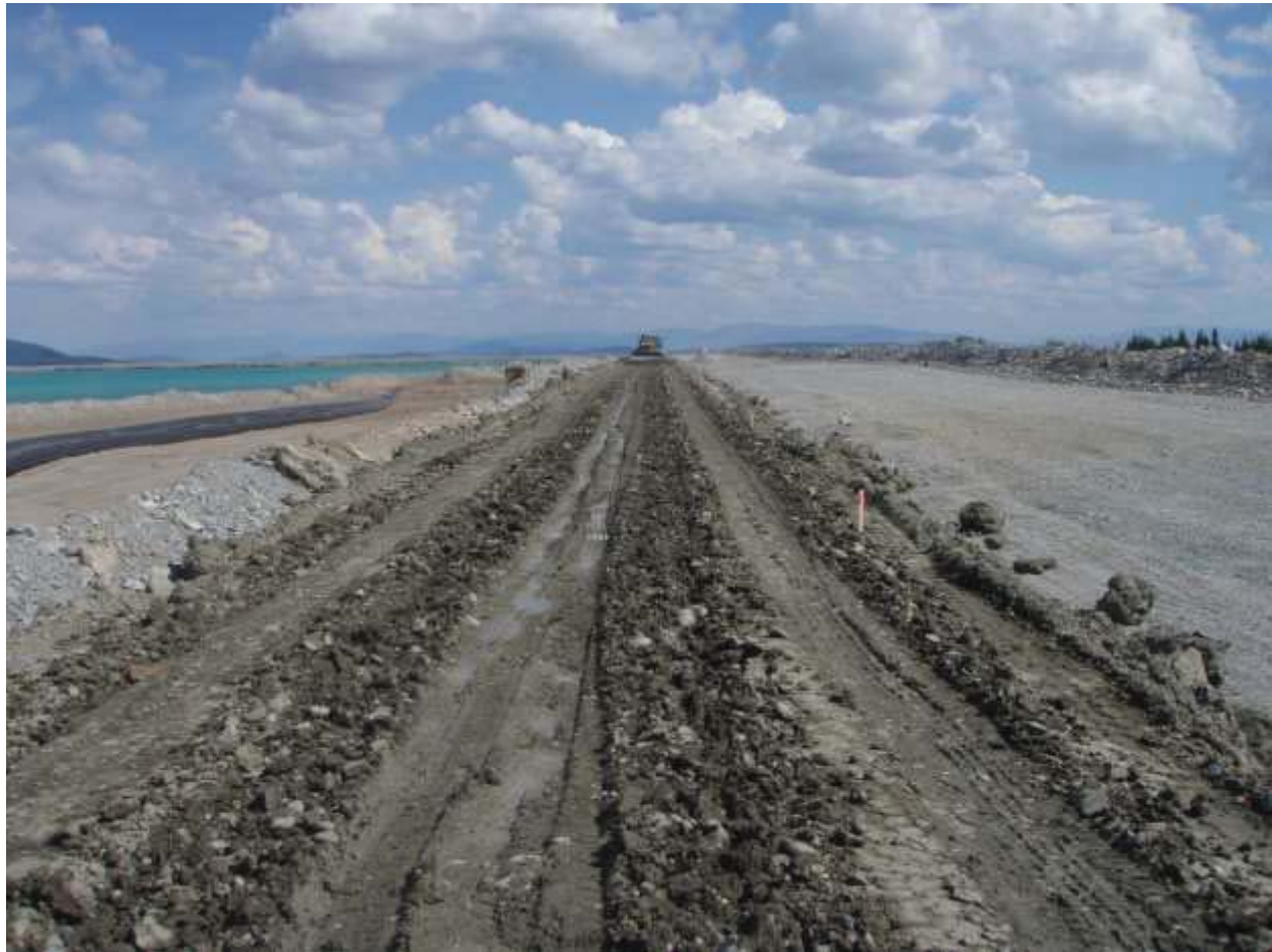
Ripped and Soaked Till on SE (SE lift #8)
