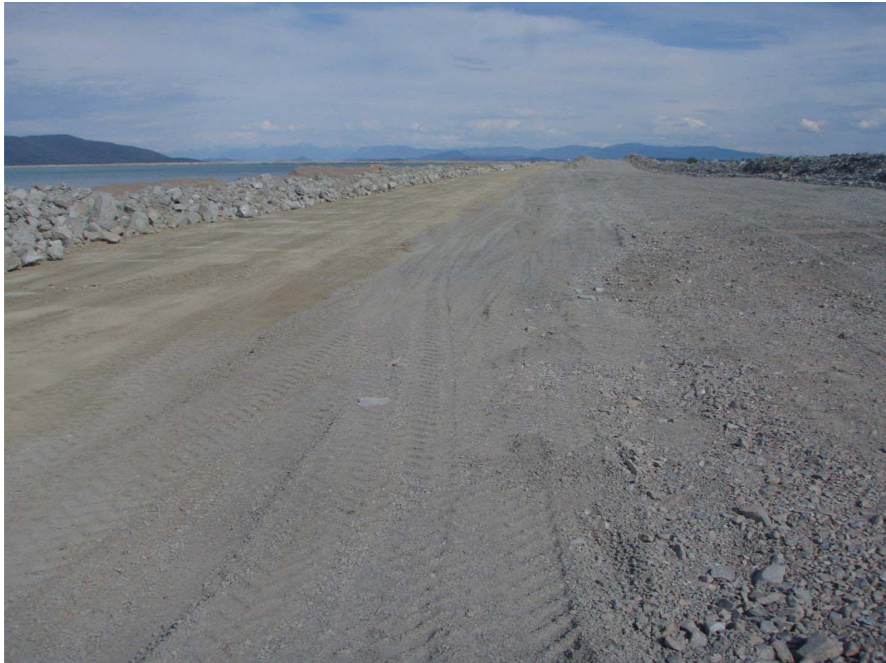
SE Zone F after filter material placement and spreading
