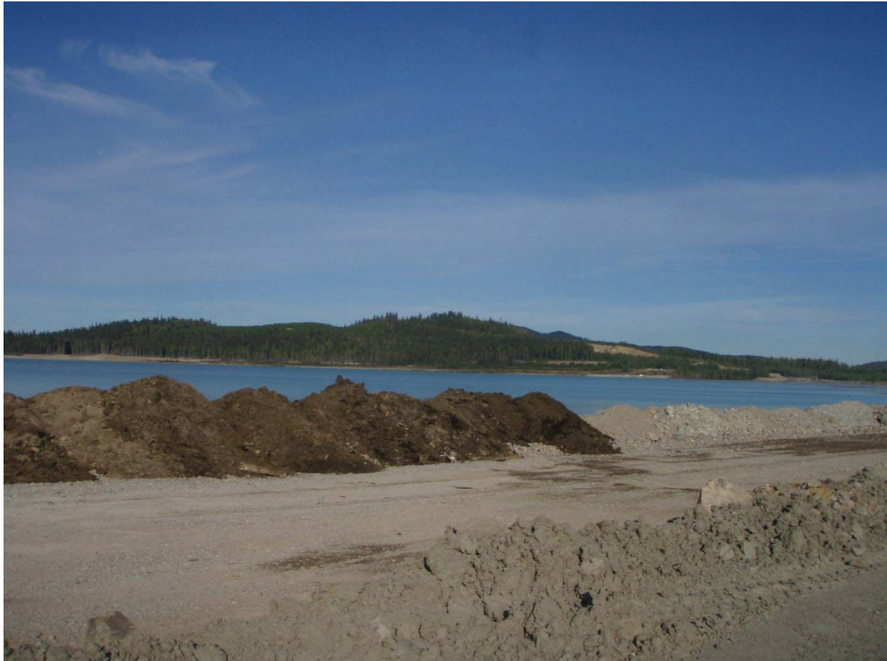
Waste material from the bottom of Corner 2 placed on top of PE US U Zone berm
