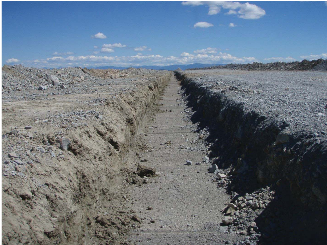
Filter trench on the SE
