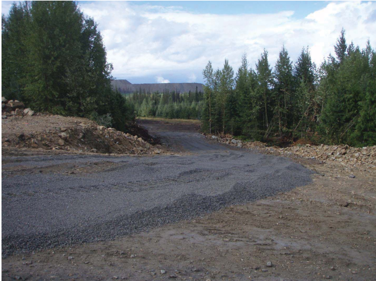
Filter material placed on new access road between 5 corner and Orica
