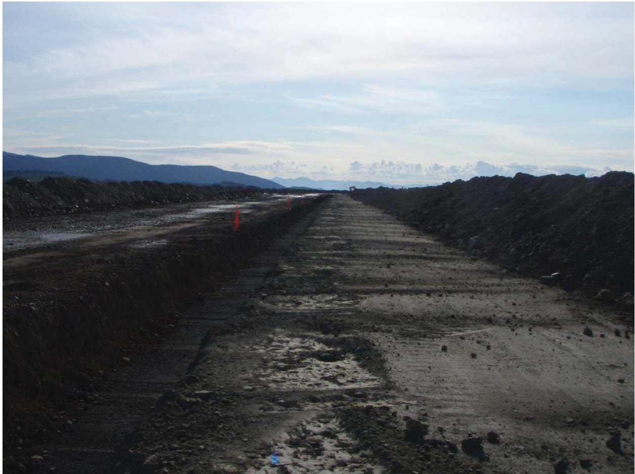
Filter trenching on PE from Station 4+500 to 3+500
