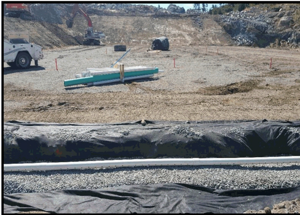
Photo 8 – Leak Detection and Leachate Collection Piping Systems
