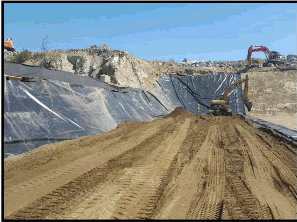
Photo 5 – Placement of Leachate Collection Sand Drainage Blanket
