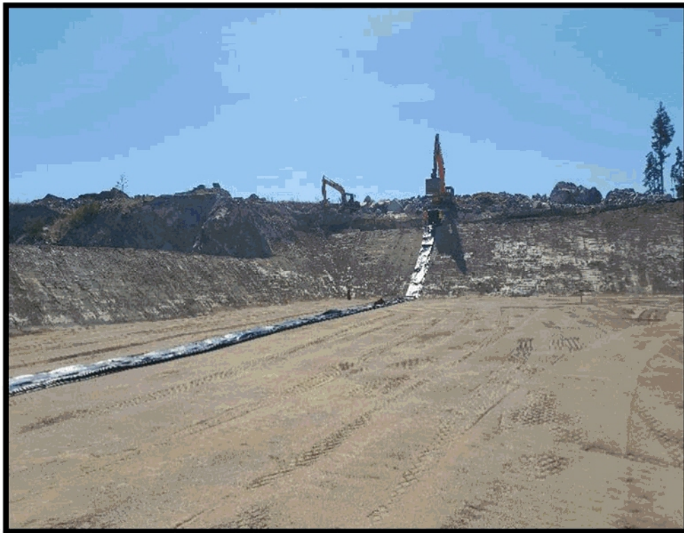
Photo 4 – Liner deployment
