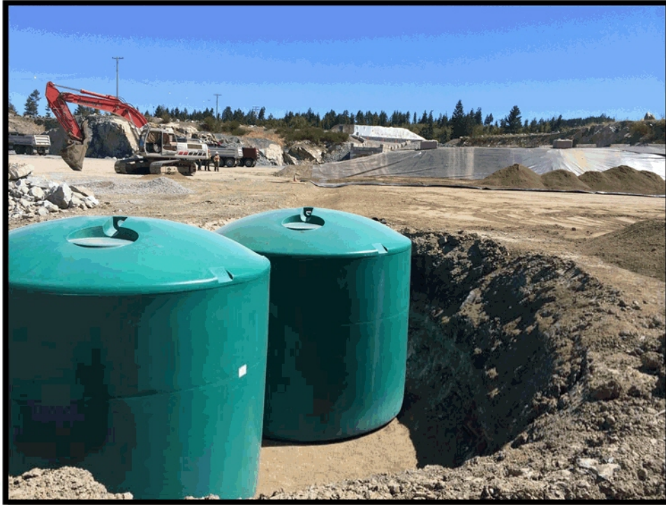
Photo 7 – Leak Detection and Leachate Collection Tanks
