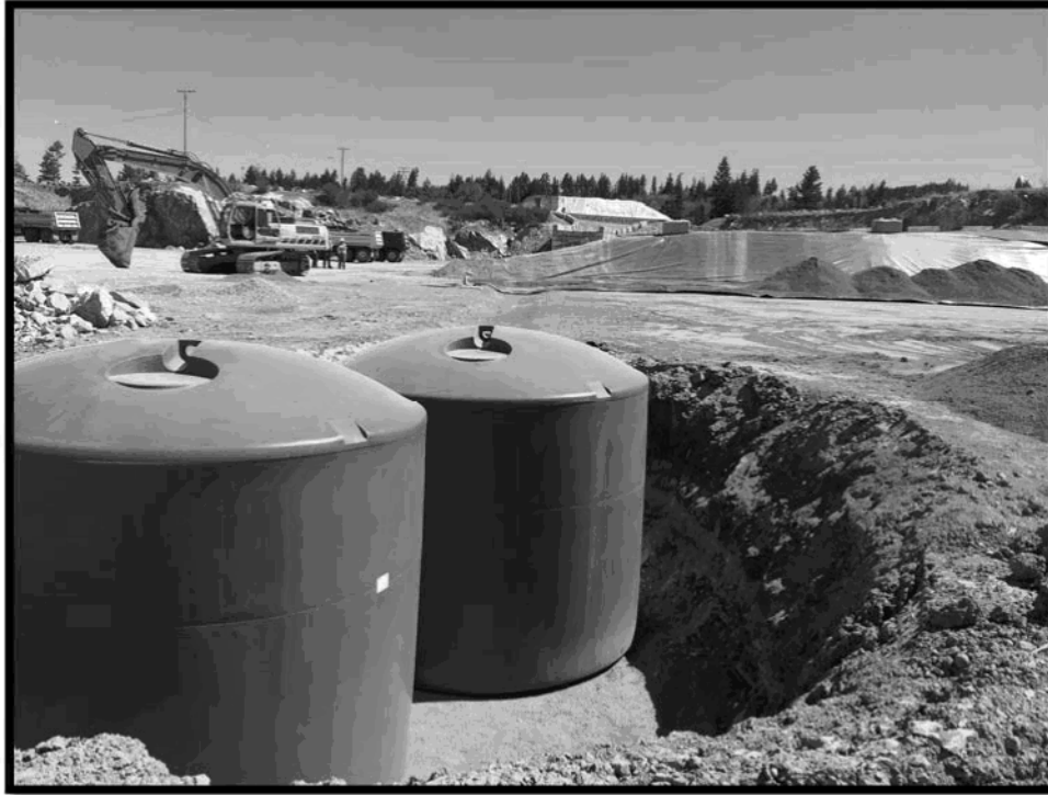
Photo 7 – Leak Detection and Leachate Collection Tanks
