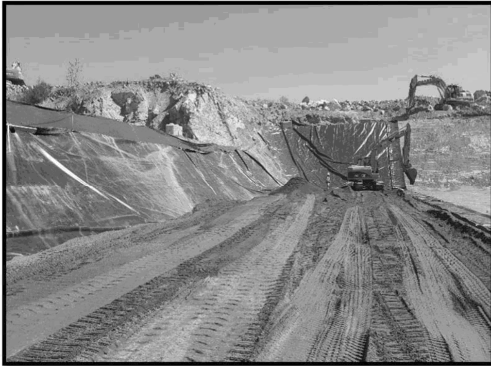
Photo 5 – Placement of Leachate Collection Sand Drainage Blanket
