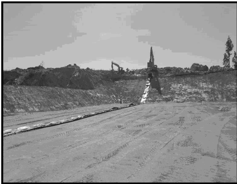
Photo 4 – Liner deployment
