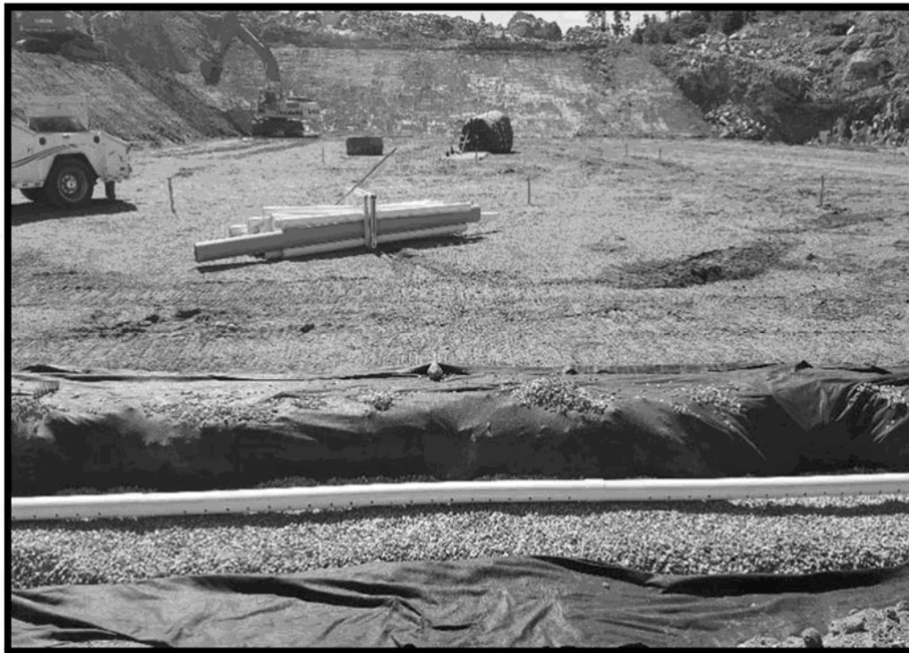
Photo 8 – Leak Detection and Leachate Collection Piping Systems
