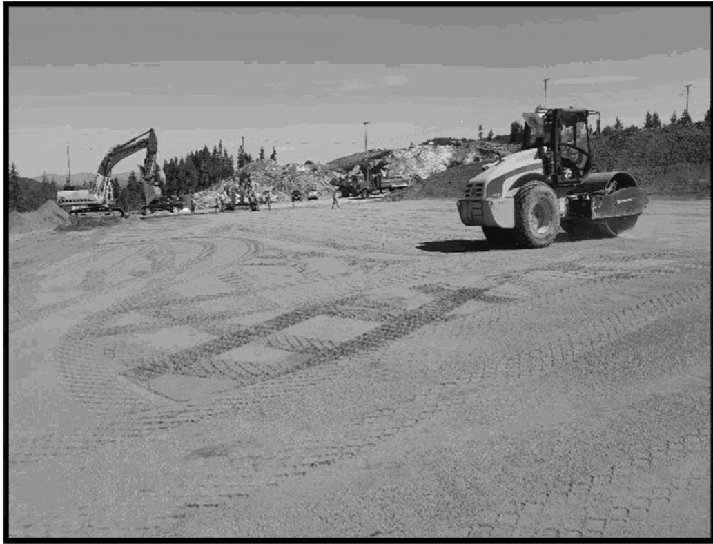
Photo 3 – Base sand surface being prepared for liner deployment
