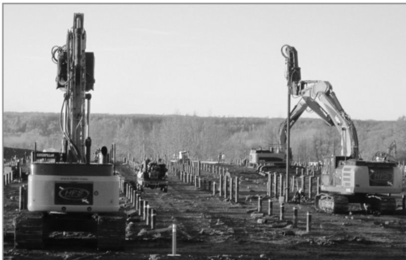
Excavators installing screw piles at the location of the worker accommodation camp.
