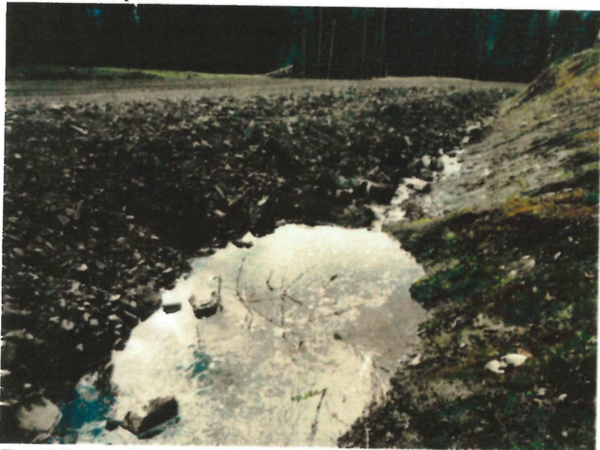
Figure 2. Drainage diversion occurring due to partially blocked culvert along the 3 – 35 km road section.
