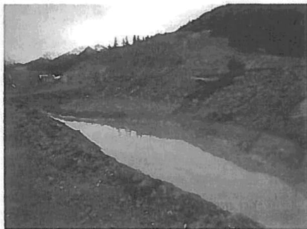
Photo 11 Exfiltration pond. Note high water level of sludge.
