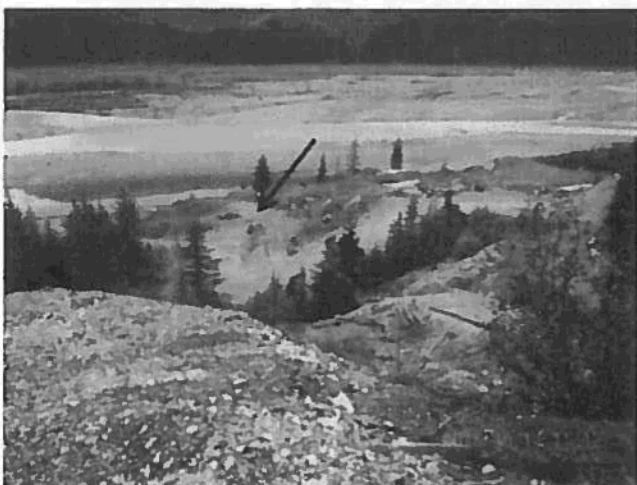
Photo 5: The black pipe (arrow) is the acidic discharge from the 5400 portal. Portal Creek and the combined non-acidic drainage discharge to the left of the picture in an underground HDPE pipe.
