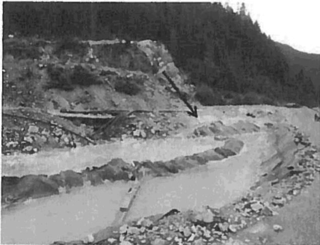
Photo 9: Exfiltration pond receiving ditch water from the 5200 portal
