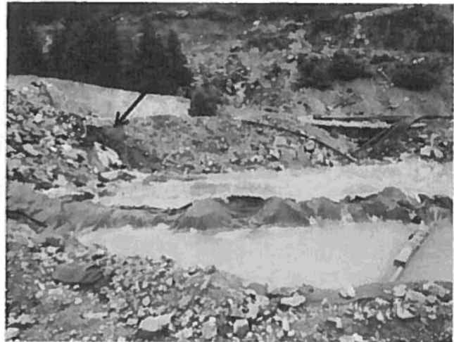
Photo 10: Exfiltration pond receiving acidic discharge from the 5400 portal
