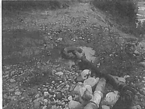
Photo 4: The neutral drainage is combined with the Portal Creek drainage into a HDPE pipe and diverted away from historical waste rock to the Tulsequah River
