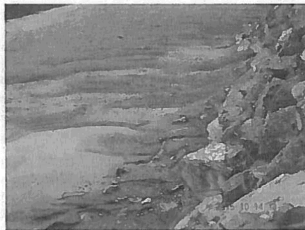
Photo 12: Diffuse discharge location through berm onto the Tulsequah river floodplain.
