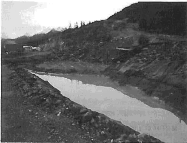
Photo 11 Exfiltration pond. Note high water level of sludge.
