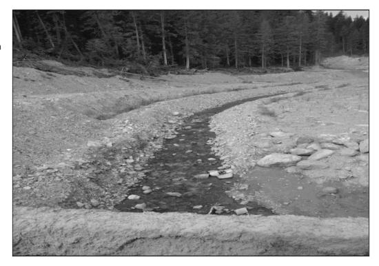
Discharge channel leading from the sediment control ponds at the end of Hazeltine Creek, leading to Quesnel Lake. Edney Creek was being diverted through the ponds and this channel at the time of the inspection, while the new creek channel was under construction.
