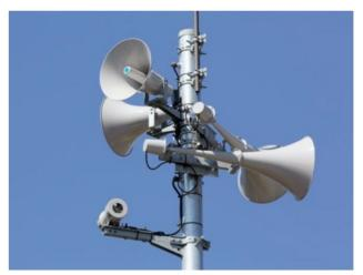
Figure 12 - An example of a Japanese loudspeaker array. Over 90% of Japanese cities, towns and villages have systems like this deployed.
