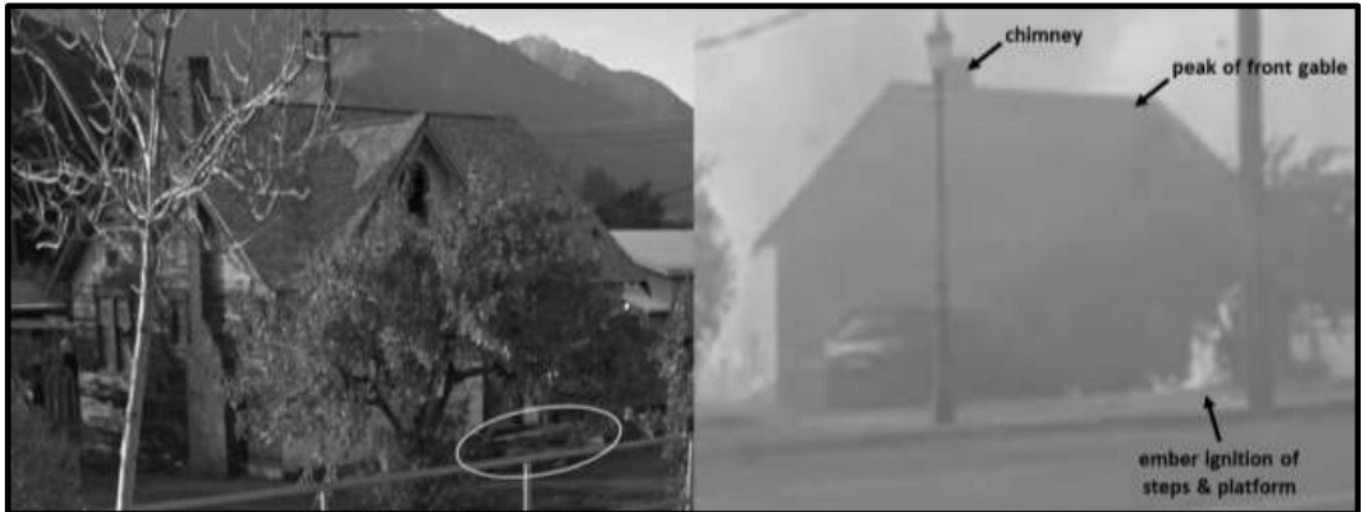
Figure 21: Burning embers ignited the ignition vulnerable wood steps and decking at the front entry way (right photo) of the house (right photo, yellow oval). Another ember ignited structure (right photo) is in the background to the left of the house in front. This house is also shown to the right of the Post Office in Figure 14.
