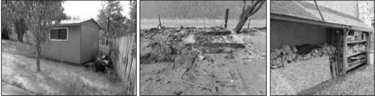
Figure 18: Outbuildings such as the shed on the left are ignition vulnerable from fire spreading in dead grass, flammable debris or a wood fence to contact and ignite it or directly ignite from burning embers such as the firewood on the right. Once ignited, the burning outbuilding or adjacent firewood ignites the house or business.
