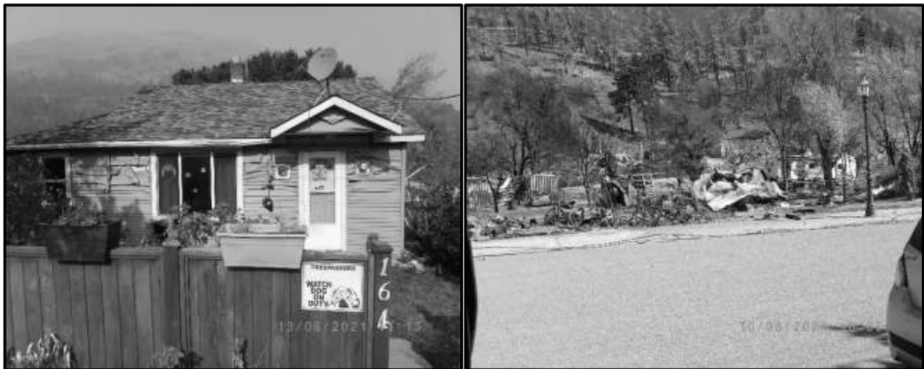
Figure 20a: Thermally softened vinyl siding on the upper third of the front facing burning structures across Fraser St. Note the wood fencing closer to the thermal source without char. (left)
