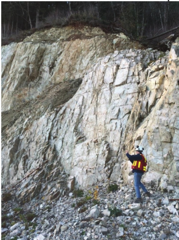
Photos 9 and 10: Overburden at crest of slope
