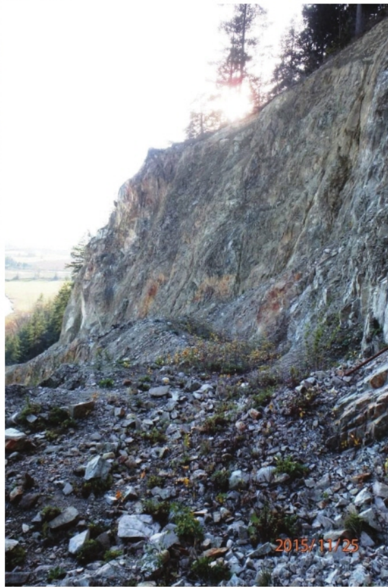
Photo 6: Upper access trail showing recent rockfall accumulation and area of failed fill slope
