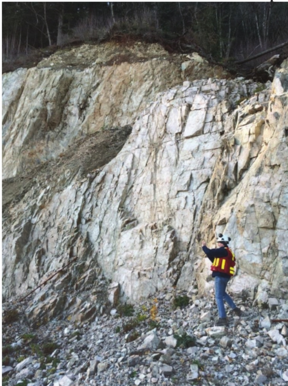
Photos 9 and 10: Overburden at crest of slope
