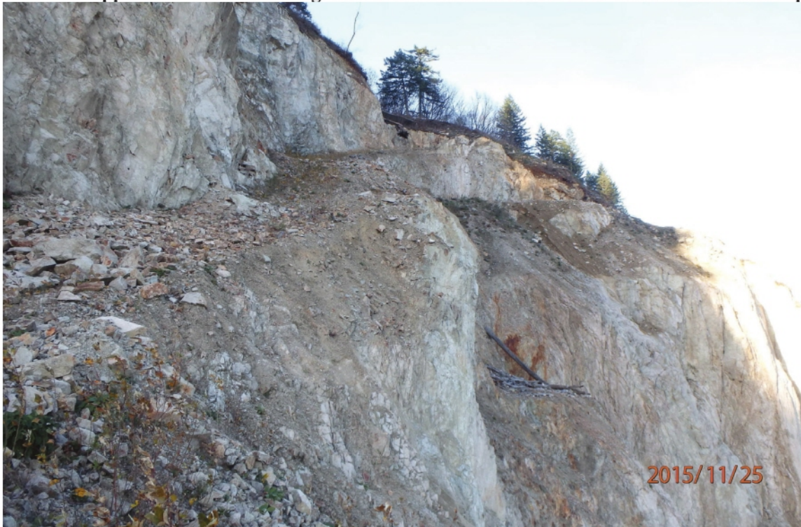
Photo 6: Upper access trail showing recent rockfall accumulation and area of failed fill slope
