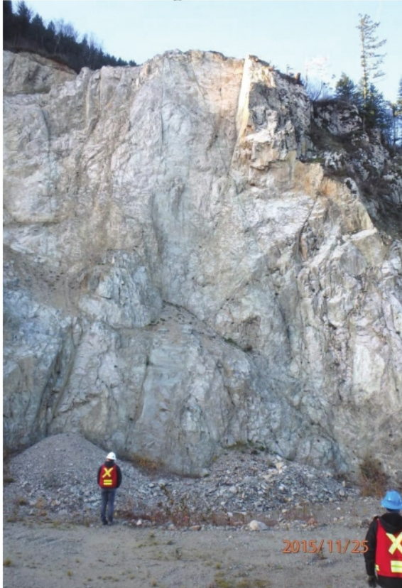
Photos 9 and 10: Overburden at crest of slope
