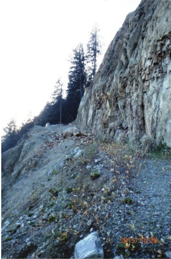
Photo 6: Upper access trail showing recent rockfall accumulation and area of failed fill slope
