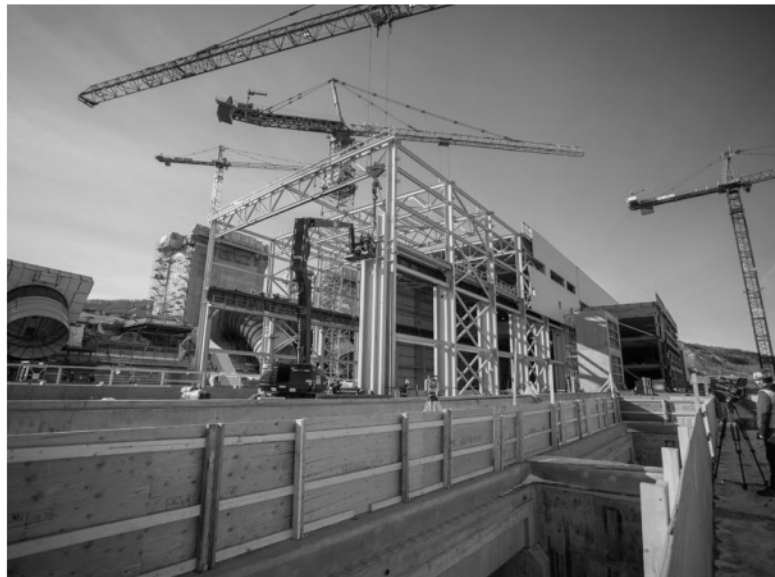
Figure A-5 Powerhouse steel superstructure construction. The powerhouse construction also includes concrete placements at the powerhouse, intakes and spillways, and the installation of penstock segments. (February 2021)
