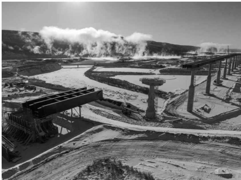
Figure A-2 Halfway River bridge construction where the final girders will connect pier 12 to the eastern bridge abutment (January 2021)
