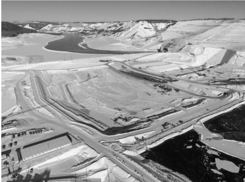
Figure A-7 The upstream and downstream cofferdams, which divert the Peace River through the two diversion tunnels (February 2021)
