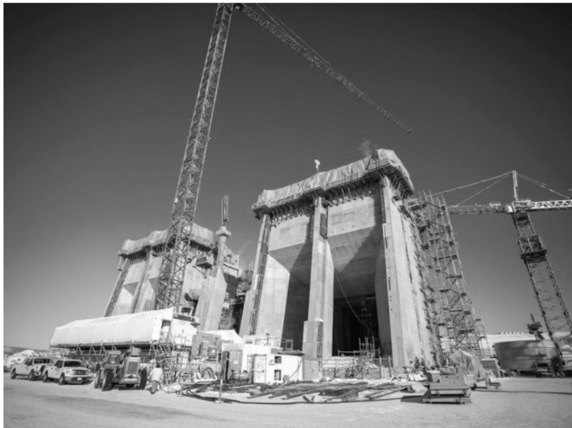
Figure A-8 Intake Units 1 and 3 are nearing completion as part of the ongoing powerhouse construction (February 2021)
