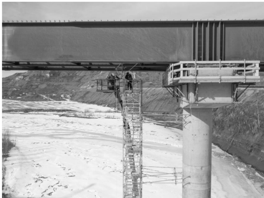
Figure A-10 Girder installation is complete, and workers remove scaffolding from the Halfway River bridge (March 2021)
