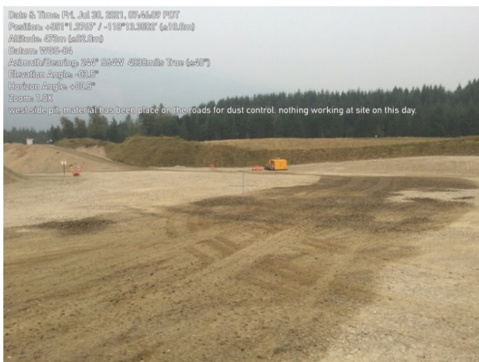
Image #2 - showing dust suppression material on the roads.
