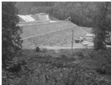
Coquitlam Dam – Zone 1 Impervious Core at El. 150 m, Oct 2007
