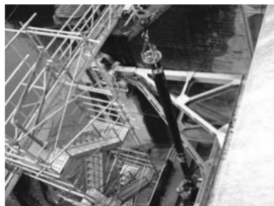
Ruskin Dam – Bay 7 Anchor Installation
