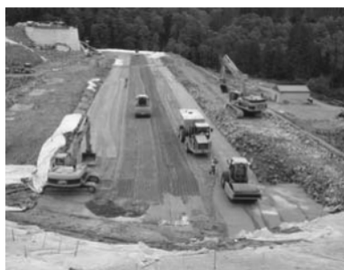
Coquitlam Dam – Zone 1 fill placement excavation, Oct 2007
