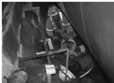
La Joie Dam – North conduit, setting up for drilling for conduit supports
