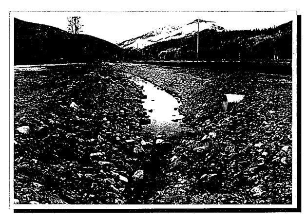
PHOTO 7: Tributary #3 approximately 200 m from the confluence with Michel Creek. Crosses main road approximately 1km upstream of rail loop bridge. Note hanging culvert blocking access to suitable upstream juvenile habitat.
