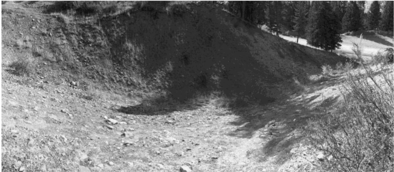
Photograph 4: View to the south to the Bull River Road, showing the lower end and deposition zone from the old washout gully. The gully was stabilized in 2015 and TSF surfaces were modified to ensure surface water, if any, would flow north away from the crest of this gully.
