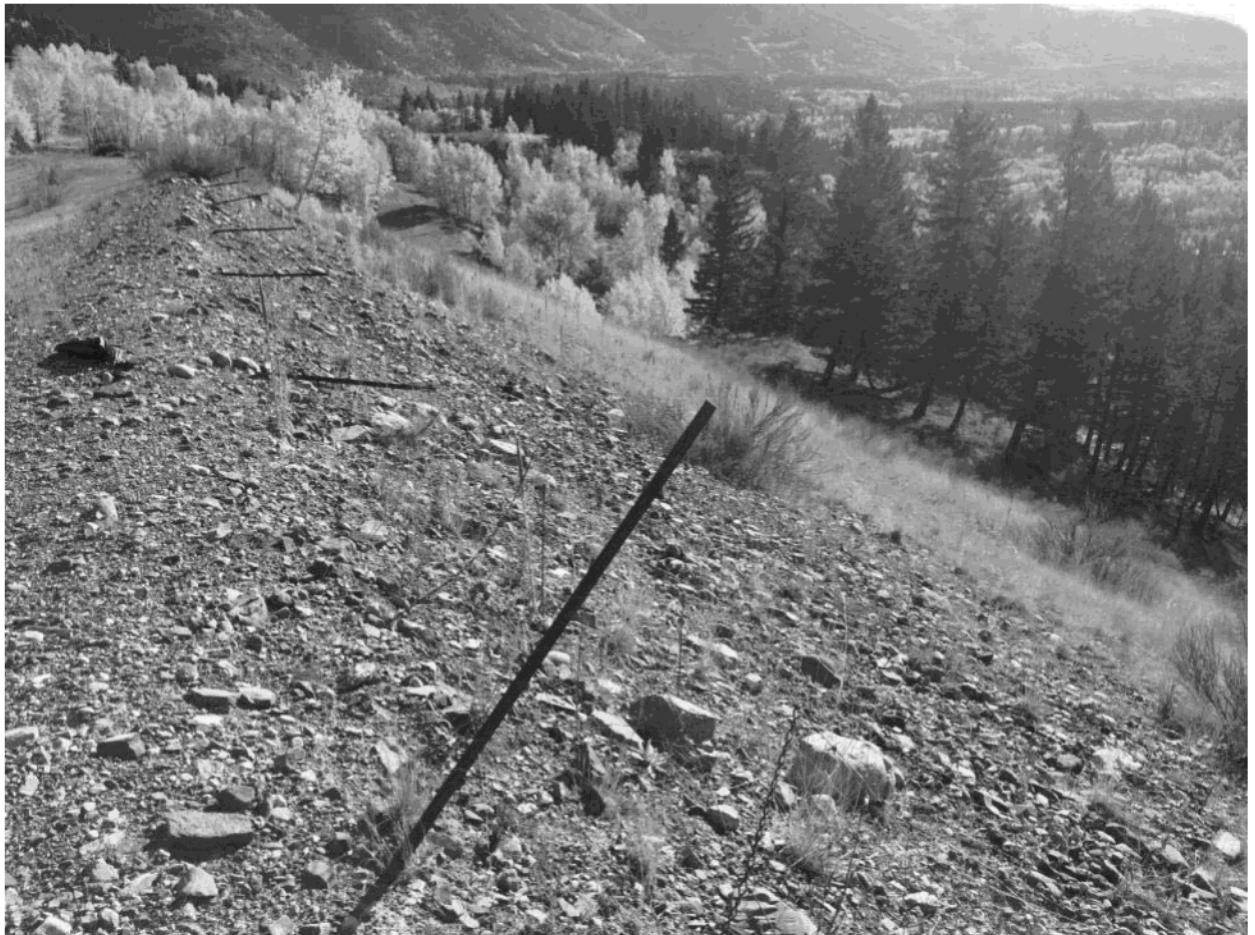
Photograph 9: View to the east along the south TSF crest, with the Bull River Road in the lower right background. The embankment's downstream face appeared to be free from signs of instability and erosion along its perimeter.
