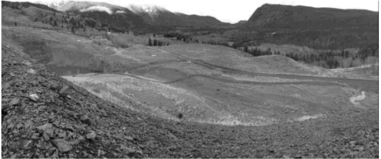
Photograph 1: View to east from the waste dump in fall 2016. The primary settling pond / open pit is visible at the left edge. A haul road transects the TSF near the center of the photograph. The south (right) edge of the TSF crest has a depression hosting the old washout gully. The TSF surface slopes north (left) to the settling pond, with ditches and a culvert under the haul road.
