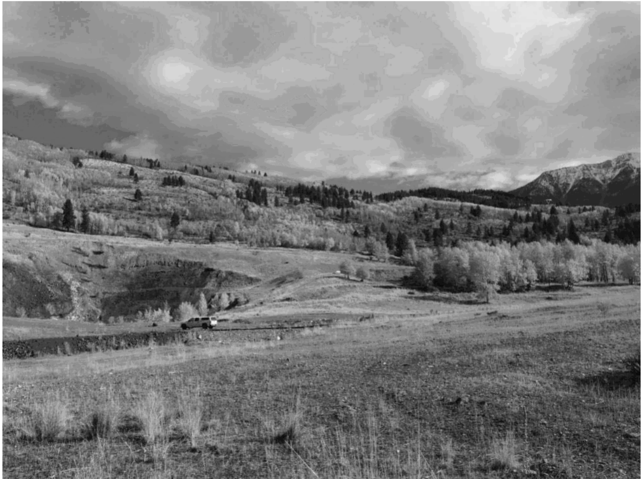
Photograph 6: View to northeast to terrain on the north fringe of the TSF, with the old open pit at the left edge of the photograph. The soils are relatively porous, and terrain graded toward the pit or to ditches flowing to the open pit situated just beyond the white pickup truck.
