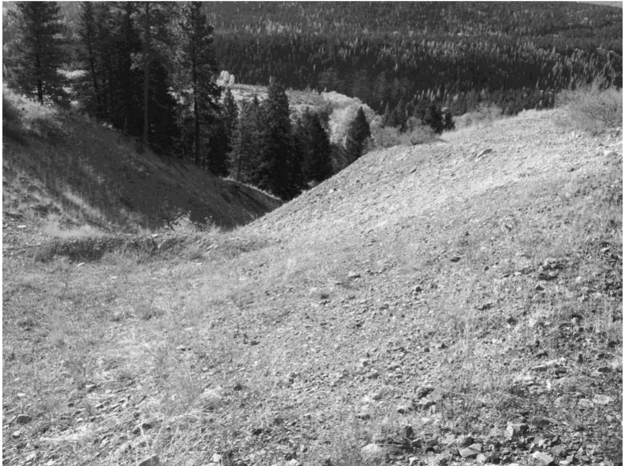
Photograph 3: View south down the old washout gully to the Bull River Road from the TSF crest. Dam soils consist of silty sands with gravels and cobbles. The side slopes were repaired and recontoured in 2015. Cross berms were installed. The TSF surface, behind the photographer, was shaped and ditched to shed water in the opposite direction from this gully, north toward the settling pond. No changes were observed compared to 2016.
