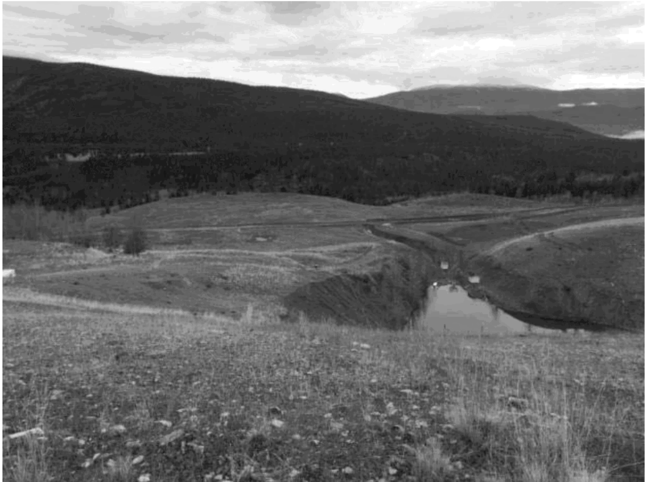
Photograph 2: View to the south from a road above the open pit / settling pond in fall 2016. The TSF is in the center background, and the Bull River canyon is located in the background beyond the TSF. Ditches draining to the settling pond are visible, and the pond is pumped daily to the southwest in pipes to old Burntbridge Creek. The old washout gully is visible just above (south) the settling pond in the photograph, beyond the haul road.
