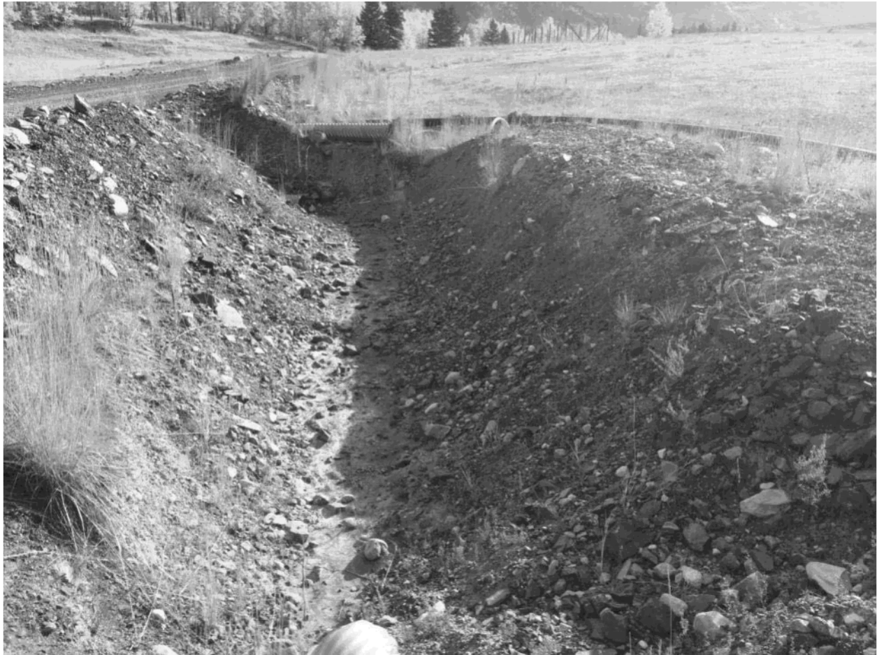
Photograph 5: View to east at the haul road through the TSF. The foreground ditch and culverts were constructed in 2015 to ensure any surface water would flow north to the primary settling pond in the old open pit, situated left of this photograph.
