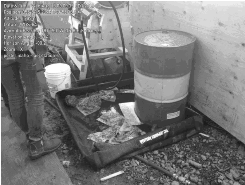
Photo is of the secondary containment at the fueling station.
